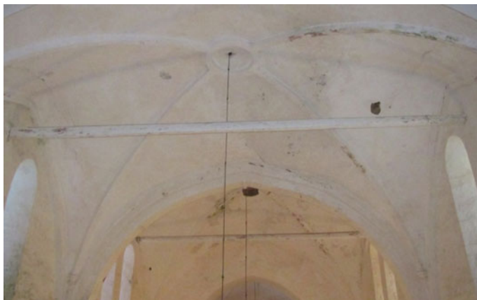
Fig. 22 To avoid additional deformations, the ribbed vault has been strengthened with tensile chords
