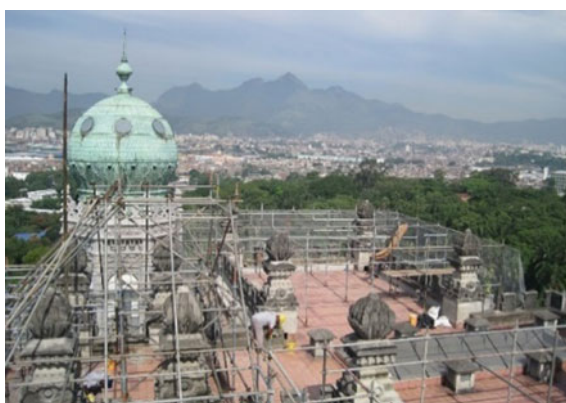
Fig. 24 Scaffolds on the seventh-floor terrace (May 2014)
