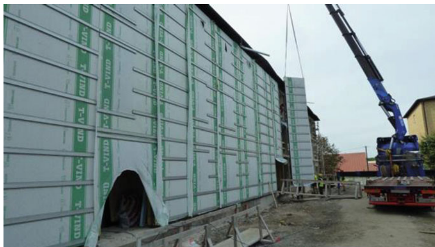
Fig. 8 Mounting of the elements at one of the buildings at Brogården. Photograph Elementum Eco AB
