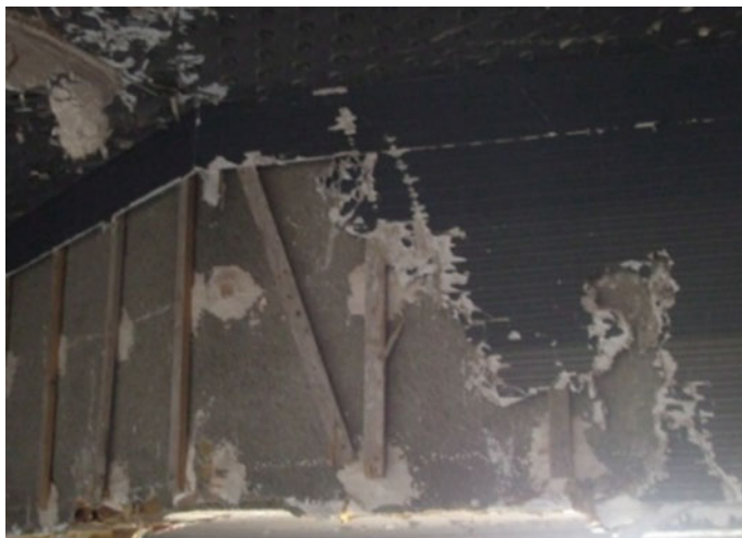
Fig. 9 Acoustic grooved panels in blue plaster
