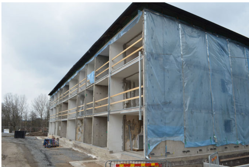
Fig. 6 The concrete frame after the old façade was dismantled
