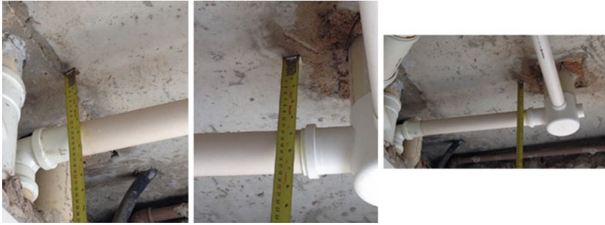
Fig. 9 Opposite slope of the siphoned drain
