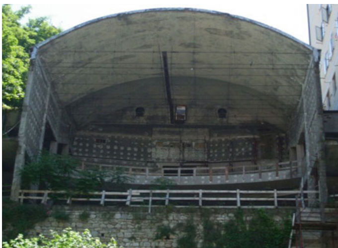
Fig. 4 The north-west facade
