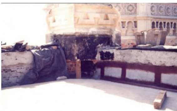
Fig. 12 North wing terrace on the seventh floor (1990)
