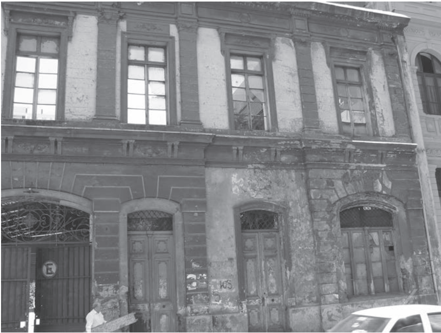
Figure 7.15 A preserved façade in Santiago, Chile, behind which is a storage yard. The façade had to be retained because it is in a conservation area. Image courtesy Peter Collier, Department of Geography, University of Portsmouth, UK.
