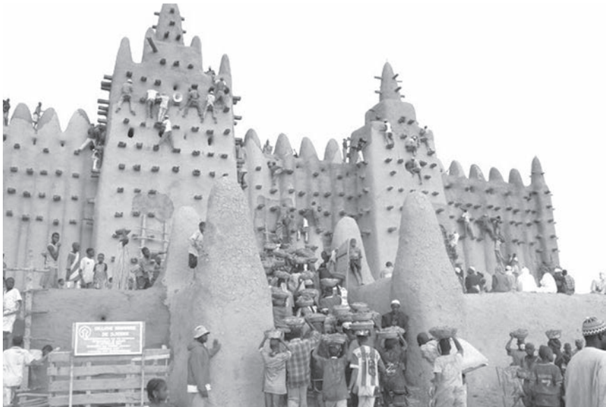
Figure 2.1 The community in Djenné participates every year in the replastering of the Great Mosque under the guidance of the guild. Image courtesy Peter Howard, www.AfricanWorldHeritageSites/Peter .
