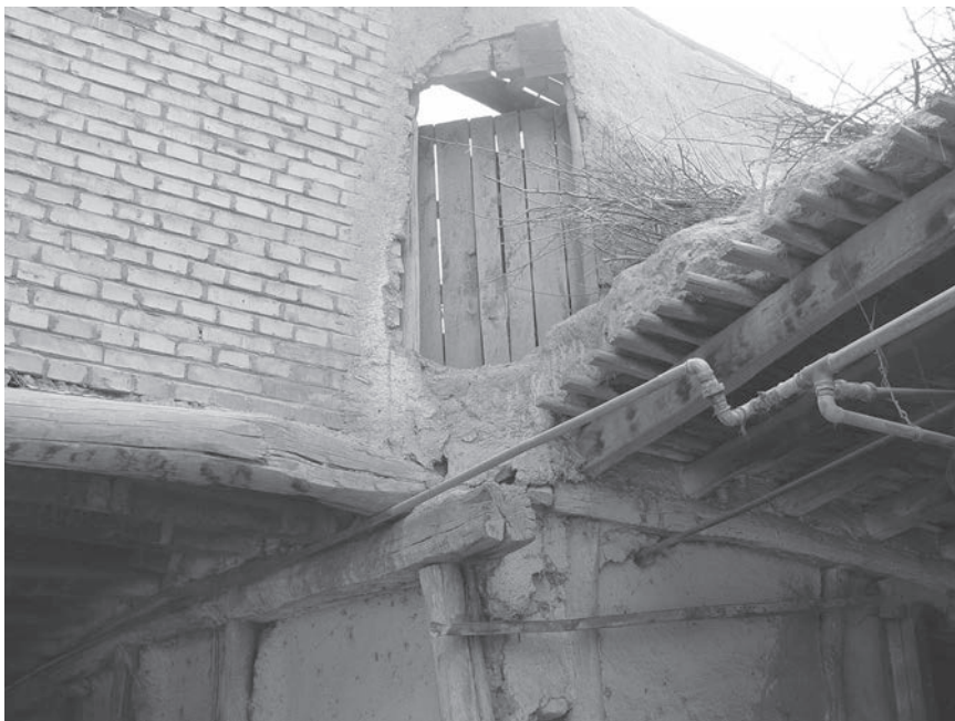
Figure 3.9 Jane Macartney quotes an old man from Kashgar who explained to her, tapping a mud-and-straw wall, that these structures have wood inside to absorb the seismic shocks: “These houses have withstood earthquakes for 2,000 years.” Photograph taken by a Kashgar resident during the destruction phase of traditional mud houses with timber supports to be replaced by concrete (name withheld).
