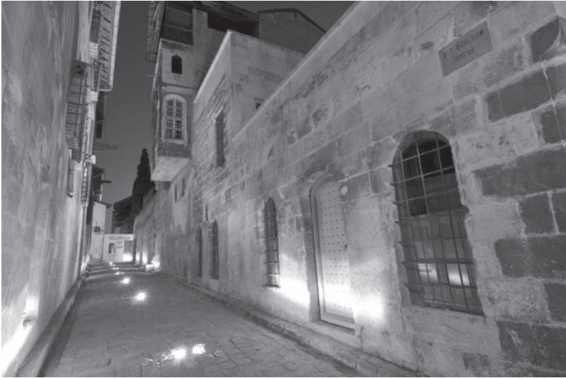
Figure 7.6 Involvement of the local authority in historic building conservation is one of the most efficient ways that community participation will increase residents' interest in historic preservation. The rehabilitation of the Bey Quarter in Gaziantep, Turkey, by the municipality of Gaziantep provides a good example. Image courtesy Gaziantep Municipality.
