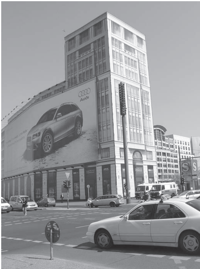
Figure 7.14 Leipzigerplatz in Berlin shows a type of façadeism where fake façades conceal empty sites. Image courtesy Peter Collier, Department of Geography, University of Portsmouth, UK.
