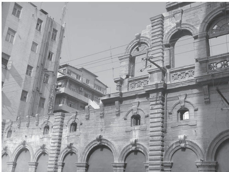
Figure 3.3 The absence of conservation area designation in Karachi has led to a rapid loss of colonial architecture and fusion architecture in the city. Courtesy Ayesha Agha Shah, University of Bahrain.
