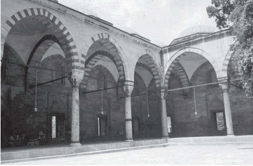
Figure 2.3 Fatih Mosque in Istanbul The arcades of the original mosque built in 1470 were reused by the Ottoman architect Mehmet Tahir Ağa in the eighteenth-century reconstruction following the earthquake of 1766. Image by Zeynep Aygen.
