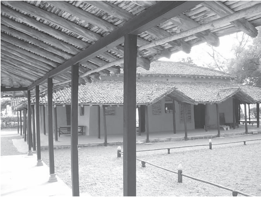
Figure 5.10 Sevagram Ashram Complex in Wardha, India, where Mahatma Gandhi lived during his mature years. It has been preserved thanks to the efforts of the community, and now the conservation architect Vikas Dilawari has developed a proposal based on reviving mud flooring and country tile roofing using bamboo matt traditions with the help of residents; it is a project in pipeline where the philosophy proposed is to follow the process rather than product. Image courtesy Vikas Dilawari.
