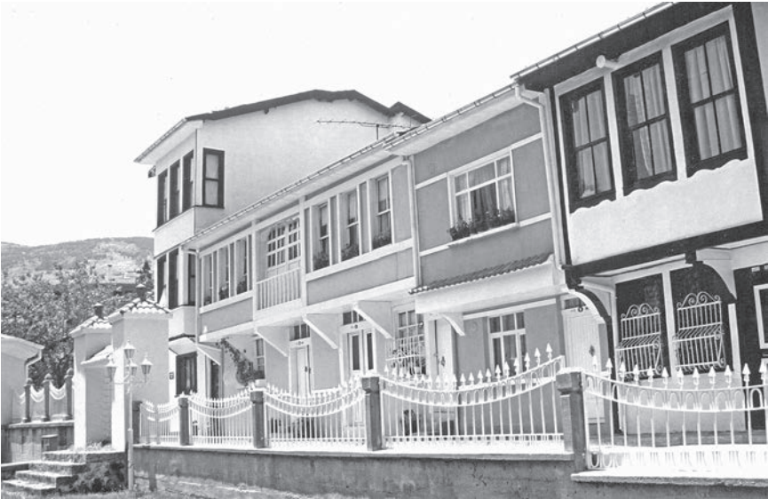
Figures 7.3 and 7.4 Osmangazi Street (before and after), another community participation project in Bursa by Basri Sönmez and Şaziye Sezginer. The project included locating cables underground, replacing asphalt with a traditional stone pavement, renovating the façades of the houses and greening the street, with the support of owners, tenants and shopkeepers. Images courtesy Basri Sönmez.
