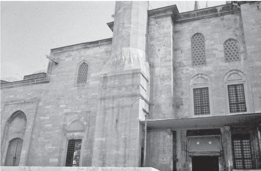
Figure 2.4 Fatih Mosque in Istanbul. Use of remaining fifteenth-century stones during the rebuilding of the minarets—an application of Burra Charter principles developed at the end of the twentieth century was developed in the eighteenth century by the Ottomans in practice. Image by Zeynep Aygen.
