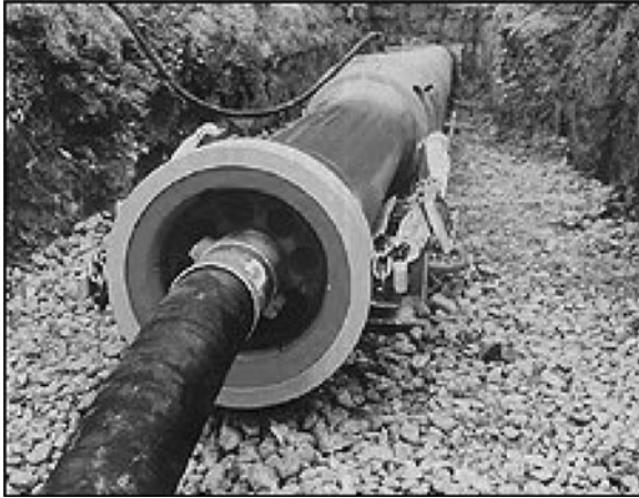
FIGURE 6-3. Casing installation with pipe ramming.
