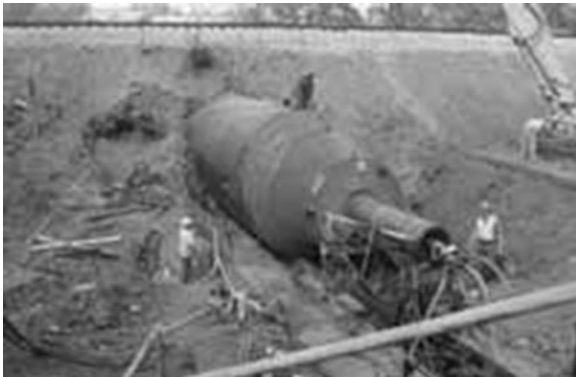
FIGURE 6-7. The 147-in. (3,734-mm) outside diameter casing.
