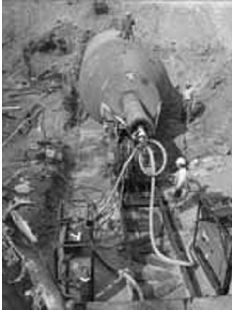
FIGURE 6-6. A 24-in. (610-mm) diameter ramming tool.
