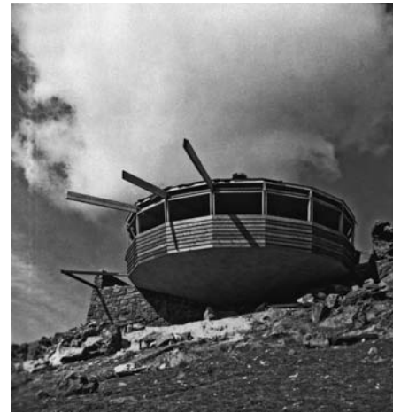
Construction of the Troutner House, Boise, Idaho 1955 Photo: Art Troutner. Used with permission.
