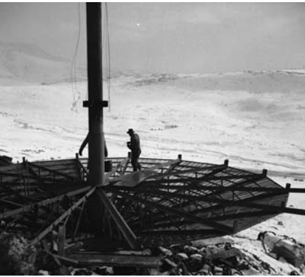
Construction of the Troutner House, Boise, Idaho 1955. Photo: Art Troutner. Used with permission.
