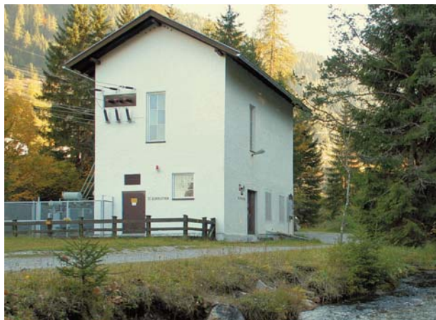
Fig. 12. Turbine house of the Austrian Biberwier/Tyrol hydropower plant using mine water of the Max-Braun-Adit located in the Silberleithe hills that can be seen in the background of the photograph. The first turbine to produce energy was installed in 1904; the currently operating turbine was installed in 1936.
