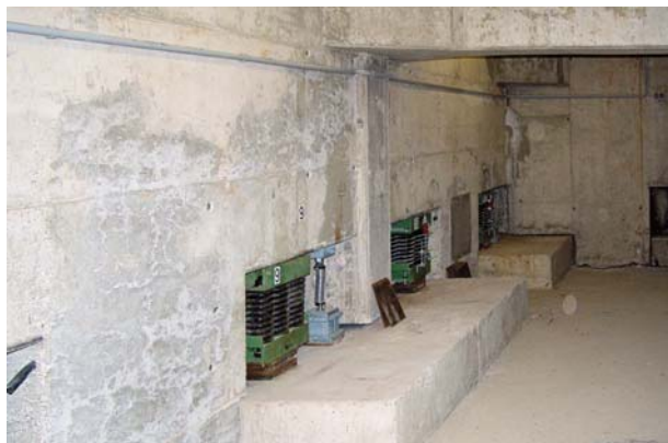
Fig. 34. Technical solution to secure a private house from destruction resulting from surface subsidence (courtesy Alexander Kattner, 25 March 2003).
