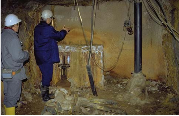
Fig. 22. An underground dam in the abandoned Königstein/Germany ISL uranium mine to prevent the discharge of highly acidic leachate fluid (8 January 1992).
