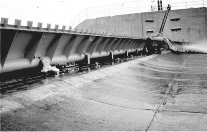
Figure 2-8. Single skinplate torque tube hinged crest gate (Courtesy of USBR).
