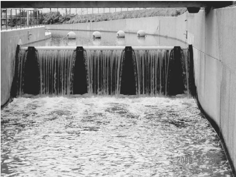
Figure 2-10. Double skinplate torque tube hinged crest gate.
