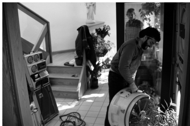
Blower door testing to check insulation and air-exchange provisions
