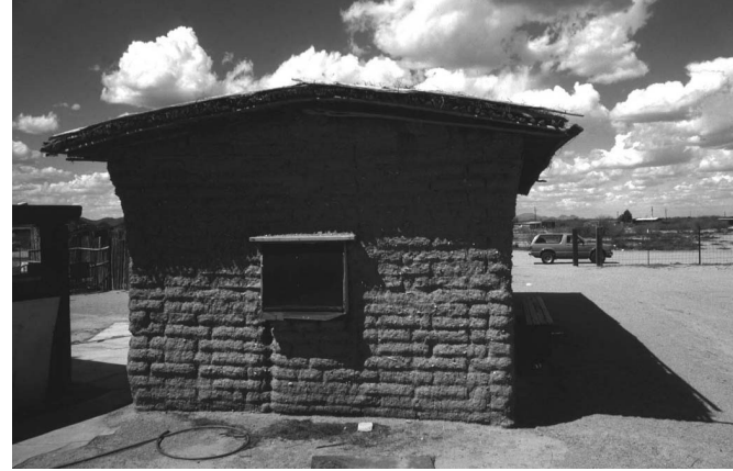
Fig. 12. Adobe home. Papago Indian Nation, Arizona. A centuries-old building tradition evident in informal house construction provides thermal time delay in hot-arid climate. Overhangs provide shading and protect the adobe
