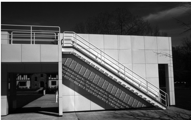
Fig. 6. Hartford Seminary. Ironwork and enamel panel construction. West Hartford, CT. Richard Meier, Architect.
