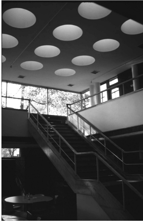
Fig. 6. Baker House Student Lounge, Massachusetts Institute of Technology, Cambridge, MA. Alvar Aalto. 1947. Splayed conical skylights provide substantial daylighting.
