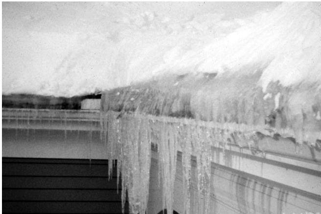
Fig. 14. Ice dam at eaves of steep roof. Thick deposit of ice causes melt water to back up and run through laps and joints in shingle roof. Eave flashing is intended to tolerate ice damming and prevent melting water from entering building.
