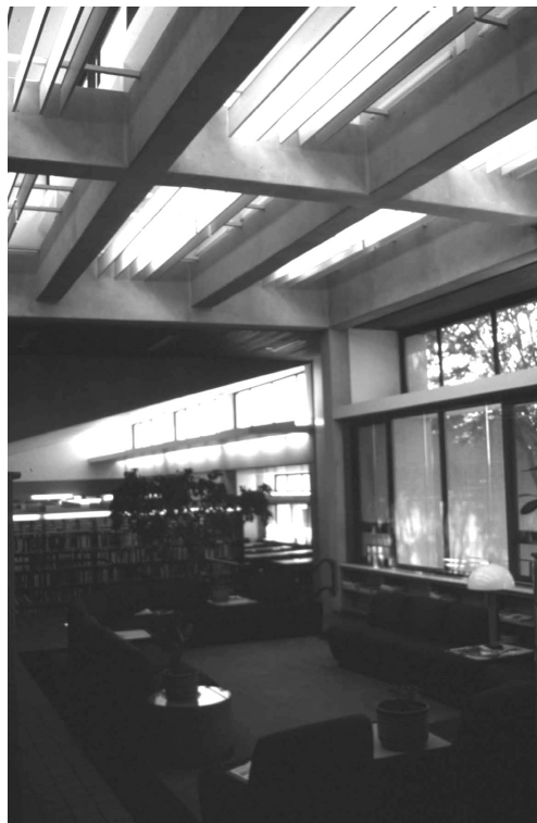
Fig. 7. South-facing clerestories with louvers. Public Library, Mt. Airy, NC. Mazria/Schiff, Architects. 1982. Louver baffles provide shading and light diffusion.
