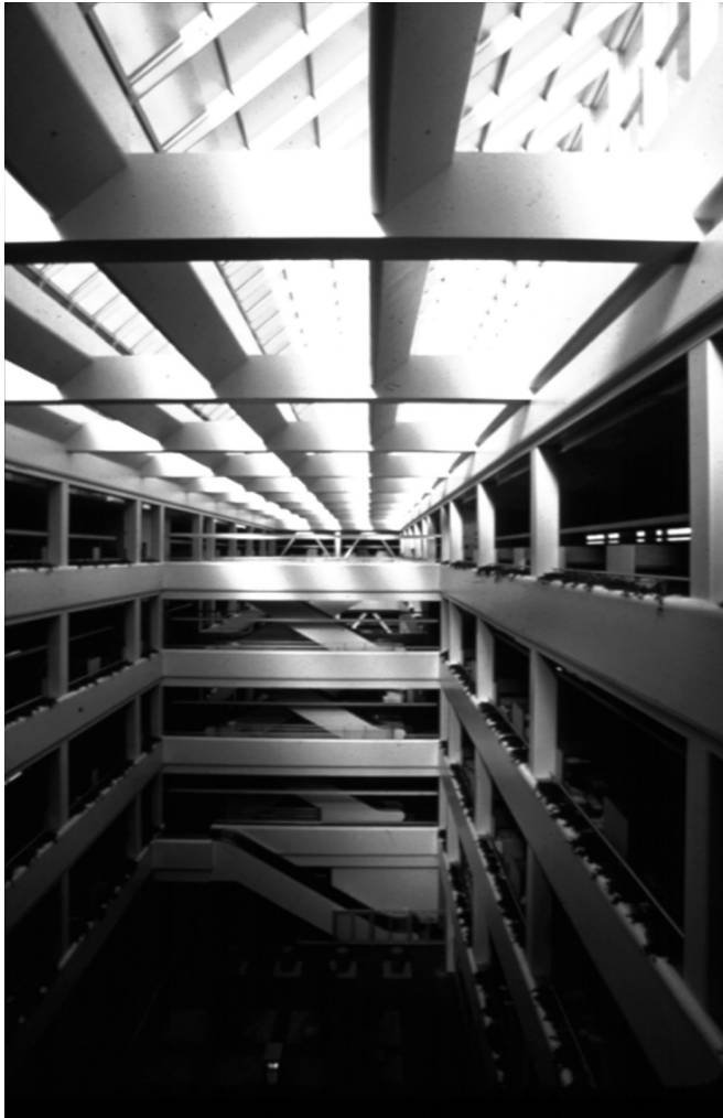
Fig. 8. The daylight-accepting atrium of Lockheed Building 157.
