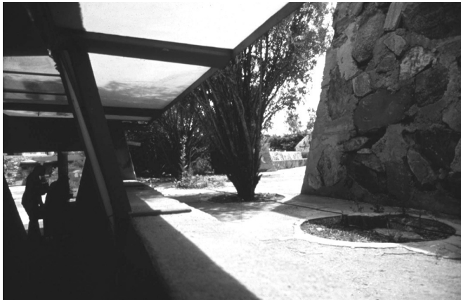
Fig. 16. Taliesin West. Scottsdale, AZ. Movable shading and subgrade thermally massive construction create a cooling microclimate. Frank Lloyd Wright, Architect.
