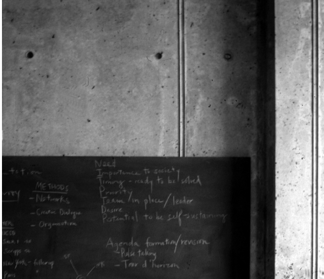
Fig. 10. Interior detailing of concrete form joints. Salk Institute, La Jolla, CA. Office of Jonas Salk. Louis Kahn, Architect.
