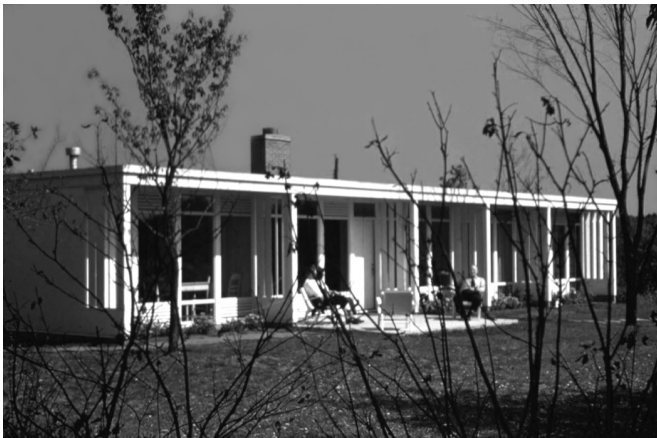
Fig. 9. Green Pre-Fab Homes, Rockford, IL, 1944. The first to be called “solar houses,” Architects George and William Keck’s home designs, beginning in the mid-1930s, combined south-facing glass, sun shading and internal thermal mass.
