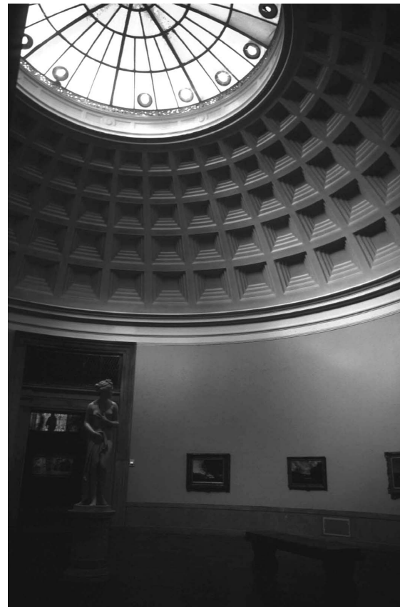
Fig. 5. Corcoran Gallery, Washington, skylight modeled after the dome of the Pantheon. Shadowing provided by the coffers allows the eye to adjust to its lighting intensity.
