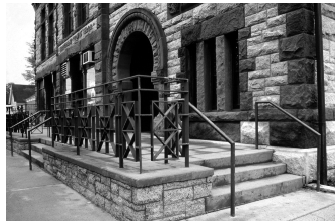
Fig. 5. Entry terrace modifications, including ramp and handrails, blending with historic design. Hopedale Town Hall, Hopedale, MA. Nichols Design Associates, Architects.
