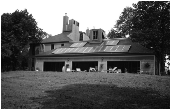
Fig. 28. Solar heating for a pool house. Private Residence, CT. Architect: Charles W. Moore, FAIA. Solar design and engineering: Everett M. Barber, Jr. 1973.
