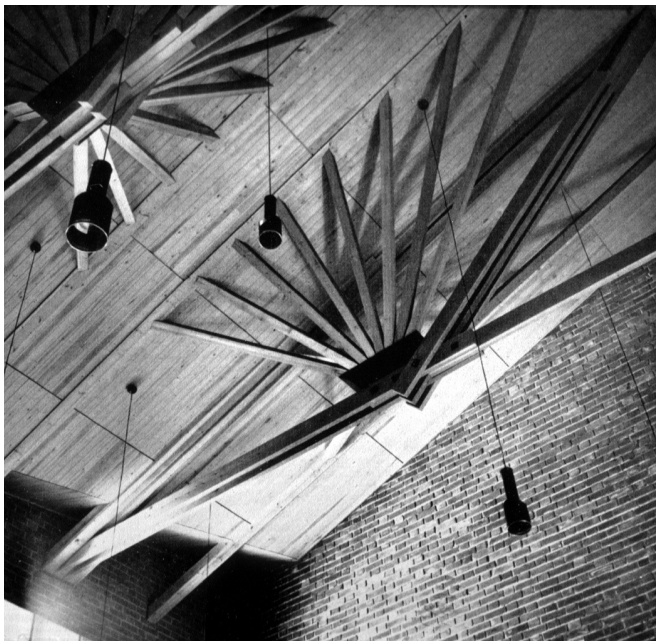
Fig. 4. Expression of structural truss. Saynatsalo Town Hall.
