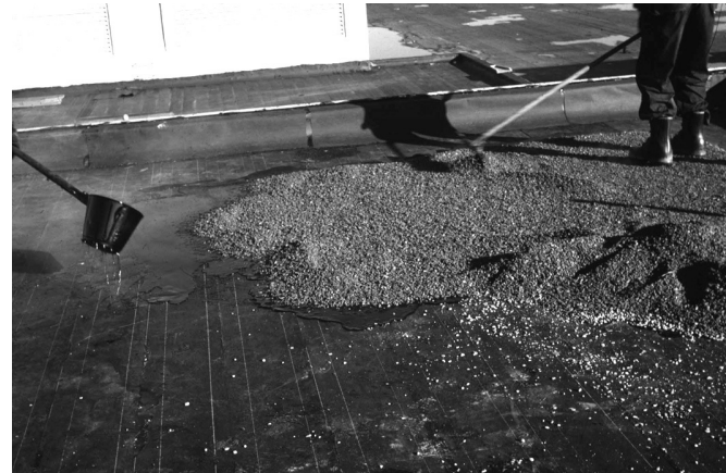
Fig. 2. Pouring asphalt over built-up roof felts, and embedding gravel aggregate.
