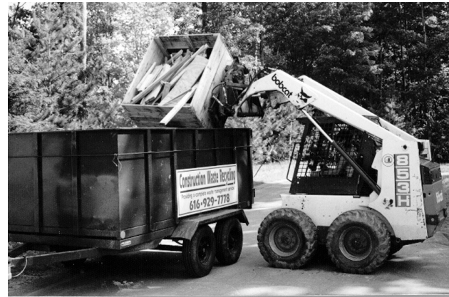
On-site separation of wood scraps for recycling. photo: NAHB/RC
