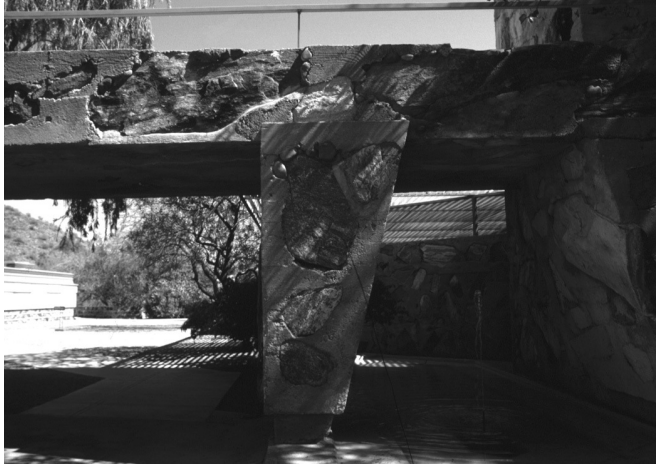
Fig. 5. Taliesin West. Scottsdale, AZ. Masonry construction. Frank Lloyd Wright, Architect.
