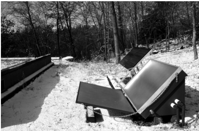
Fig. 27. Batch water heater with adjustable reflecting cover panel on an earth-covered home. New Canaan, CT. 1982.
