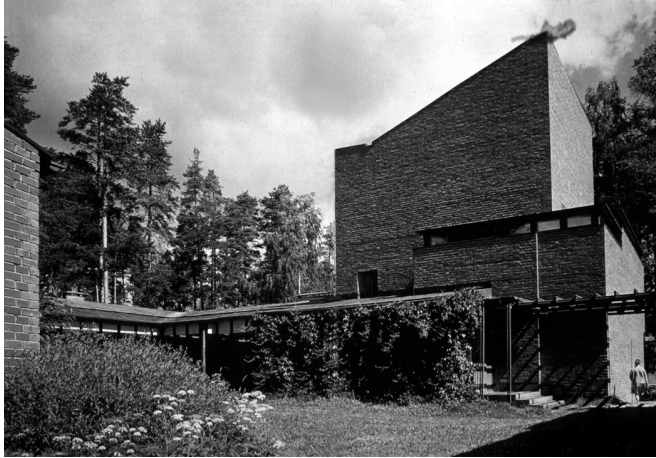
Fig. 3. Town Hall. Saynatsalo, Finland. Alvar Aalto, Architect. 1949-52.
