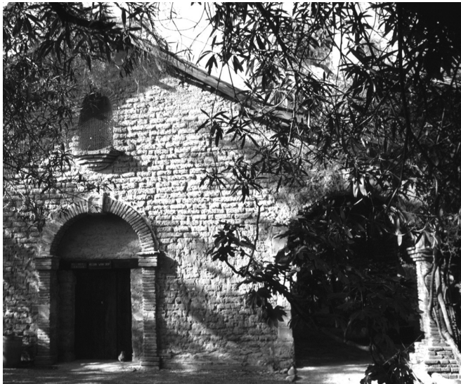
Fig. 2. Adobe block and brick construction. Spanish Mission, Capistrano, CA.
