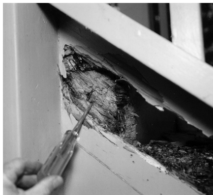
Fig. 4. Termite damage
