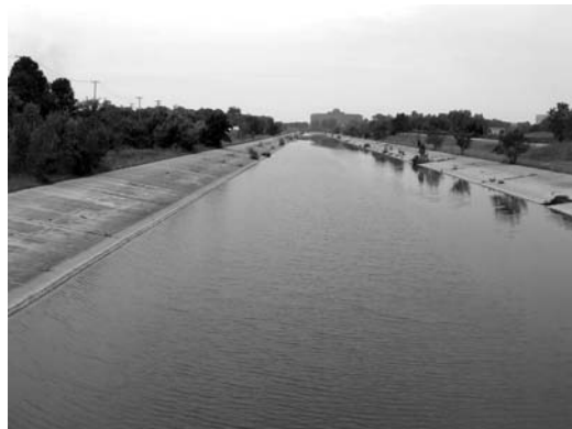
FIGURE 15.4 Channelized portion of an urban river. (Photo by Kent S. Murray.)
