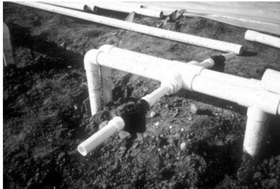
FIGURE 11.3 Electronic valves control fresh air circulation in a treatment cell. (Photo by Kent S. Murray.)
