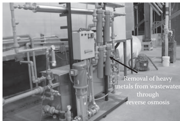
FIGURE 13.11 Reducing heavy metals in wastewater. (Photo by Daniel T. Rogers.)
