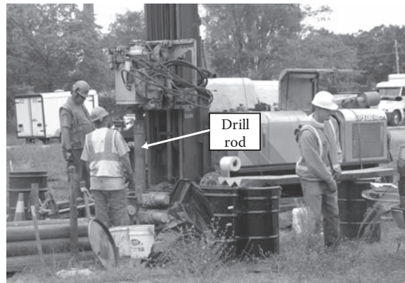
FIGURE 4.13 Roto-sonic drilling rig. (Photo by Daniel T. Rogers.)
