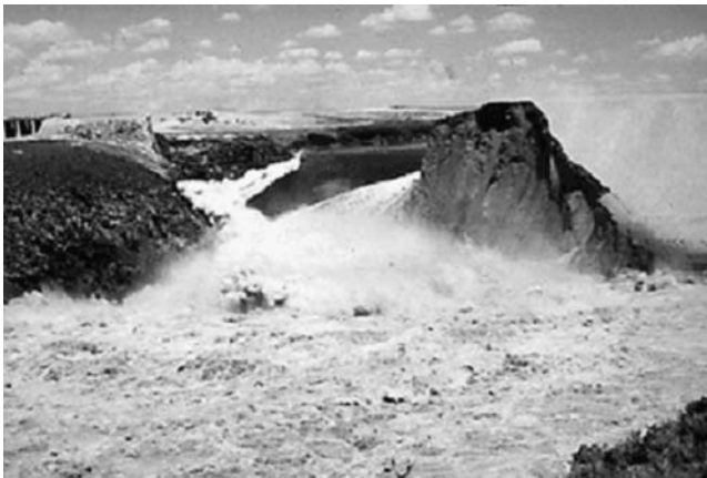
FIGURE 3.50 Teton Dam failure. (Photo by Mrs. Eunice Olsen, June 5, 1976.)
