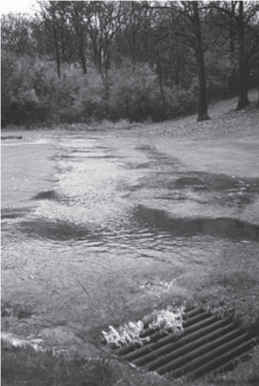
FIGURE 9.2 Runoff from a compacted urban soil. (Courtesy of nih.gov.)
