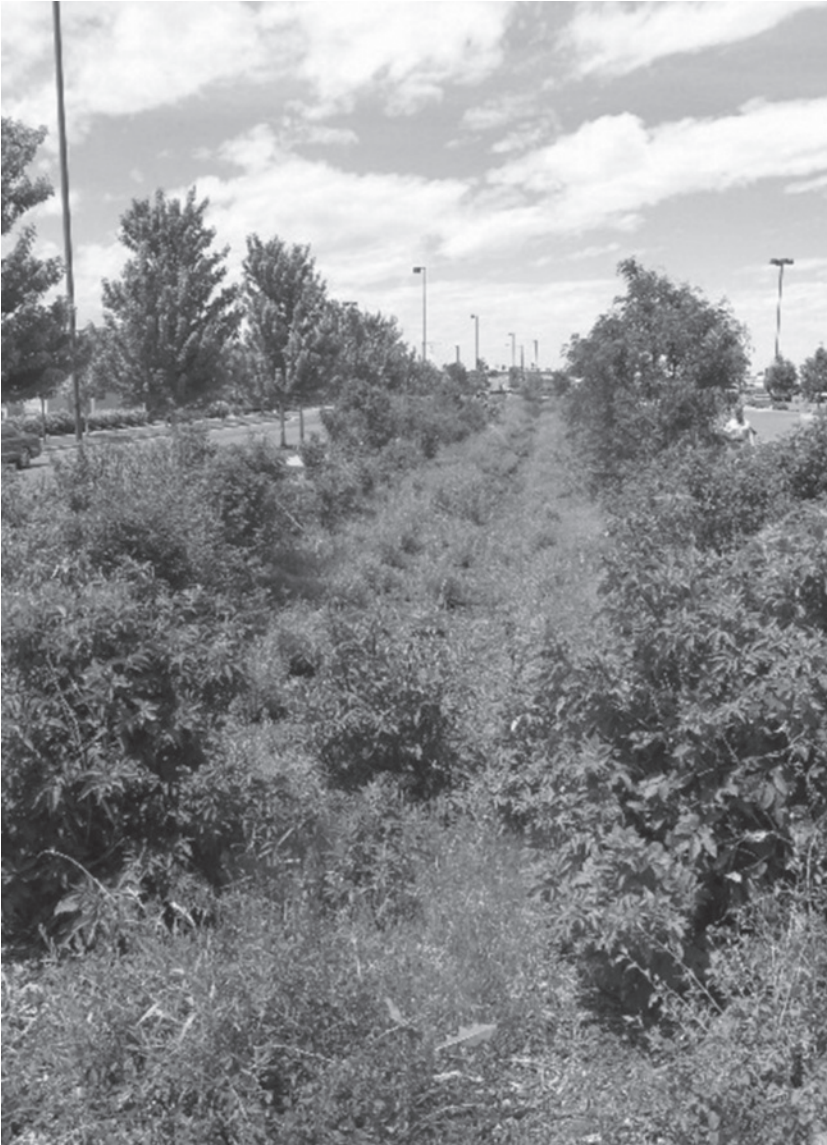
FIGURE 9.4 Bioswales, like this in Denver, CO, and other vegetated patches in the urban landscape help infiltrate rainwater and encourage optimal soil hydrologic properties by improving soil organic matter, porosity, and structure. (Courtesy of epa.gov.)
