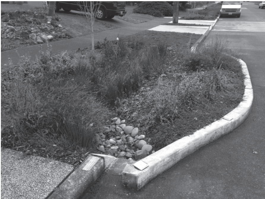
FIGURE 10.5 A bioretention system for stormwater in Seattle, WA.
