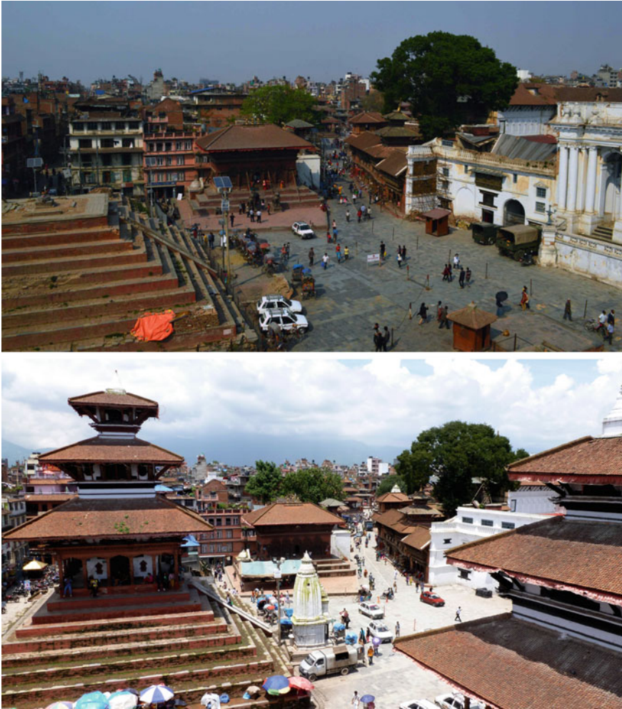
Fig. 8.1 Kathmandu Durbar Square before and after the earthquake ( top taken April 2016, source Rupesh Shrestha, bottom taken April 2013)
