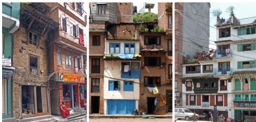
Fig. 5.8 Examples of vertical division and addition of storeys on traditional houses in Kathmandu Centre
