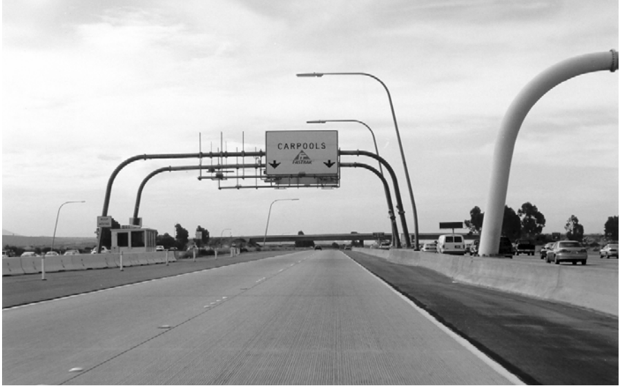
Figure 4.11 The HOT lane on Interstate 15 to San Diego, segregated from other traffic (to the right)
