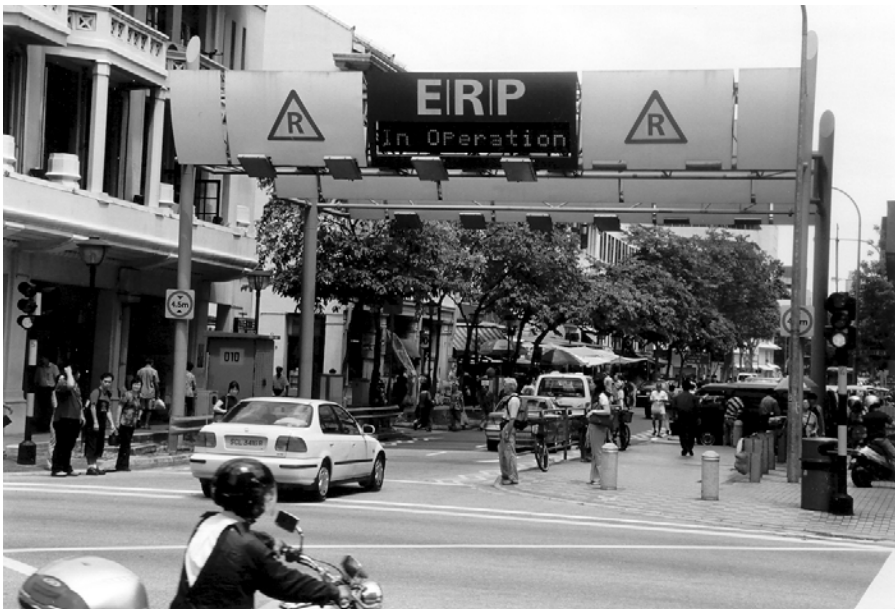
Figure 4.6 An Electronic Road Pricing entry gate in Singapore. These are purposefully conspicuous to ensure that motorists know they are entering the charge area
