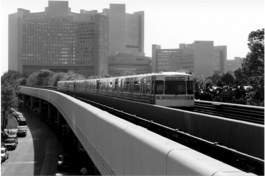
Figure 3.1 A new section of the Vienna Metro. The cost of the Vienna Metro was partially met by the Dienstgeberabgabe Employer Tax
