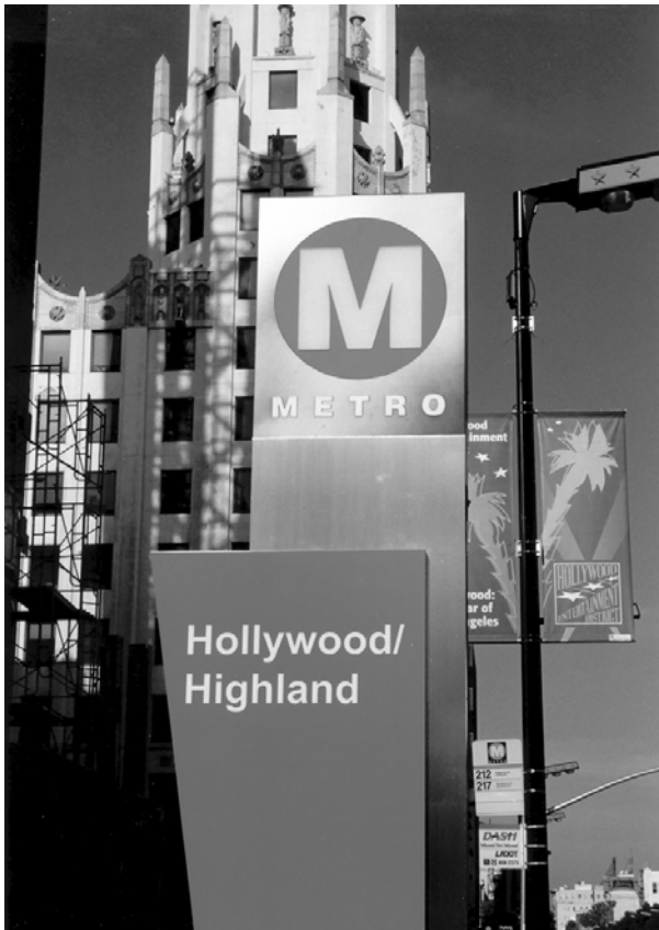
Figure 2.3 New Metro Station in Los Angeles – a classic case of difficult and expensive public transport operating territory
