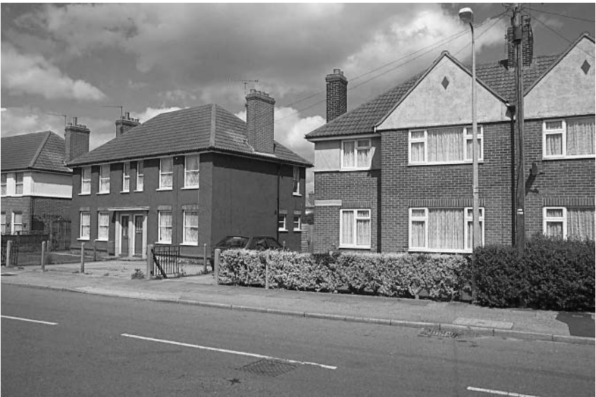
Picture 2.8 Town, semi-detached houses
