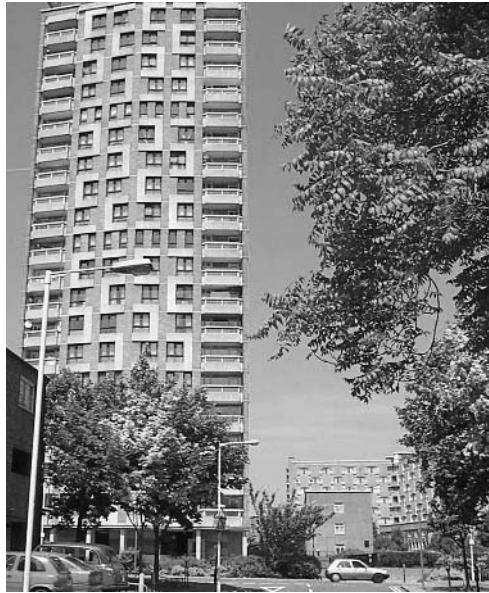
Picture 2.4 City, tower block
