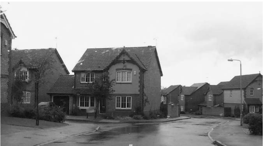
Picture 2.20 Suburb, detached houses
