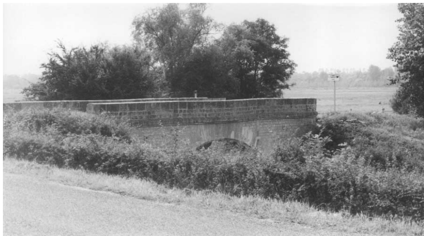
Photo 13.1 Bridge over Merderet River at La Fièvre
