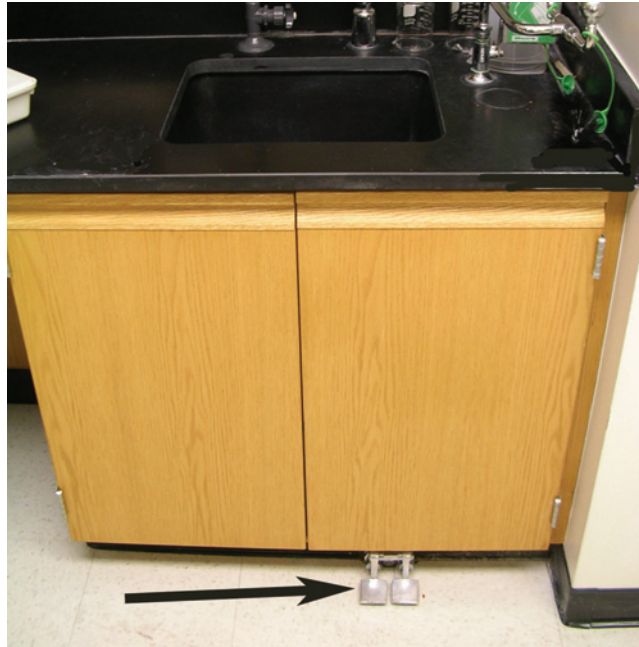
FIGURE 26.4 All sinks in the cell culture areas are foot-pedal controlled (arrow), allowing hand-washing without contamination of or by fixtures.
