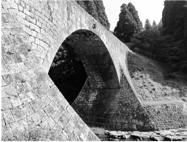
FIGURE 21.12 Tsujun Bridge and arch structure.
