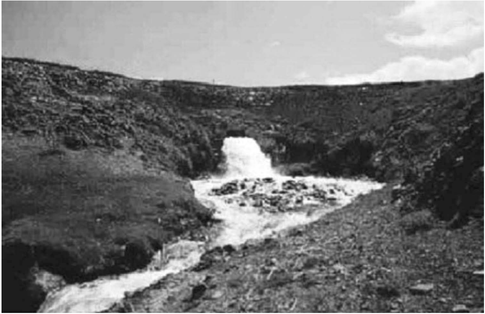
FIGURE 18.5 Bottom sluice of Rusa Dam today (constructed 700 BC).
