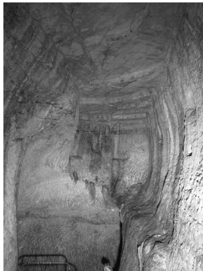
FIGURE 5.8 The face of the north bore at the meeting point. At the bottom of the picture is the south bore eastside. The face of the south bore is at the bottom-left corner.
