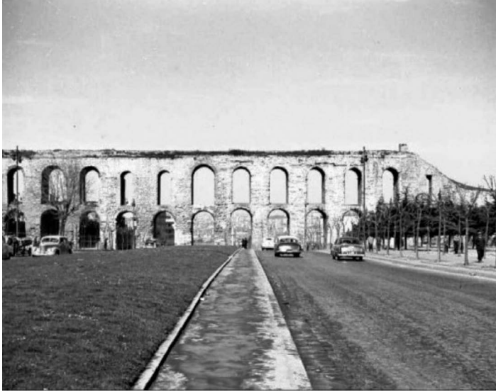
FIGURE 15.7 Bozdoğan (Valens) aqueducts.
