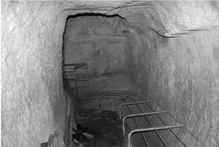
FIGURE 5.9 The south face at the meeting point. The marks of the two miners working side by side are visible. The north bore emerges at the left side of the picture.
