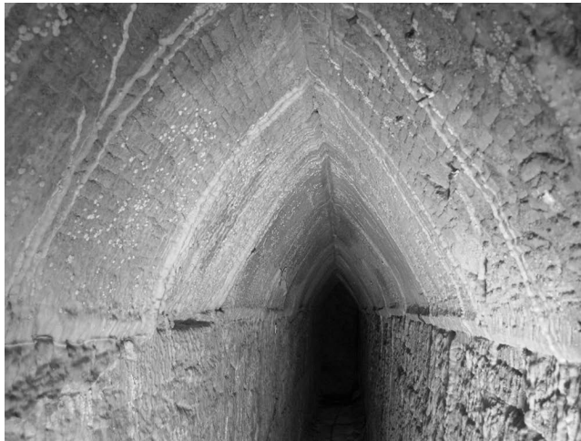
FIGURE 5.12 Perfectly fitting and beautifully curved archaic masonry lining.
