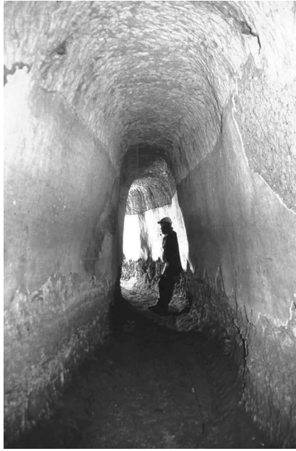
FIGURE 11.20 Plastered tunnel near Abila.
