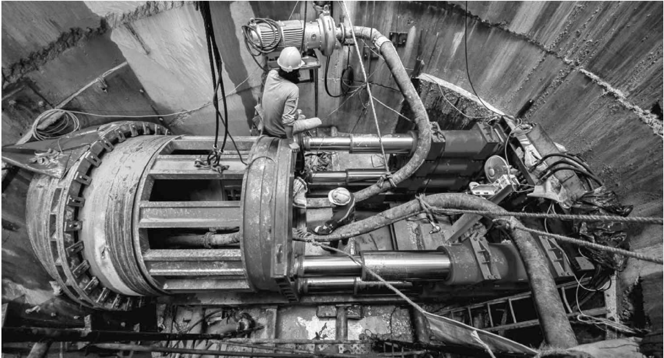
FIGURE 26.5 Slurry microtunneling at 14 m depth (water transmission pipelines from east side of Chao Praya river to the Bang-Pra reservoir). (Courtesy of Thai Triumph, 2015.)
