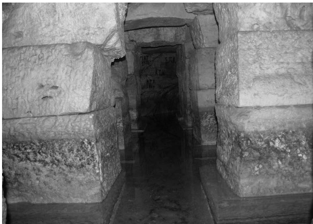
FIGURE 5.3 The interior of the cistern. The mineral and organic deposits on the surface of the pillars indicate the variation of the water level.
