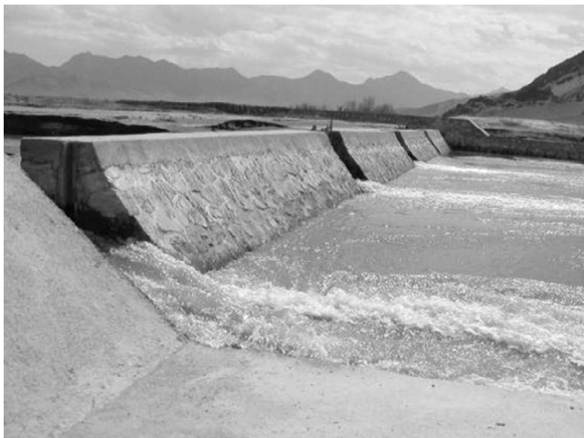
FIGURE 22.5 New dam on the Logar River.
