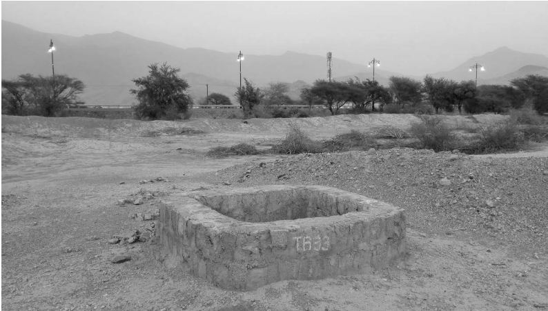
FIGURE 12.6 The mother well, Umm Al-Falaj, of the underground aqueduct Falaj Daris in Nizwa (Oman). (Courtesy of Megdiche-Kharrat 2015.)
