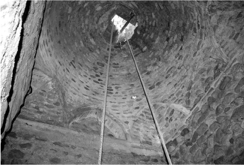
FIGURE 19.5 Architectural elements on the 40-stairs dome Shai, Ordubad. (From Guliyev, A.G. and Hasanov, A.M., International Conference on Traditional Knowledge for Water Resources Management , Yazd, Iran, 2012.)
