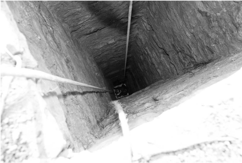
FIGURE 2.12 Vertical shaft of “Ravne njive” tunnel. (Courtesy of T. Bartulović.)
