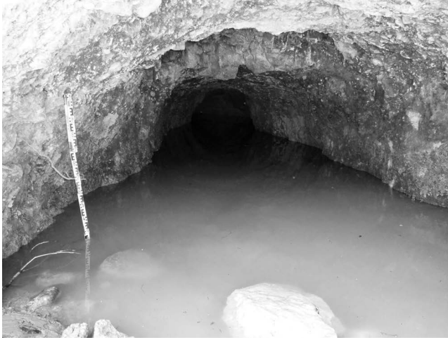
FIGURE 10.8 El-Balad spring. A hewn spring tunnel, 4 m wide. (Photography by Yechezkel.)
