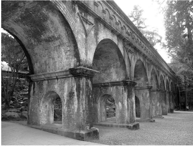
FIGURE 21.15 Brick-masonry arch bridge in Biwako Canal.
