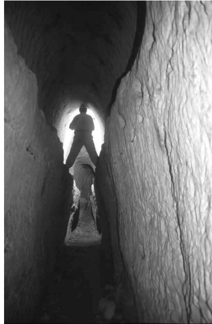
FIGURE 11.13 Errors in height calculation: Above, the tunnel that was laid too high.
