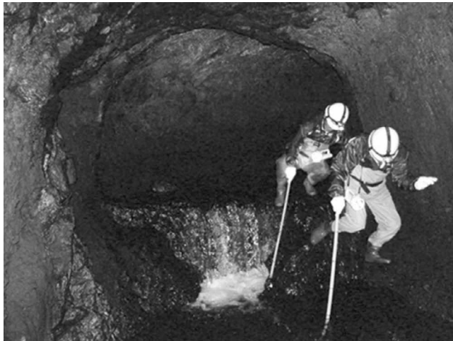
FIGURE 21.11 Heritage study tour at the breakthrough point in Fukara Tunnel (From HP/Wikipedia, Fukara Aqueduct, 2015b. With Permission.)
