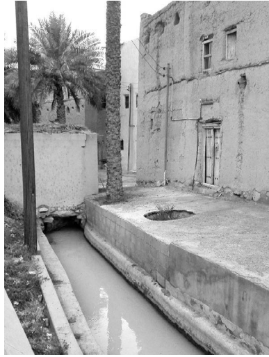
FIGURE 12.7 Water of the underground aqueduct Falaj Daris temporarily affected (for a few seconds). (Courtesy of Megdiche-Kharrat 2015.)
