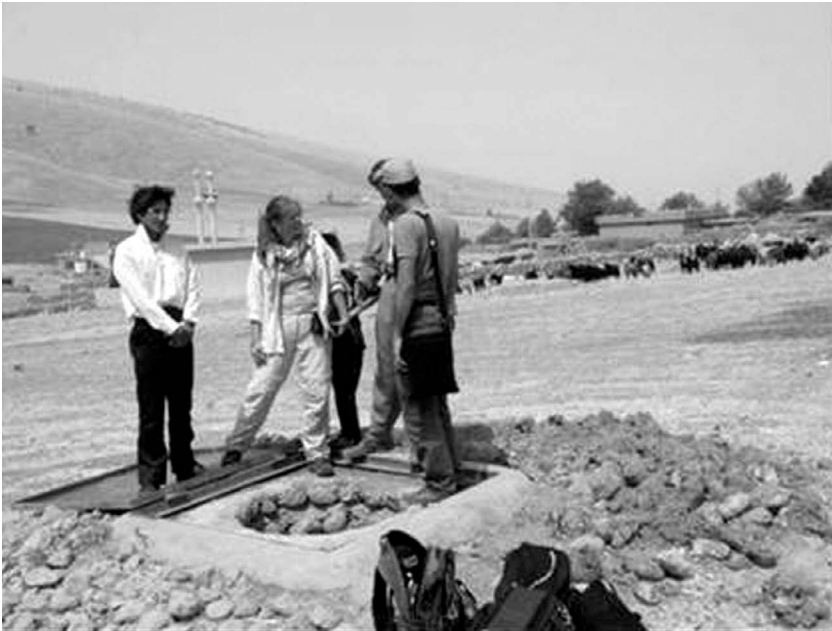
FIGURE 29.6 Iranian/Dutch team of qanāt experts rehabilitating a qanāt in Kurdistan, 2010/2011 for a UNESCO qanāt renovation project.
