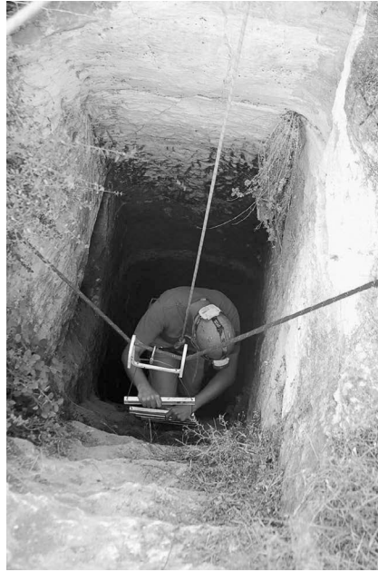
FIGURE 11.3 Entrance into a construction shaft at 'Alcāl.
