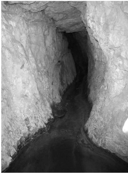
FIGURE 10.9 El-Habis spring. A hewn spring tunnel roofed with stone slabs. (Photography by Yechezkel.)
