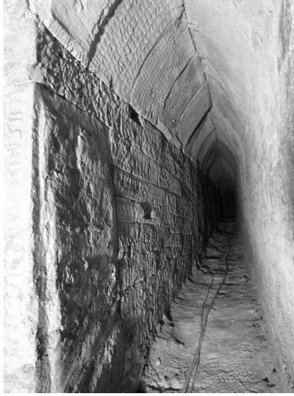
FIGURE 5.11 The archaic lining between Ch. 245 and Ch. 263, with the characteristic treatment of the surfaces of the stone blocks.
