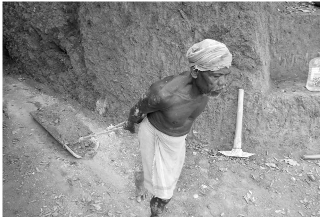
FIGURE 24.3 A suranga under construction.
