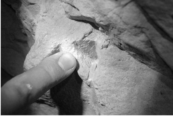
FIGURE 11.18 Mark left by a quadratic moil chisel.
