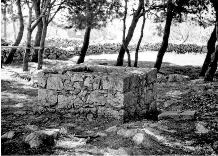
FIGURE 2.17 Shaft no. 7 of Navalja aqueduct tunnel. (From Ilakovac, B. VAMZ , 3.s., XLI, 129–166, 2008. With Permission.)
