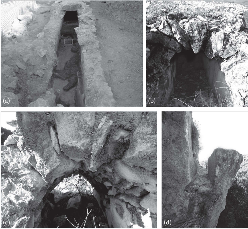
FIGURE 4.13 The aqueduct’s channel. (a) At Prineri Katifori. (b) At the Roman quarry. (c) Detail of the channel’s vaulted top. (d) At Kourtzi thermal springs. (By permission of Y. Kourtzellis.)
