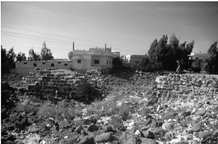
FIGURE 11.5 The west dam made from basalt blocks.
