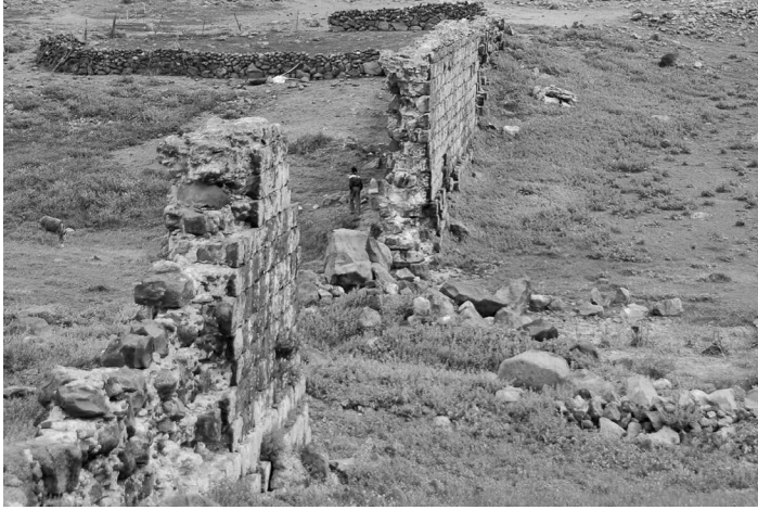
FIGURE 11.6 Aqueduct bridge over the Wādī Qanawāt. The middle section has collapsed.
