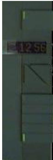
Figure 10: User interface unit for the Luxmate control system in the Intelligent Workplace. The topmost button is to activate the lighting; the two buttons in the middle allow increase/decrease in light levels, and the five buttons below that correspond to five programmable “scenes”.
