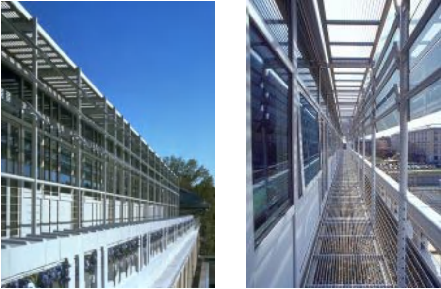
Figure 6: The Robert L. Preger Intelligent Workplace at Carnegie Mellon University has a layered enclosure, with dynamic light-redirection louvers, operable windows, high visibility glass, and internal shading devices, to maximize daylighting and solar control
