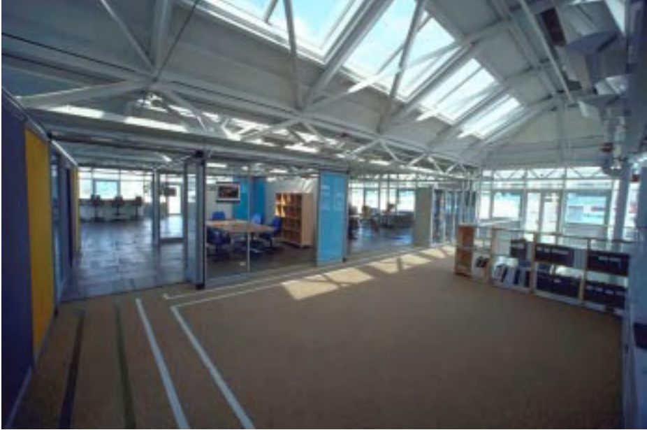
Figure 3: Interior view of the Robert L. Preger Intelligent Workplace. 75% of the façade area is glazed with high-visibility glass, maximizing daylight use throughout the year.
