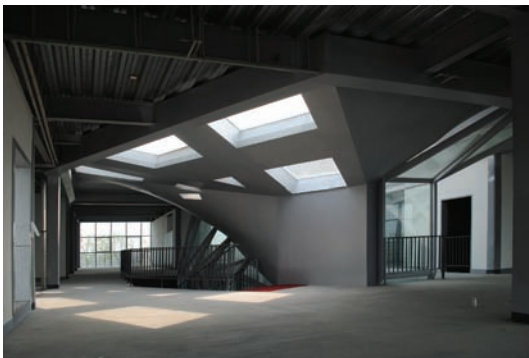
Figures 25.26–25.27 Interior view and details of inner GFRC light well
