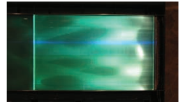
Figure 6.23 Controllable RGB LED modules at each lite of glass enable color definition to be both precise and dynamic
