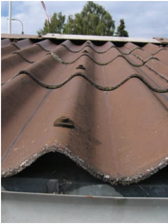
Figure 5.5 Future trends in Danish roof construction: fiber tiles bolted straight into metal framing
