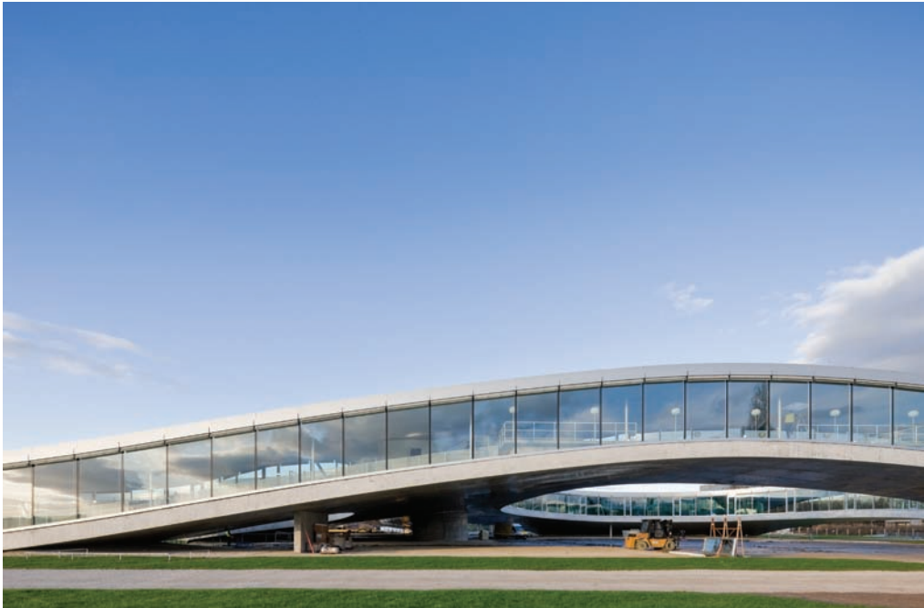
Figure 13.4 SANAA, Rolex Learning Center , Lausanne, Switzerland, 2010. Here the sheets repeatedly depart from the ground plane to define space beneath the building volume and alter the silhouette drawn by the roof plane
