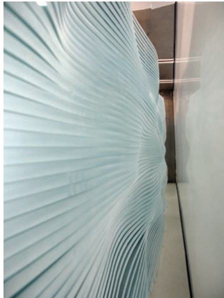
Figure 6.10 Smooth gradient of curved back side of glass
