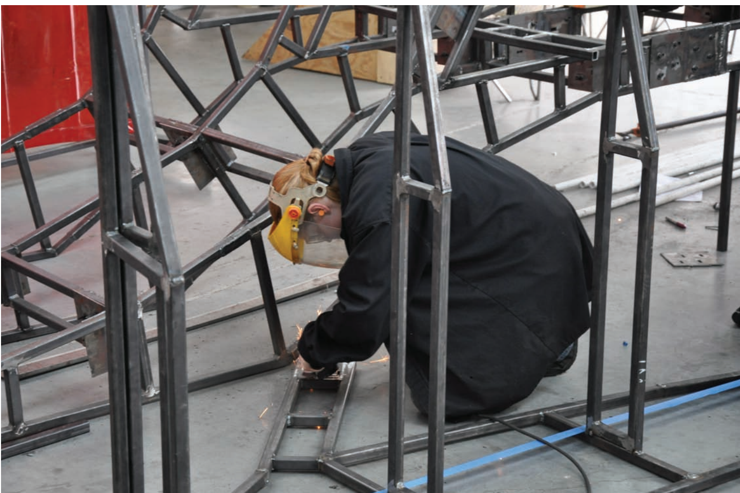
Figure 23.4 Welding Microliving frame, Houston, 2009
