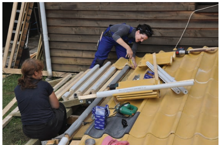
Figure 5.18 Walk-on test of construction. At this point the surface was quite flat so the performance was deceptively good
