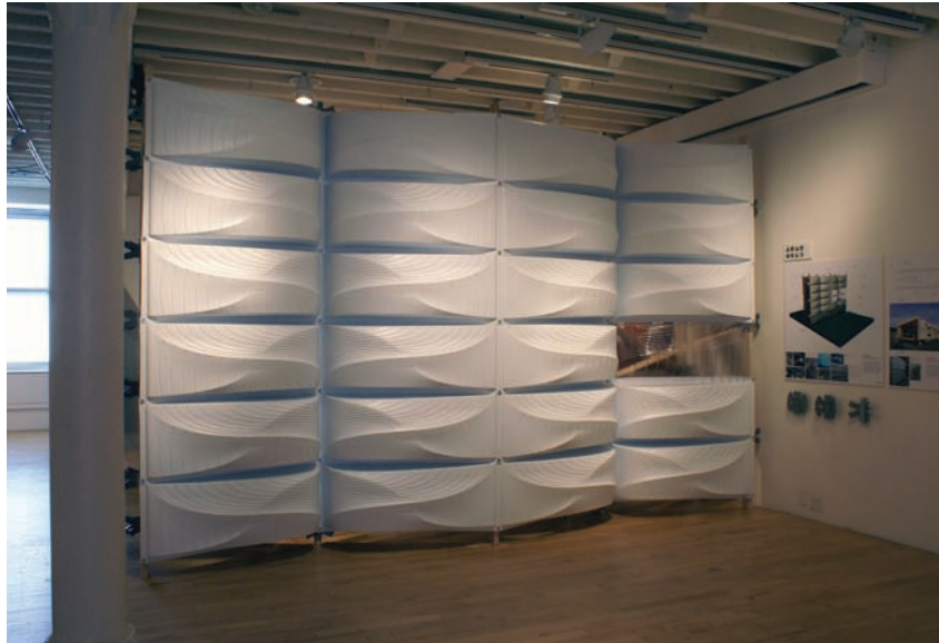
Figure 18.15 OSWall prototype. The exterior of OSWall , as seen at the Pratt Manhattan Gallery, NY. Vacuum formed panels arrayed over a two-by-four timber frame
