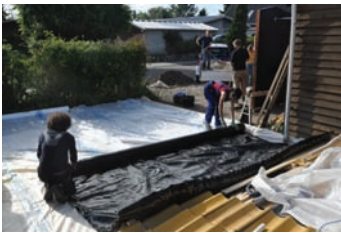
Figure 5.20 The basin membrane being laid out. The ground was flattened, removing twigs and roots and filling any dips with sand, then a layer of polyethylene felt underlayment preceded a thick layer of EPDM liner molecularly bonded along the seam with tape from the manufacturer
