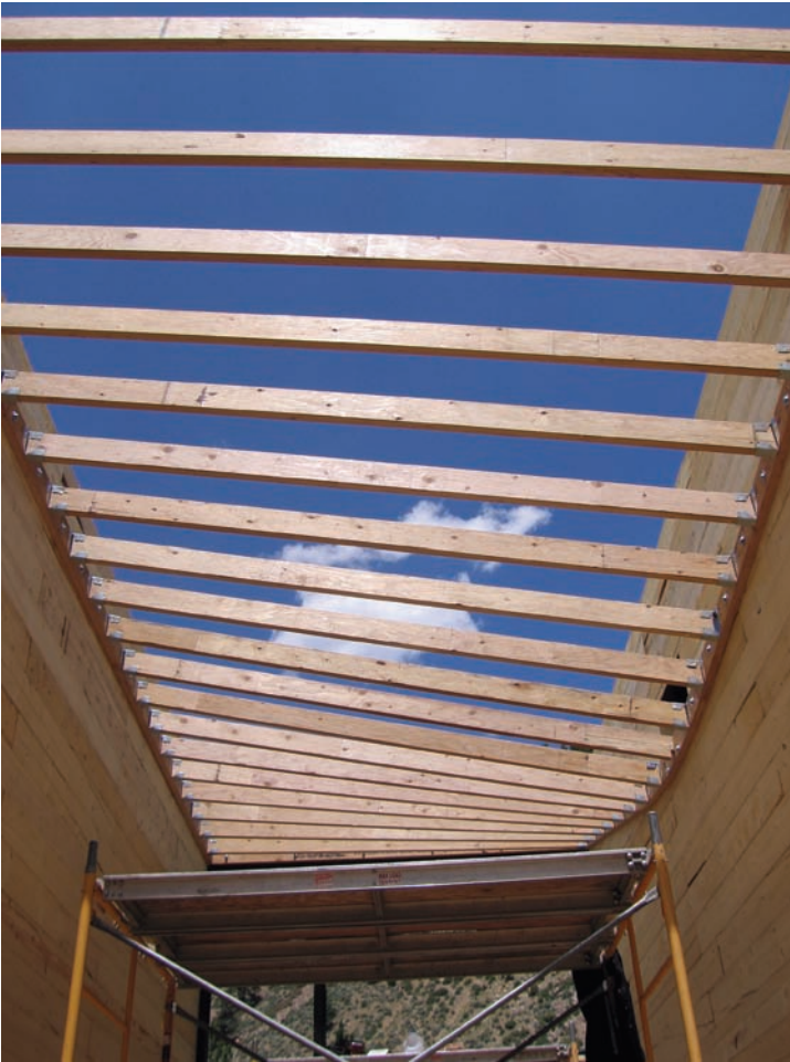
Figure 19.12 Roof framing from below Figure 19.13 Ceiling view
