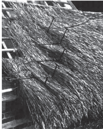
Figures 1.6–1.7 Separating bunches during thatching
