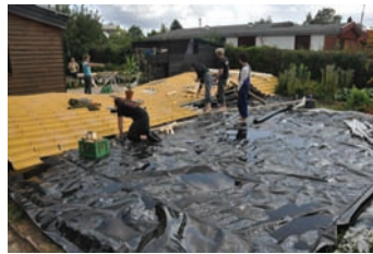
Figure 5.20 The basin membrane being laid out. The ground was flattened, removing twigs and roots and filling any dips with sand, then a layer of polyethylene felt underlayment preceded a thick layer of EPDM liner molecularly bonded along the seam with tape from the manufacturer
