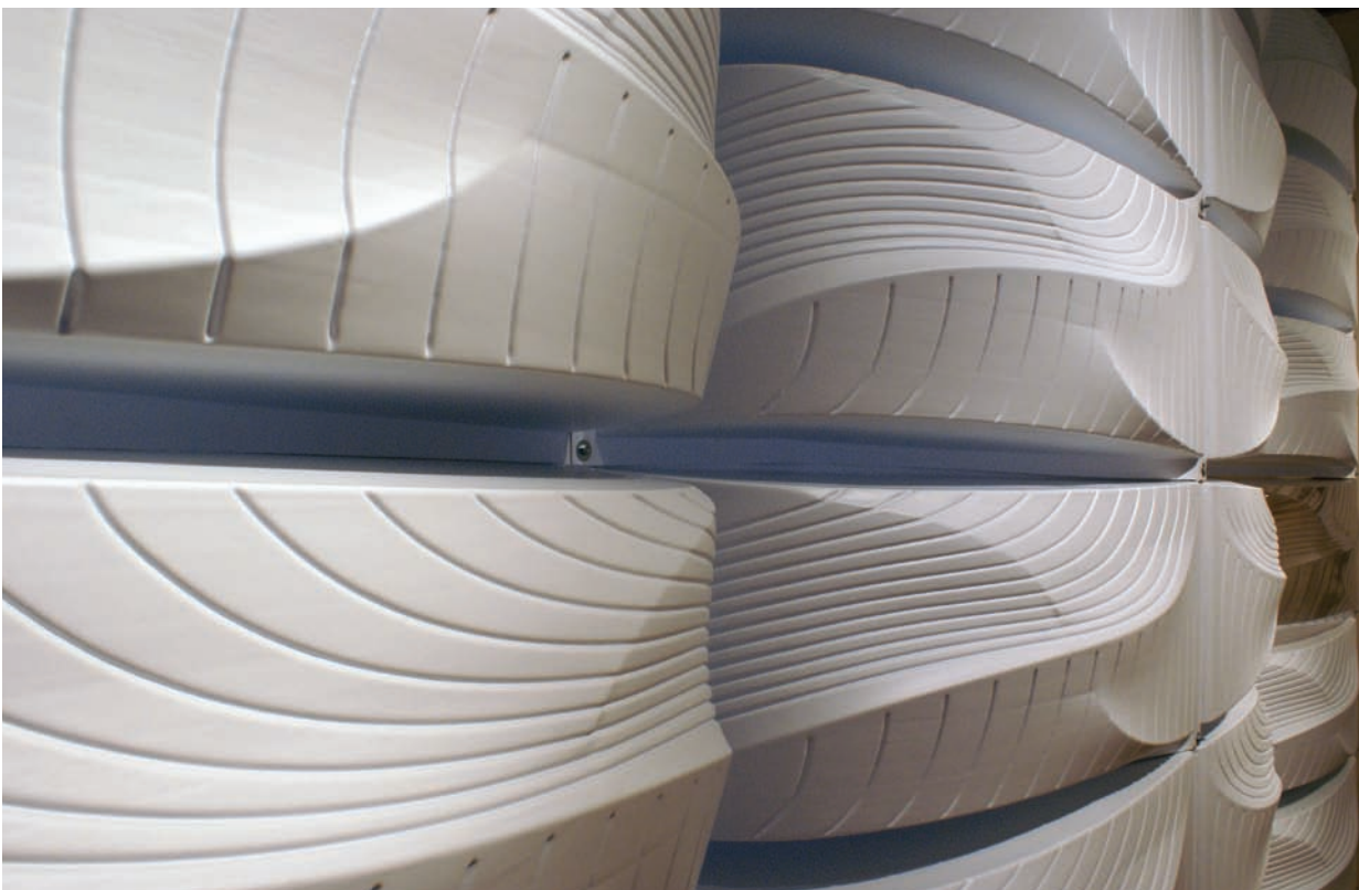
Figure 18.10 OSWall exterior. A formal skin pattern developed to channel water into storage bladders at the base of the wall construct. The pattern was informed by whale anatomy. Ridges and folds on the whale’s body allow the animal to expand its throat when feeding. The same ridges streamline the animal
