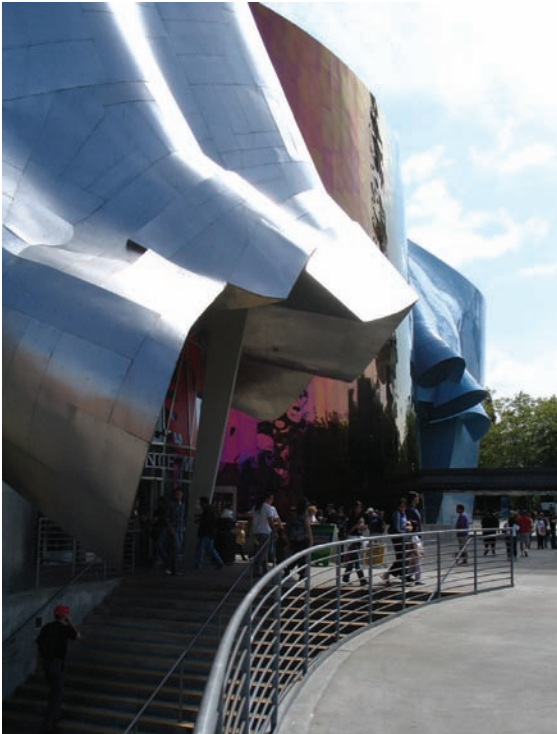
Figure 13.6 Frank O. Gehry and Associates, Experience Music Project , Seattle, USA, 2000. Sheet manipulations occur at the master plan scale to accommodate the arrival of rail transportation, connect the museum to the park, and respond to vehicular flows. Other modulations occur between building and ornament scale to define areas of pedestrian intensity
