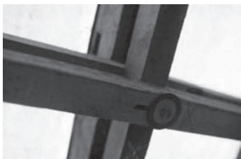
Figure 14.4a–b Frei Otto, Multihalle , Mannheim, 1975, detail
