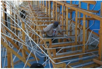
Figure 17.11 Live Wire . A wood jig was constructed to support the individual tubes prior to being welded together. Because the system of fabrication involved creating a joint between each bend in the tubes, the jig was an essential in ensuring the overall three-dimensional geometry
