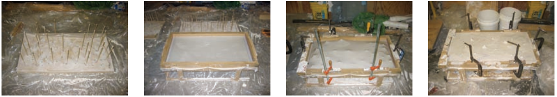
Figure 30.9a–d Fabrication sequence (from left): base constraint point template, lower support frame, upper fabric frame, cast panel in mold
