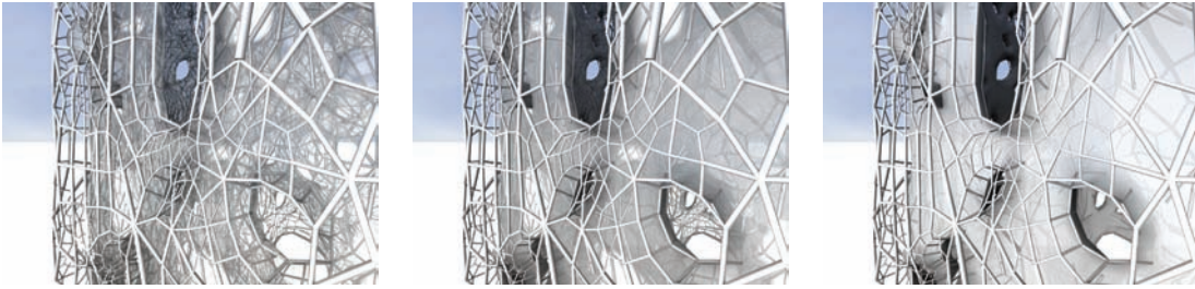
Figures 29.9–29.11 Close-up sequence showing transformation of exposed inner building surfaces through the crystalline build-up of salt
