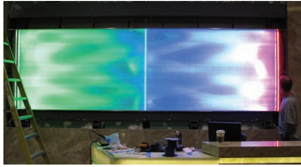
Figure 6.19 The effect of color fades and washes are a result of the controlled by RGB LED modules at each layer of glass in combination with the curvature of the backside of the glass
