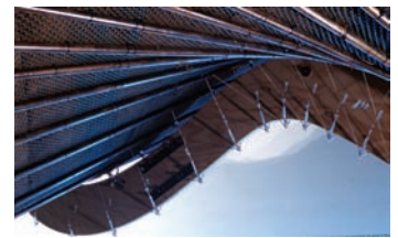
Figure 16.18 Detail view of supports
