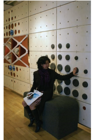
Figure 18.18 OSWall prototype detail. Here a responsive pattern of holes provides space for storage bags
