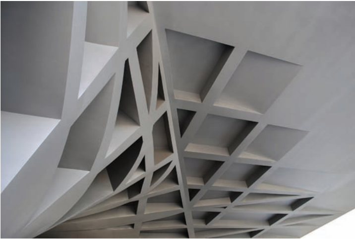
Figures 25.20–25.21 GFRC coffered torque surfaces seen from underneath
