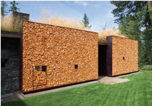
Master House (counterclockwise from top): Entry courtyard at dusk Entry courtyard looking northwest North facade of courtyard
