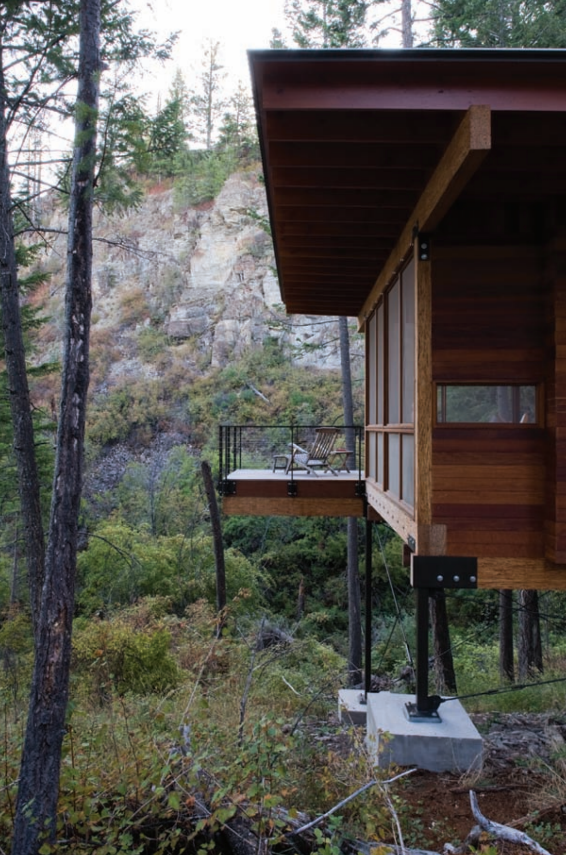
View of deck from below
