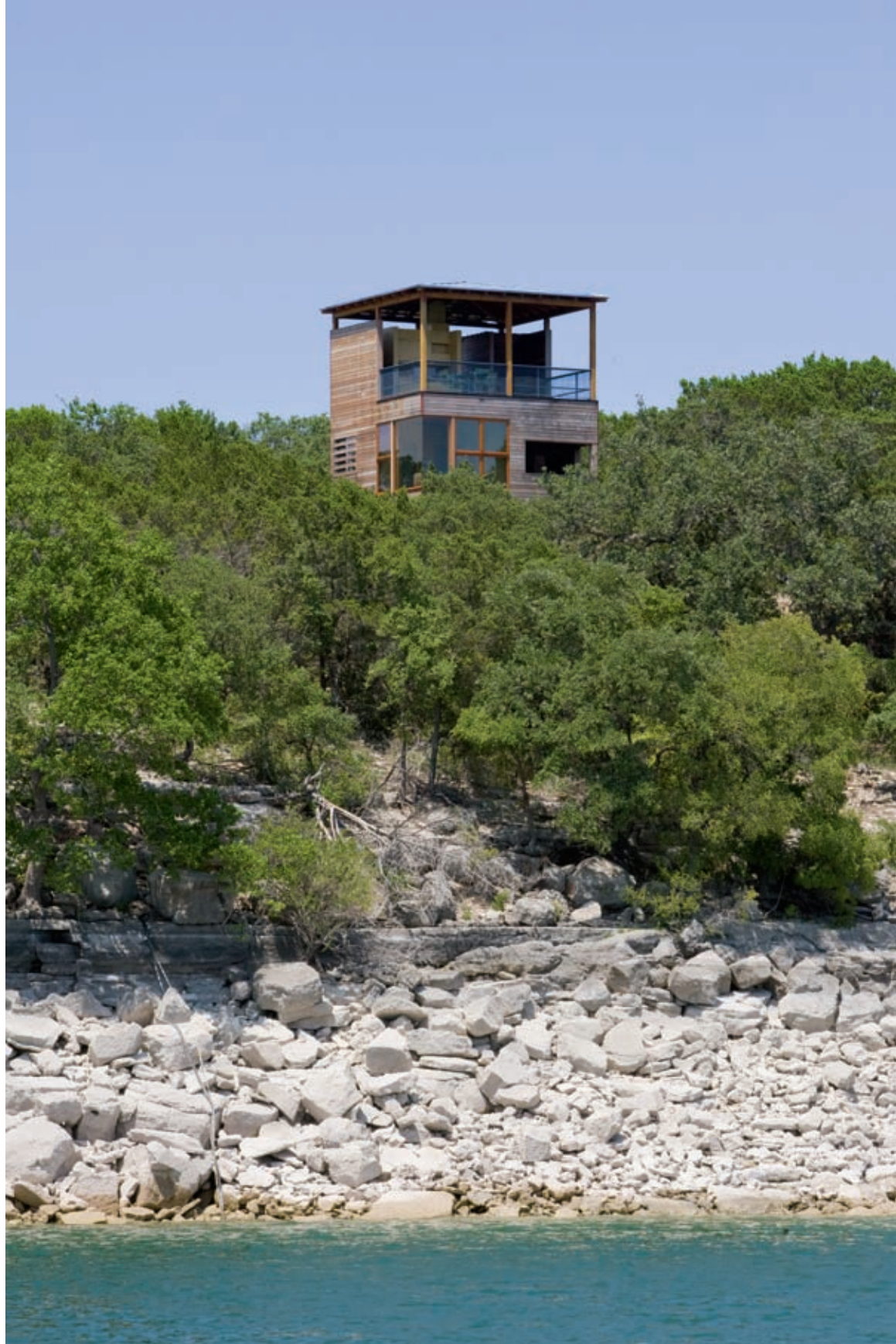
View of Tower House from Lake Travis
