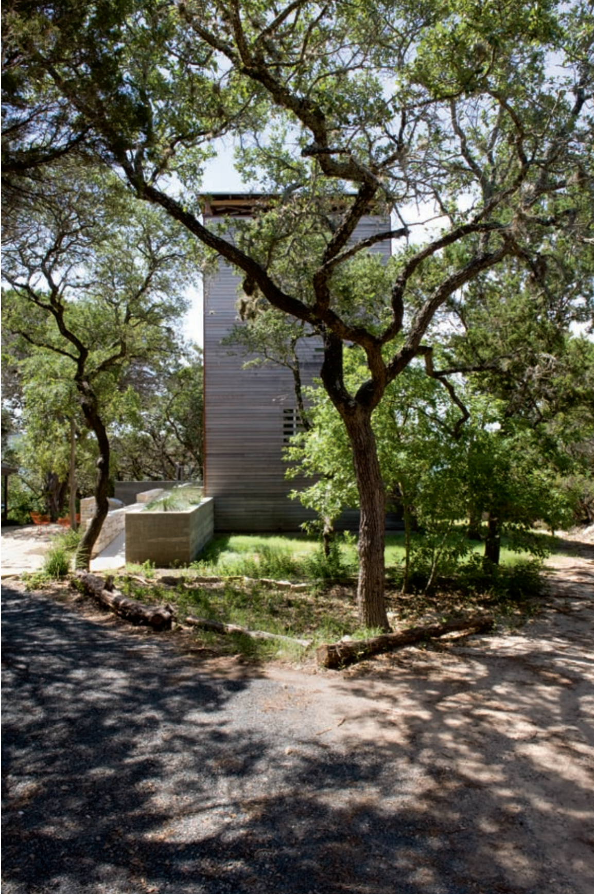
Tower House north facade
