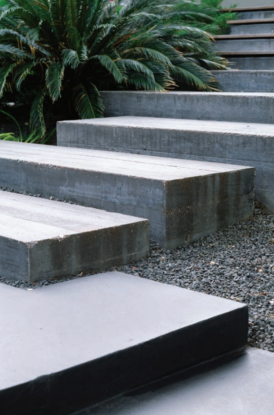
Entry stair detail
