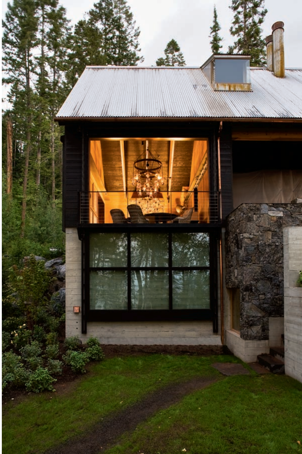
Lodge, dining room window and balcony in open position
