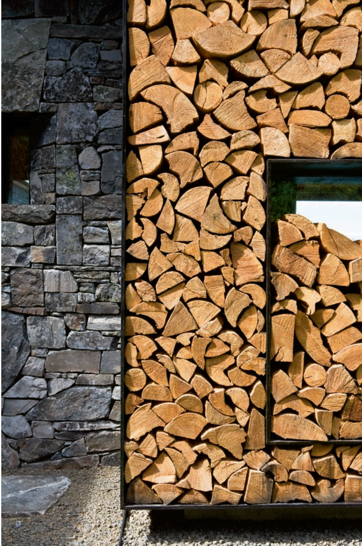
Stone and cordwood wall detail
