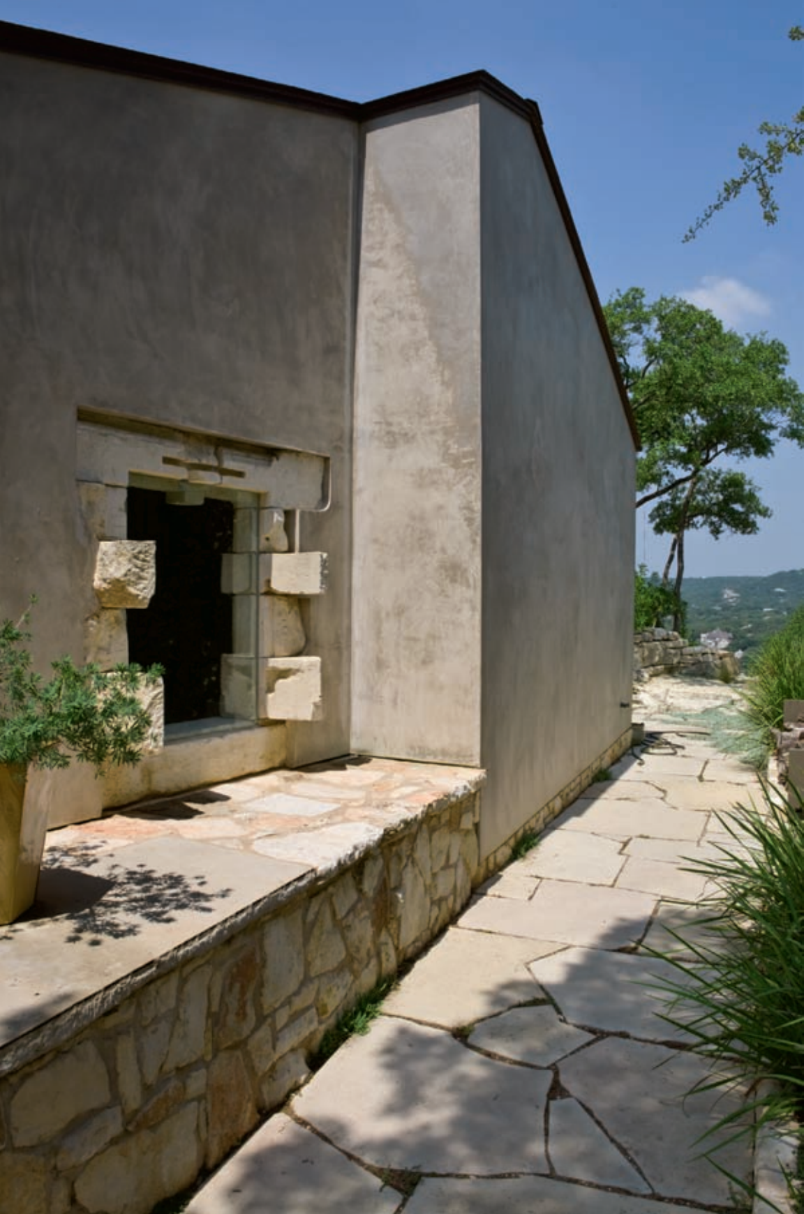
View of north facade
