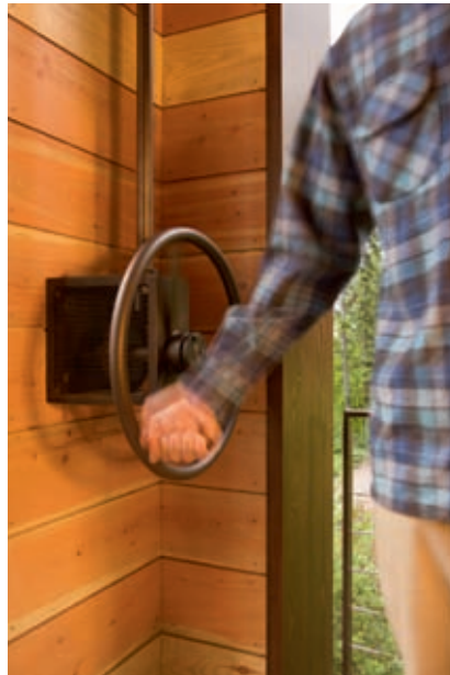
Lodge (top to bottom): Indoor outdoor dining room Crank mechanism for moveable wall
