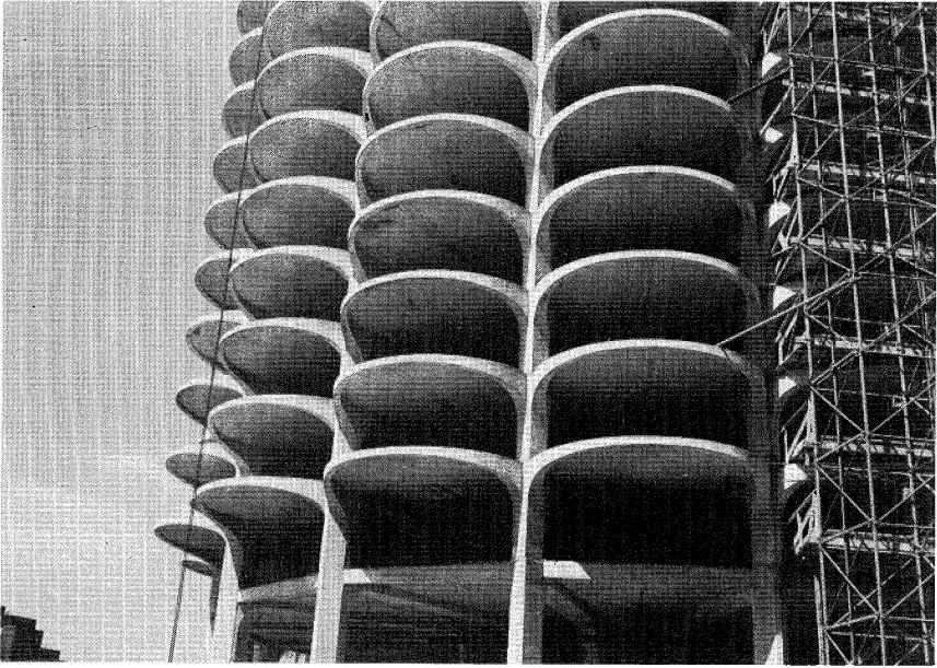
Figure 1-2. Reinforced concrete building. (Courtesy of the Portland Cement Association, Chicago, IL.)
