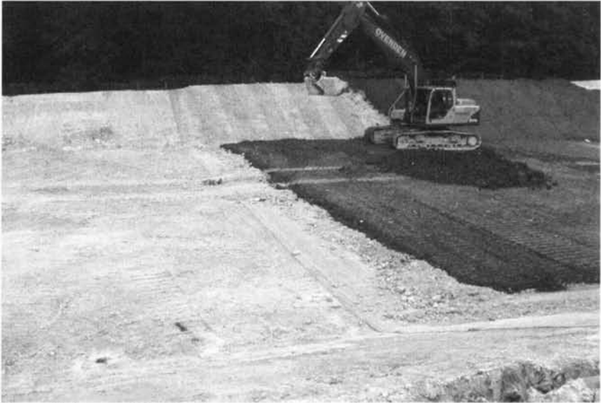
Figure 5, Laying GCL barrier in drainage run-off ponds
