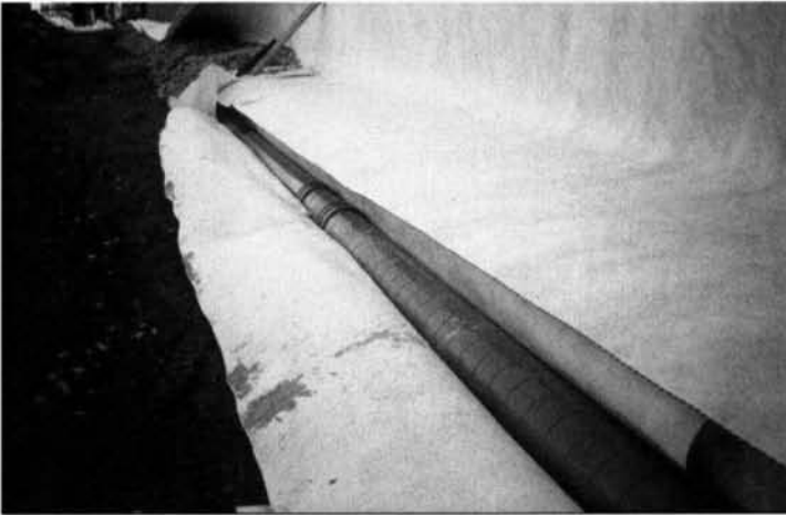
Figure 14, Perforated drain wrapped in a geo-composite drain
