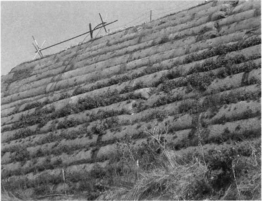
Figure 3, A2/M2 J1 to 3 -reinforced slope using geogrid
