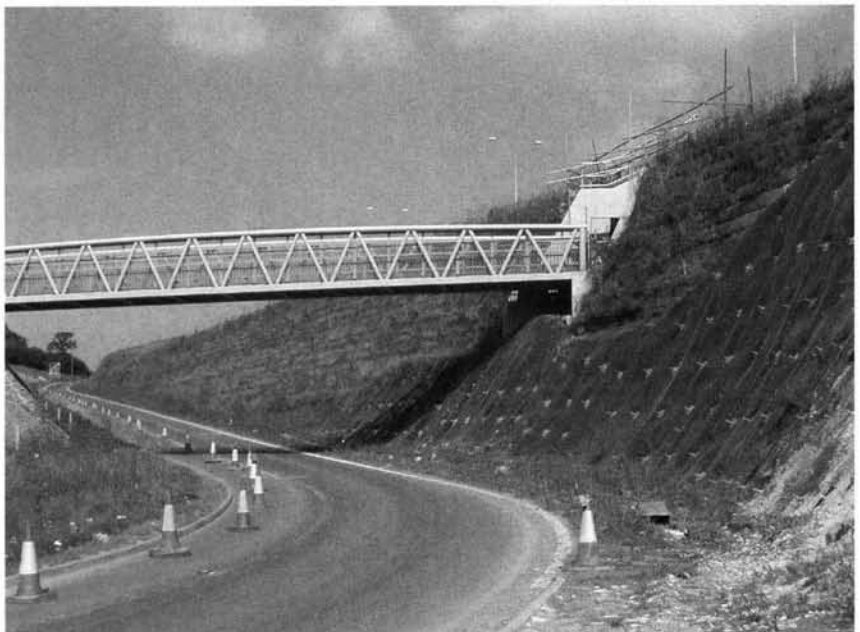
Figure 4, Soil nailing with erosion control matting
