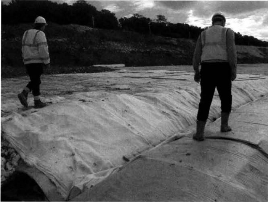
Figure 9, Multi-layer barrier/ protection/ reinforcement/ gas venting system
