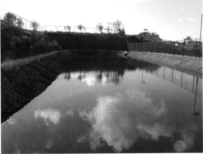
Figure 7, Pond with soil covered barrier & protection GTX
