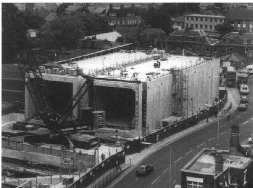
Figure 9, Vehicular tunnels, Silver Street Station, London
