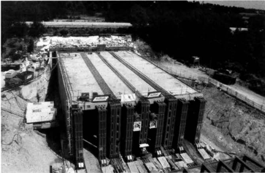
Figure 15, Culvert ready for installation, Dorney, Berkshire
