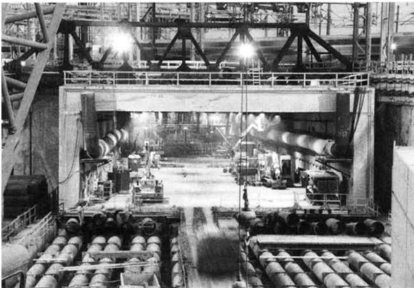
Figure 18, Rear view of I-90 Eastbound box during tunnelling, Boston
