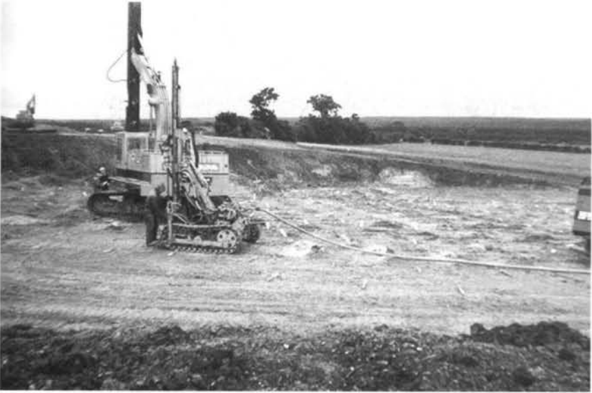
Figure 15, Installing prefabricated geosynthetic band drains
