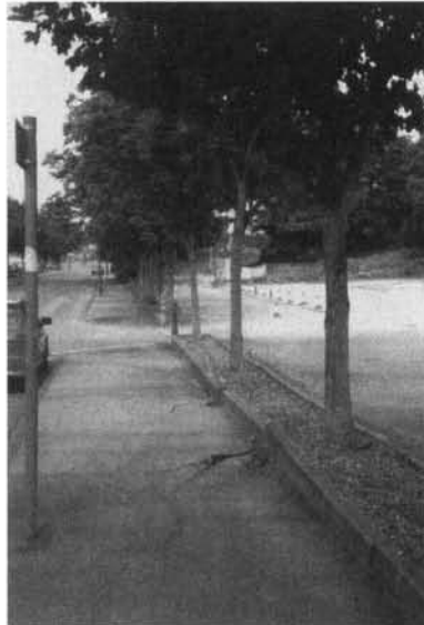
a). Damage to pavements due to tree roots, Nottingham Trent University car park
