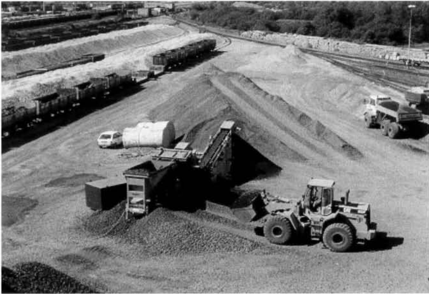
Figure 2, Recycling railway ballast
