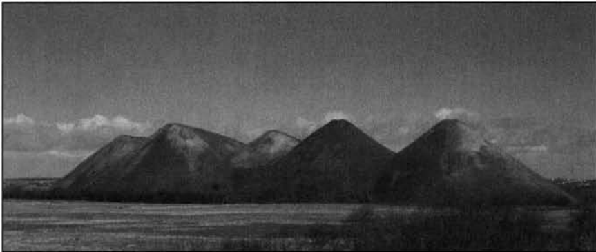
Figure 3, The Five Sisters spent oil shale West Lothian. (Recent estimates indicate that around 100,000kt of spent oil shale is stored in similar tips in the eastern central belt of Scotland)
