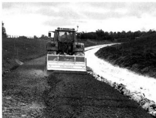
Plate 2, HBFM pulverisation and stabilisation processing
