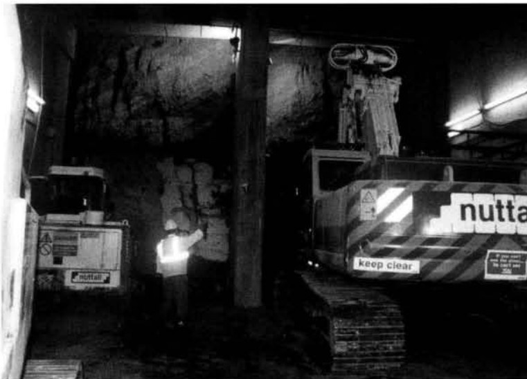
Figure 14, Excavation of frozen sands and gravels, Dorney, Berkshire
