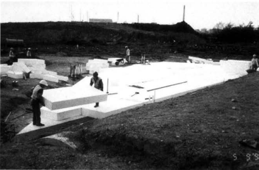
Figure 10, Laying ultra lightweight fill (EPS foam blocks)
