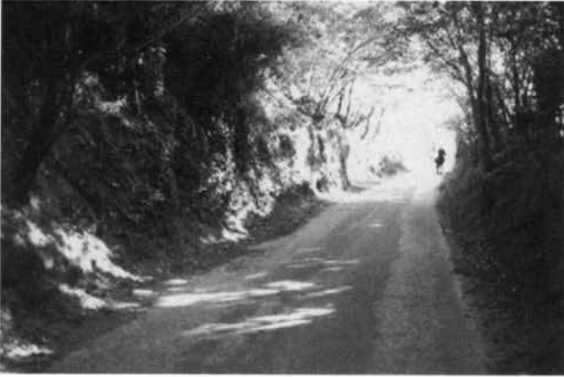
a) Water Lane, Kent. Vegetation root network permits steeper slopes in Greensands
