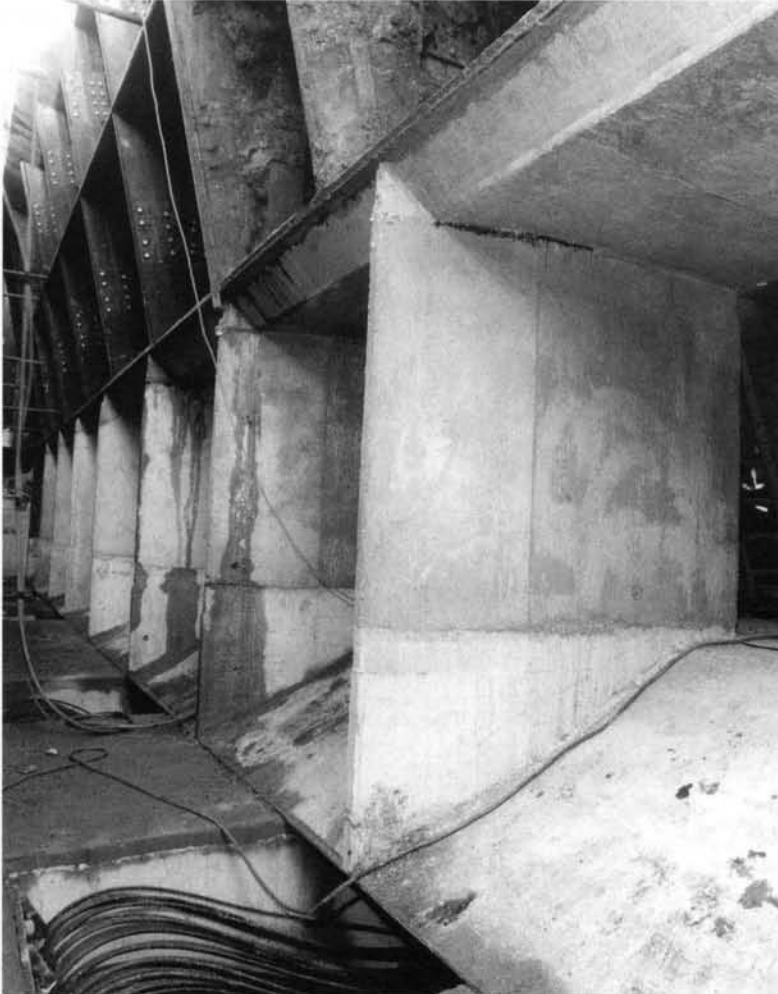
Figure 2, The composite reinforced concrete and steel shield, Lewisham Station, London
