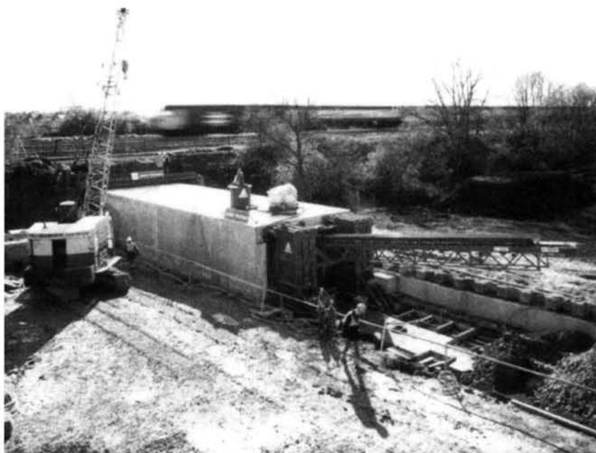
Figure 5, Pedestrian/ cyclist subway, Didcot, Oxfordshire
