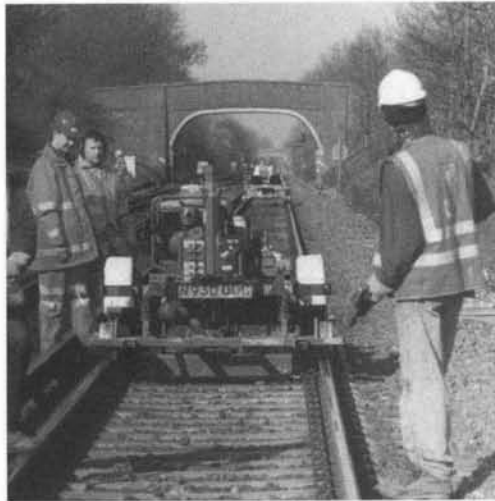
Figure 18, The Falling Weight Deflectometer in use on rail track
