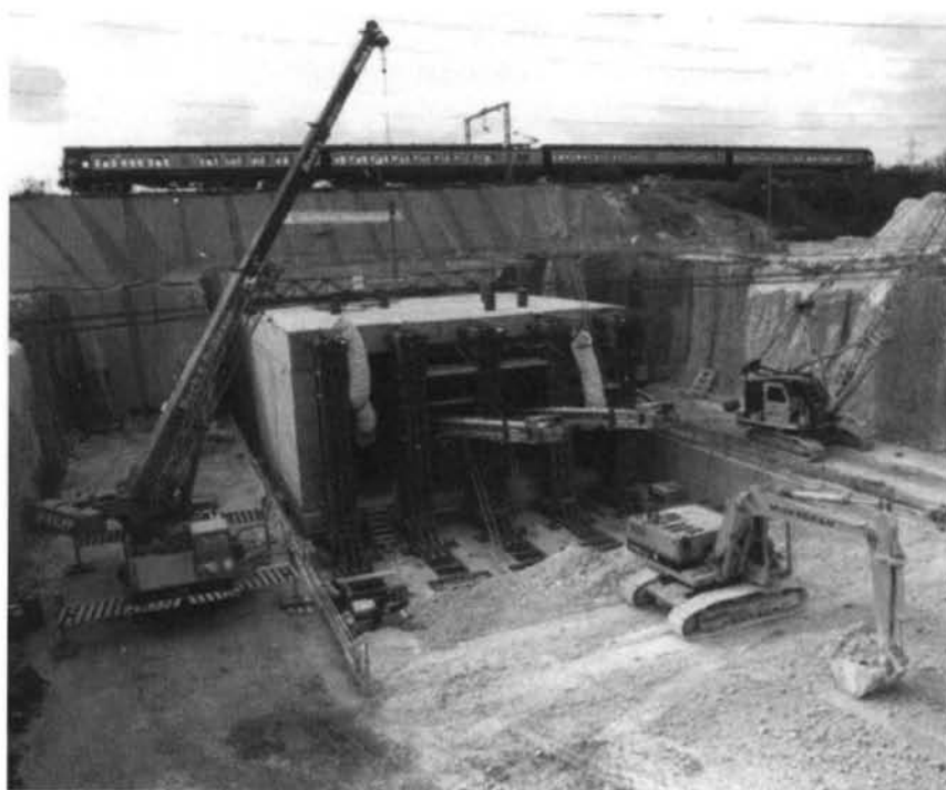
Figure 7, Vehicular underbridge, West Thurrock, Essex
