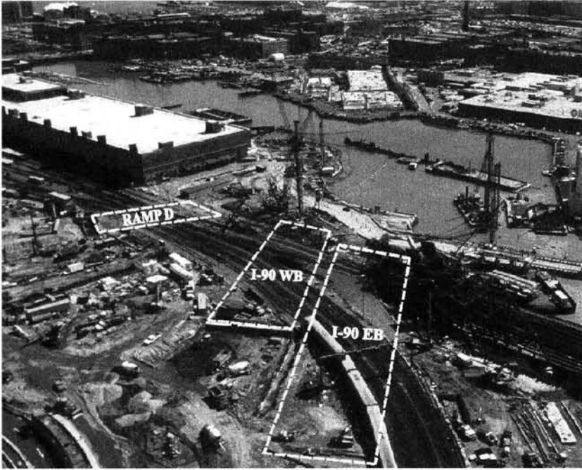
Figure 17, Boston site, showing the position of the three jacked box tunnels
