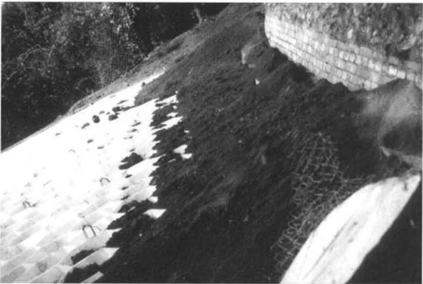
Figure 16, Geotextile erosion control system
