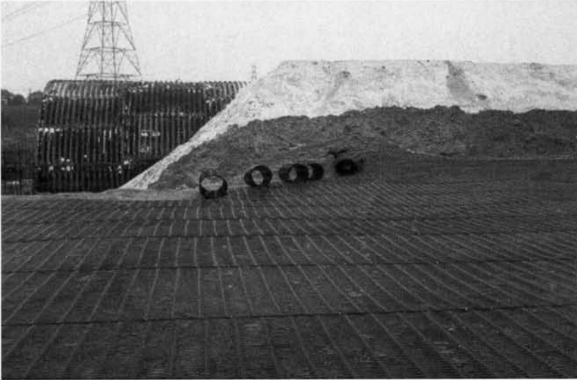
Figure 11, Geogrid basal reinforcement at base of embankment
