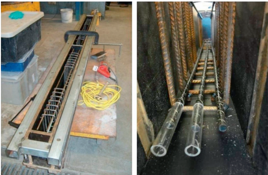
Figure 14.3 Wood mold and reinforcement cage for test beams.
