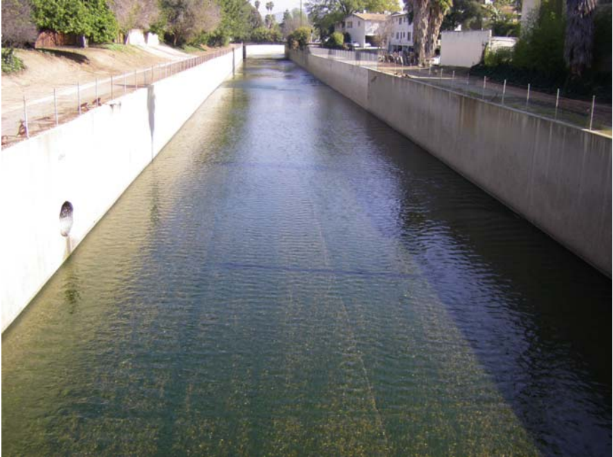
Fig. 6.2 View of a non-alluvial channel, whose boundaries cannot be modified under the current discharge regime (Los Angeles River, California)
