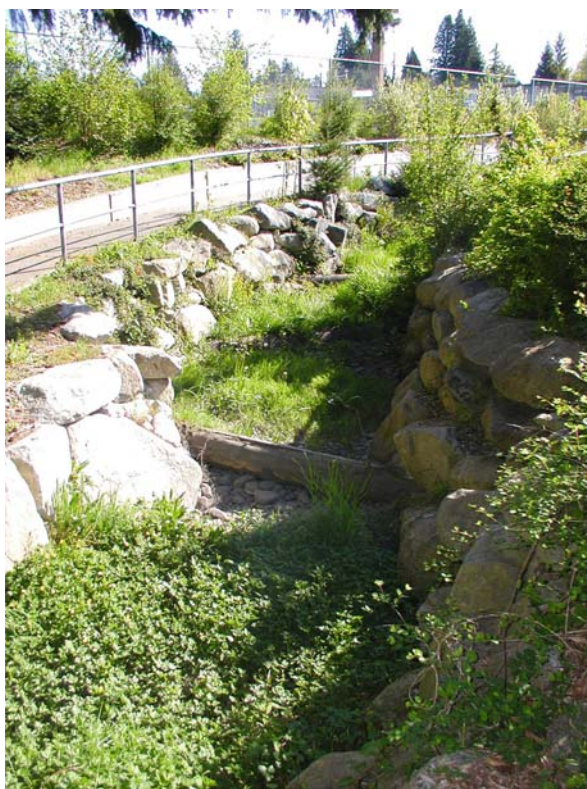
Fig. 8.5 Viewlands Cascade, Seattle's first natural drainage project. This vegetated swale receives runoff from approximately 26 acres of urban land, reducing the total runoff volume that enters a salmon stream below this location. Photo by K. Hill
