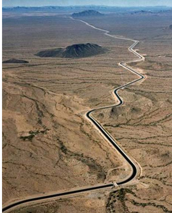
Fig. 4.5 Typical concrete canal in the western USA delivering water from distant reservoirs and rivers to urban regions in the desert
