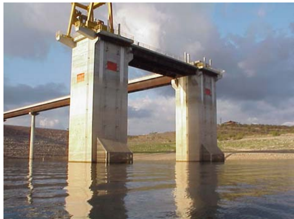
Fig. 4.3 Photographs of a typical outlet structure located in a reservoir (Lake Pleasant, Arizona)
