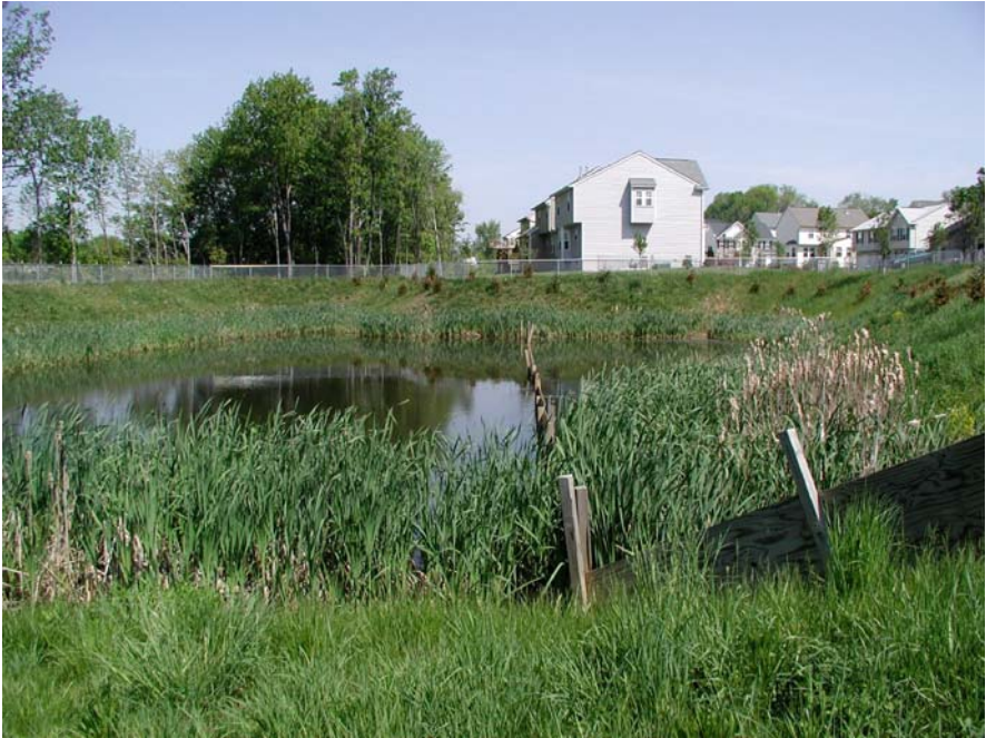
Fig. 2.5 Stormwater detention basin in suburban Baltimore, MD. Photo by Claire Welty
