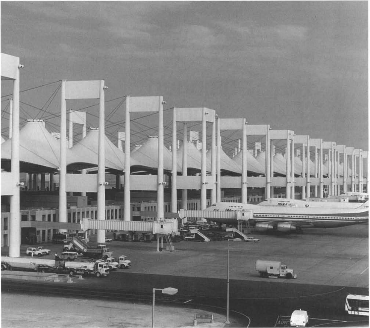
The Hajj Terminal at Jeddah International Airport in Saudi Arabia is the world's largest tensioned fabric roof.
