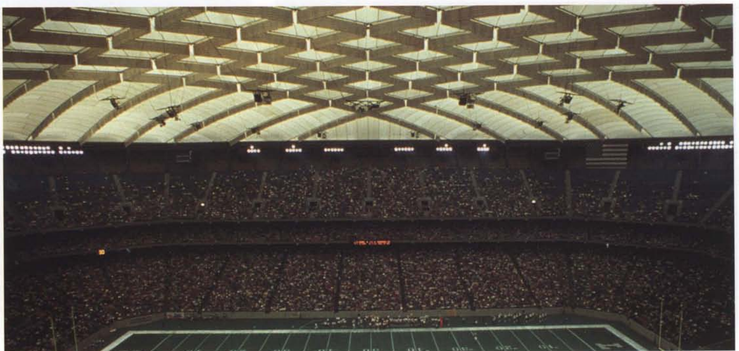
PLATE 18 THE TENSIONED FABRIC ROOF
