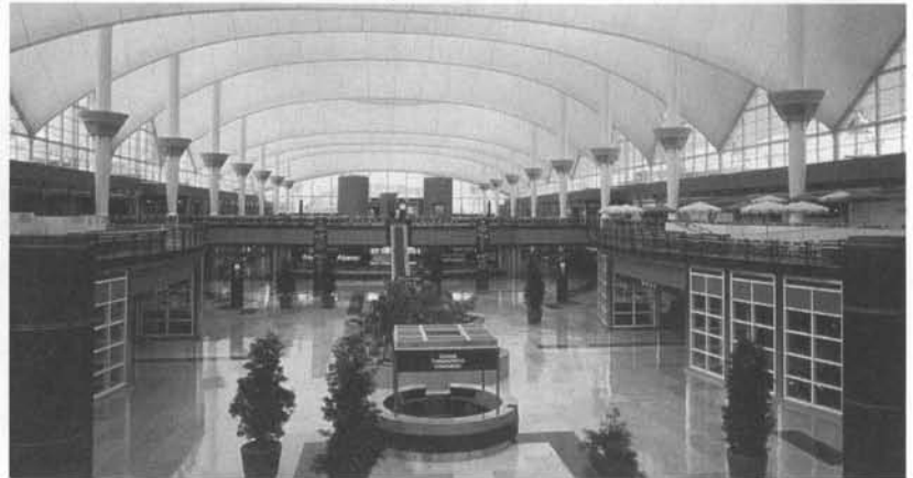
[ABOVE] The repeated ridge and valley modules of the enormous Denver Airport roof provide its classic sawtooth form.
