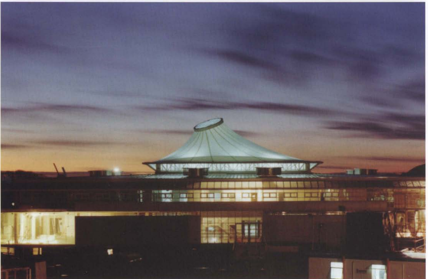
PLATE 6 THE TENSIONED FABRIC ROOF
