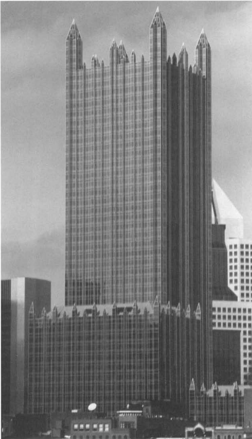
The Pittsburgh Plate Glass office tower is a monument to the potential of glazed fascia that offers no hint of the structure that supports it.
