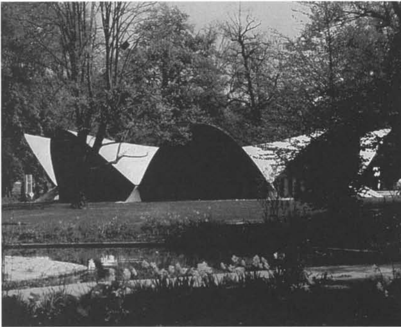
[LEFT] Jörg Schlaich's Stuttgart Garden Fair roof achieves a structurally expressive form with a glass fiber-reinforced concrete shell of only 10-mm thickness.
