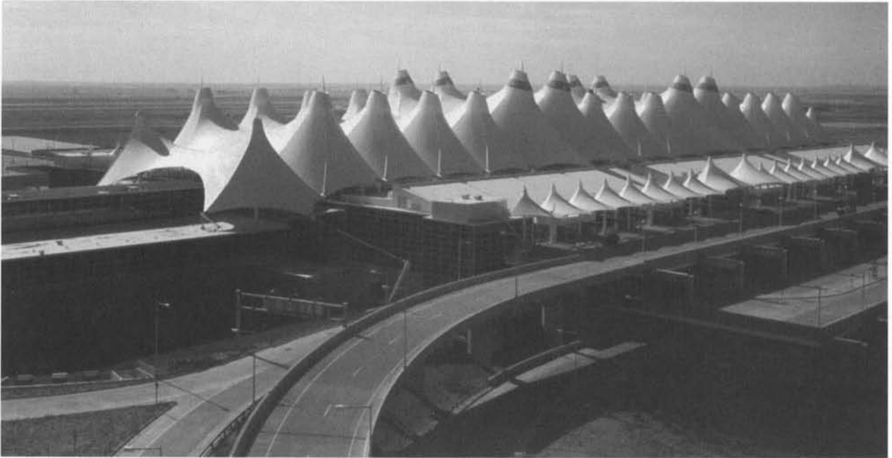
[ABOVE] The repeated ridge and valley modules of the enormous Denver Airport roof provide its classic sawtooth form.
