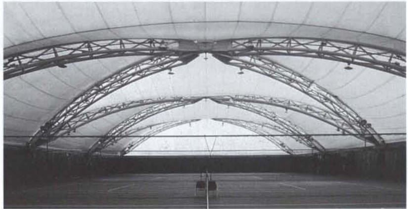
(RIGHT) The crossed arches used at the Pizzitola Athletic Facility eliminate the need for lateral bracing.
