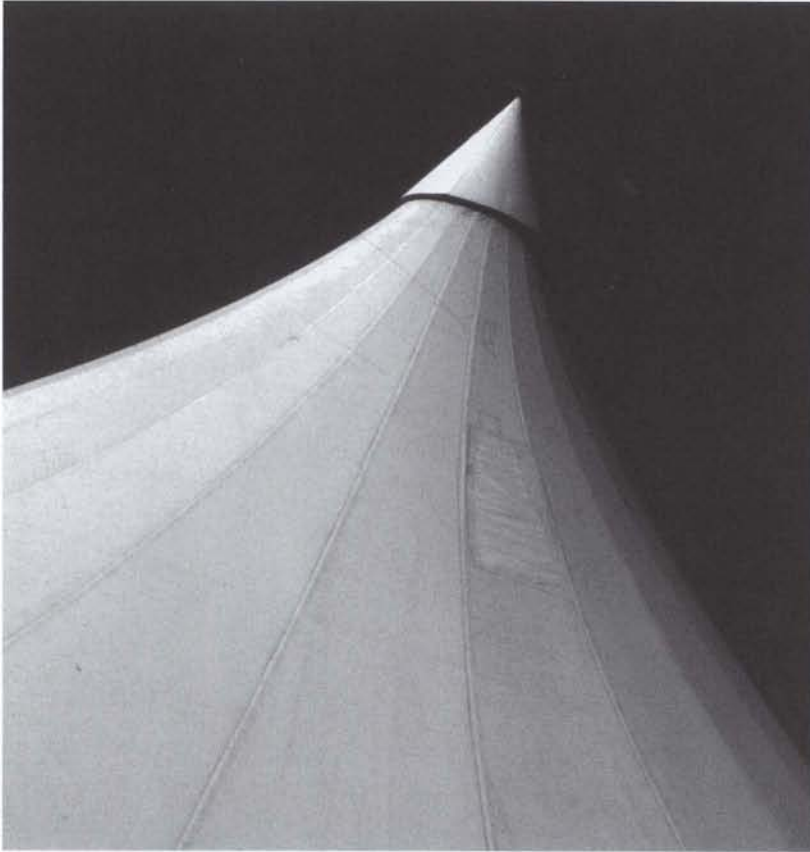
The mast peak baffle used at the University of La Verne mirrors the fabric itself in shape and color.
