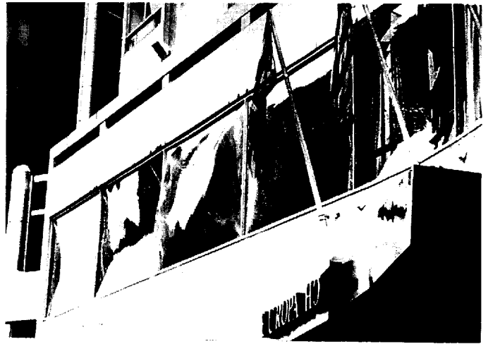
Fig 11. Europa Hotel, Belfast - laminated glass remaining intact
