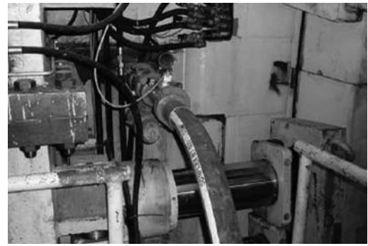
Figure 22. Grout port at axis of TBM.
