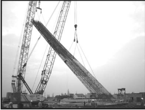
Figure 5. Lifting of reinforcement cage.
