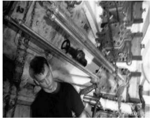
Figure 11. Demonstration for changing cutters in the centre of cutter head.
