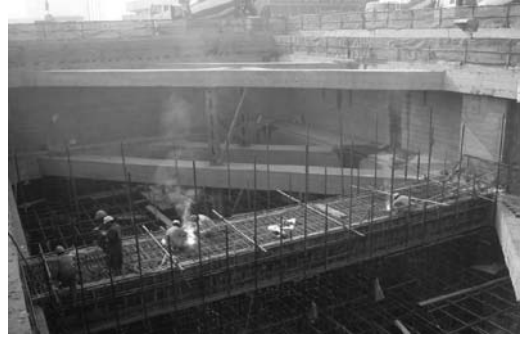
Figure 4. Xiangyin Road Tunnel – inner structure construction.
