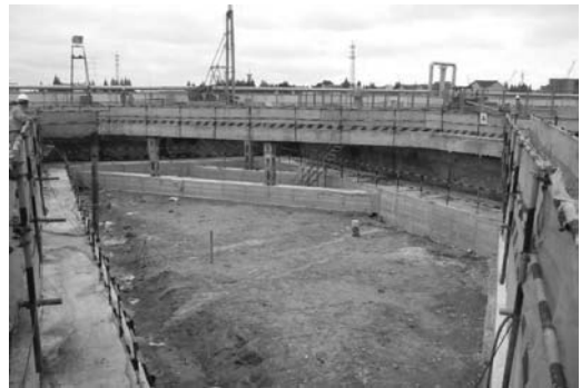
Figure 5. Changjiang Tunnel – Enclosure structure construction.
