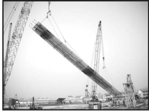
Figure 3. Lifting of GFRP reinforcement cage.
