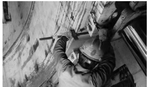
Figure 24. Measuring ‘tailskin gaps’.
