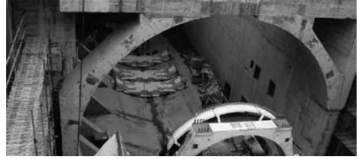
Figure 7. Concrete reaction structure.
