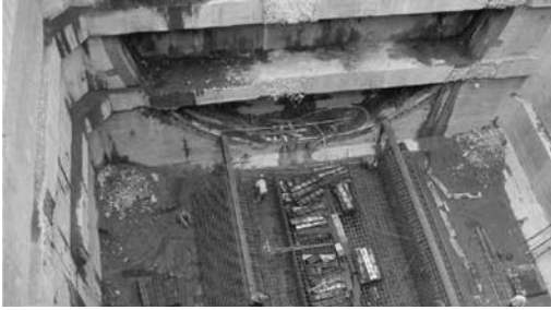
Figure 6. Cradles for launching.
