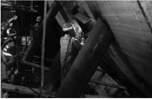
Figure 10. Propping 'shove' rings in shaft.
