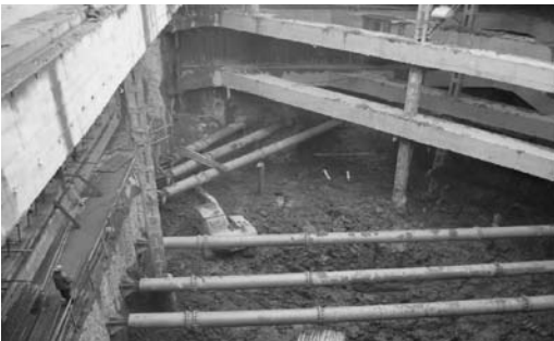
Figure 3. Fuxing (E) Tunnel – Foundation pit excavation.
