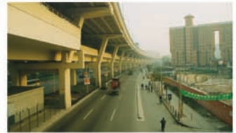
Honghexin Road Elevated Project the first project combining ground road, rail transit and viaduct in China
