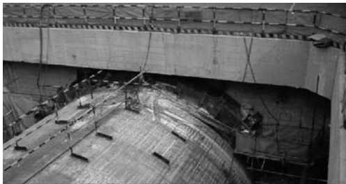
Figure 11. Installing extra supports at the steel launch seal.
