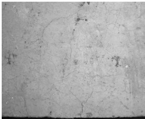
Figure 7. Spalling and cracks of the specimen without polypropylene fiber.
