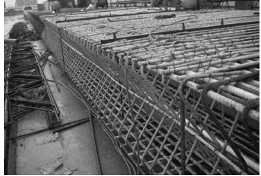
Figure 17. GFRP bars binding site.
