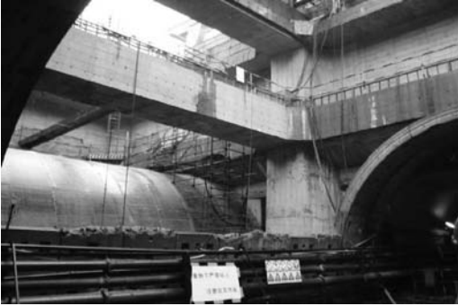
Figure 2. Dalian Road Tunnel – Shield launching.
