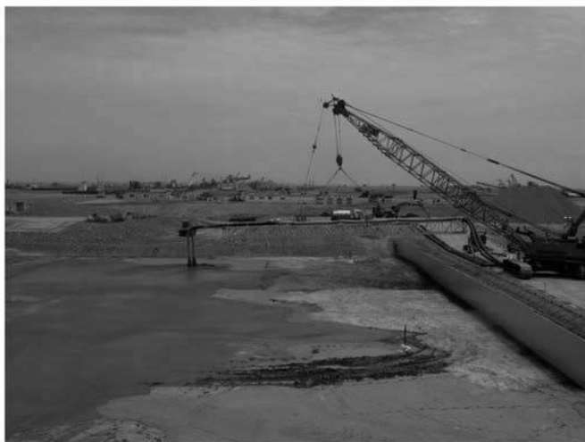
(b) Placement of stabilized soil for land reclamation.
