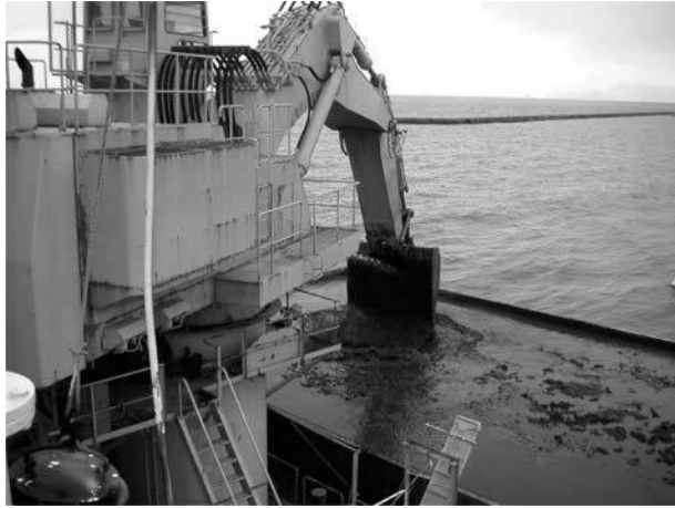
Figure 5.12 Remolding dredged soil in the transportation barge.
