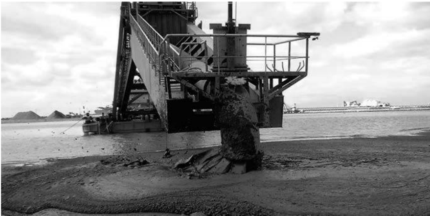
Figure 4.14 Placement of cement-stabilized soil in Tokyo/Haneda International Airport construction.
