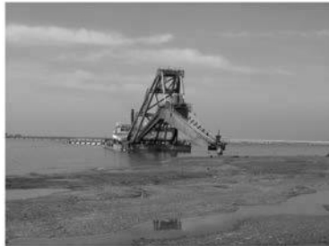
(b) Placement barge.
