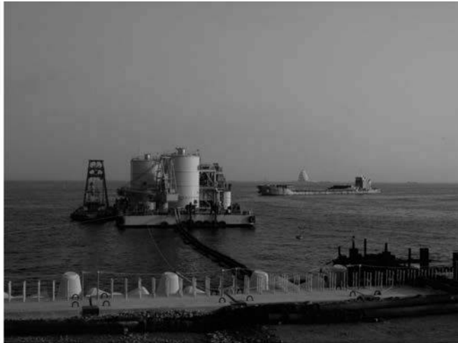
(a) Special barges for marine works.
