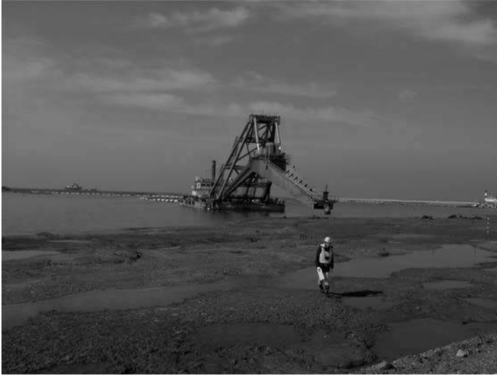
Figure 1.9 Pneumatic flow mixing method at the Central Japan International Airport construction project.
