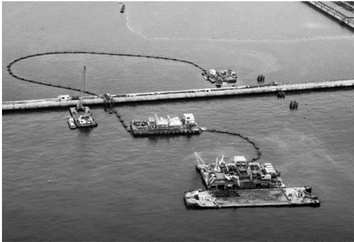
Figure 1.8 Barges for the pneumatic flow mixing method.
