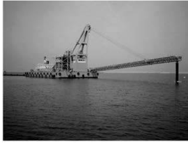
(a) Pumping type placement barge.
