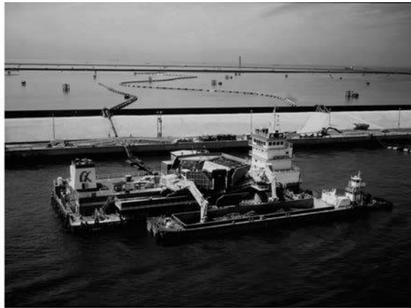
(a) Soil transfer barge.
