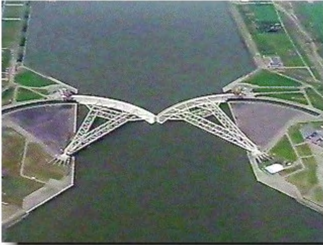
Fig. 1. Top view of the Maeslant Kering near Hoek van Holland. At the top of the figure the Nieuwe Waterweg flows to the North Sea; in the bottom direction is Rotterdam. The Nieuwe Waterweg is about 300m wide.
