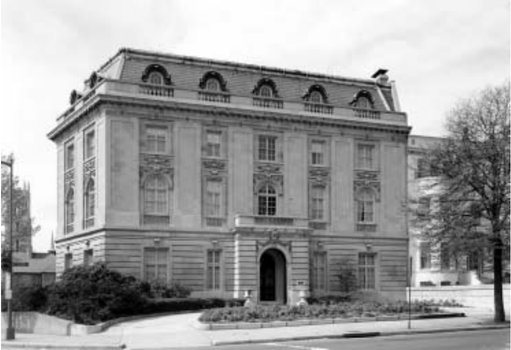
FIG. 20. Alexander Stewart House, 2200 Massachusetts Ave., NW, designed by Jules-Henri de Sibour, built 1908–9. Photograph by Jack E. Boucher, Historic American Buildings Survey, 1970. (Courtesy Library of Congress.)
