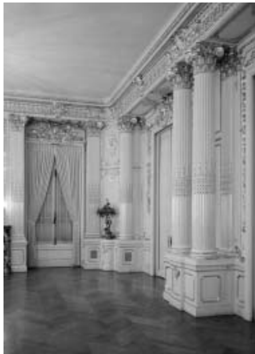
FIG. 23. Pullman House interior, northeast corner of the first-floor salon. (Courtesy Library of Congress.)
