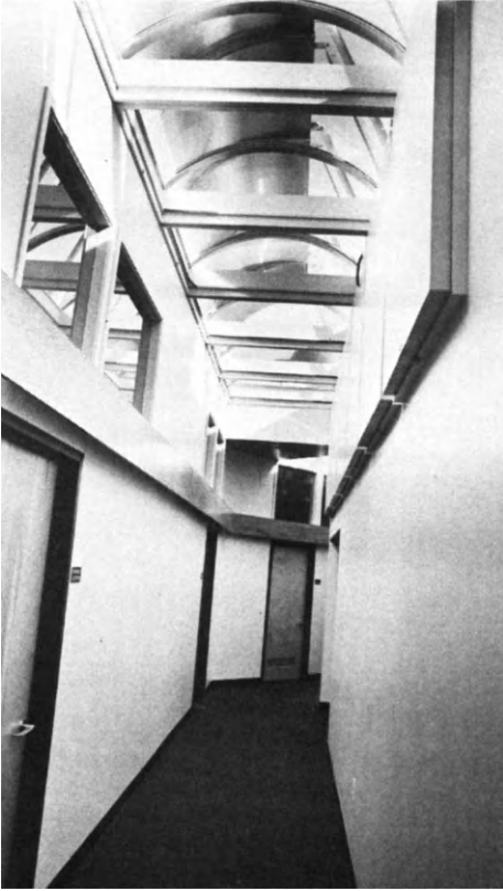
Illustration 3. Hallway with Reflectors and Moveable Insulation
