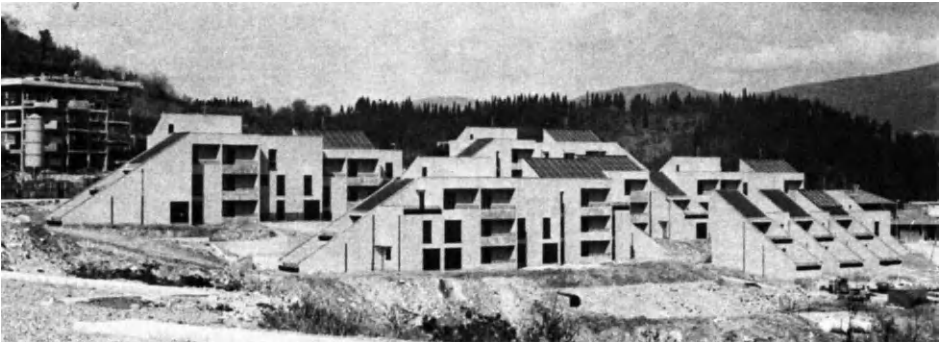
Fig. 1 - General view from South-West
