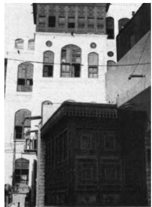
Fig. 18. Old Nasif House in the background & new Rushaan work in the foreground used as an office. Note the glass panels behind the new Rushaan
