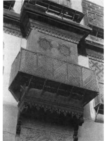
Fig. 3. Typical Rushaan with the wooden screen surrounding the openings for privacy.
