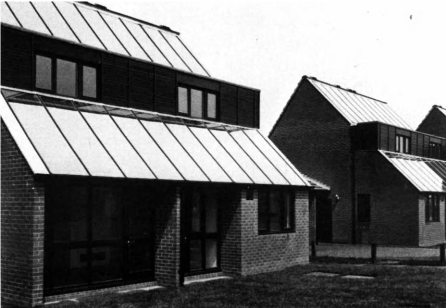
Linford Houses (John Laing Contractor)
