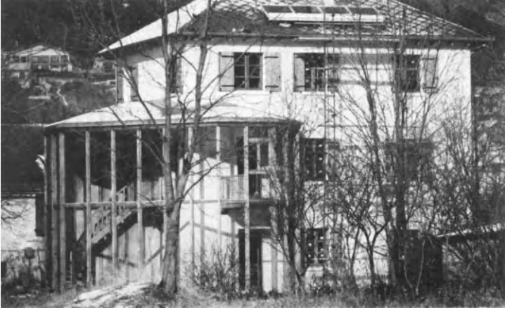
Fig. 2. Maison du Lac. View from South.
