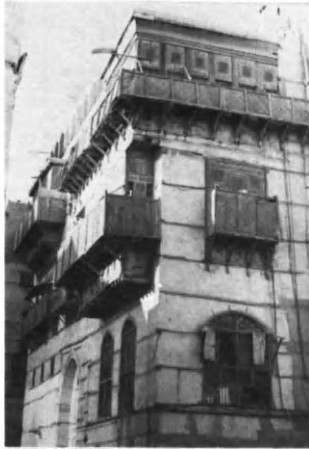
Fig.16. Typical simple window and Cantilevering Rushaan & A Mabit on the top
