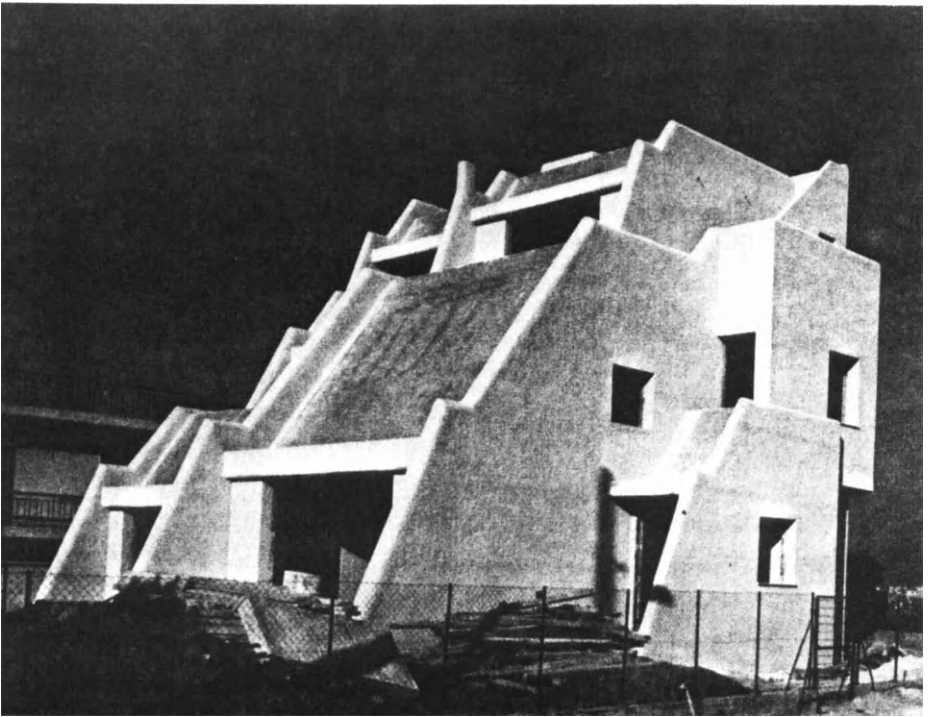
Fig. 3. Initial sketch and actual construction state.
