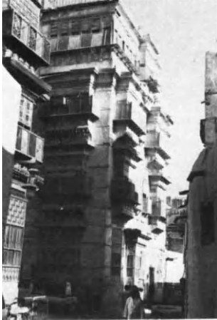
Fig.15. Rushaan on the ground floor did not have screens around them as this floor is to be used by men.
