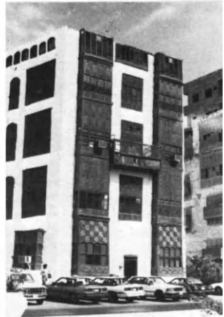
Fig.17. Rawashin were either connected vertically or horizontally for decorative purposes
