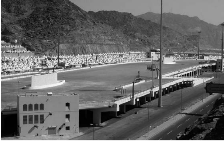
Fig. 21: Safety tuning: The first Jamarat Bridge after renovation in 2004.
