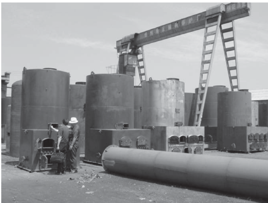
Plate 6.1 Yang Wenzhu's 'Xinzhou Welfare Boiler Plant of Shanxi Province' located in the centre of Yuanping City
