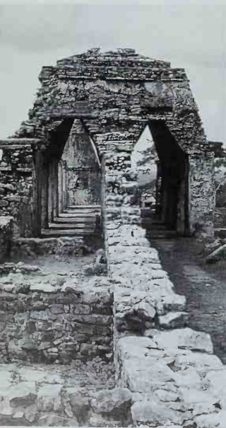
25. Palenque architects both stabilized and enhanced the corbel vault by setting the heavy roofcomb along the central load-bearing wall, possible in the parallel corbel constructions of the Palace.
