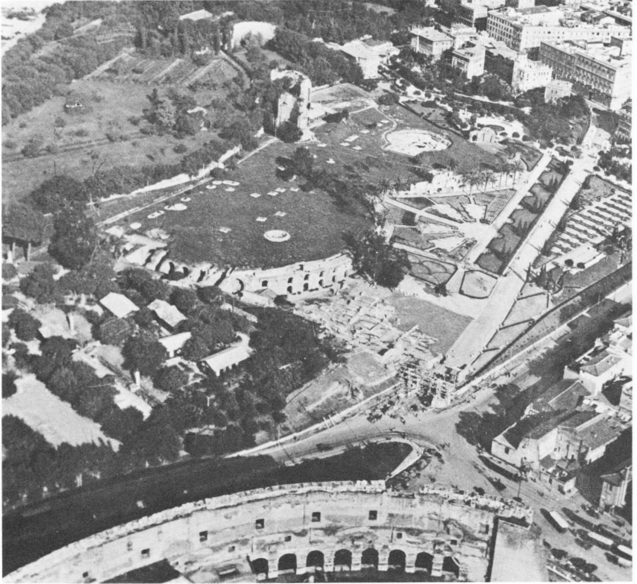
22. The Baths of Trajan and the site of the Domus Aurea Esquiline wing from the air
