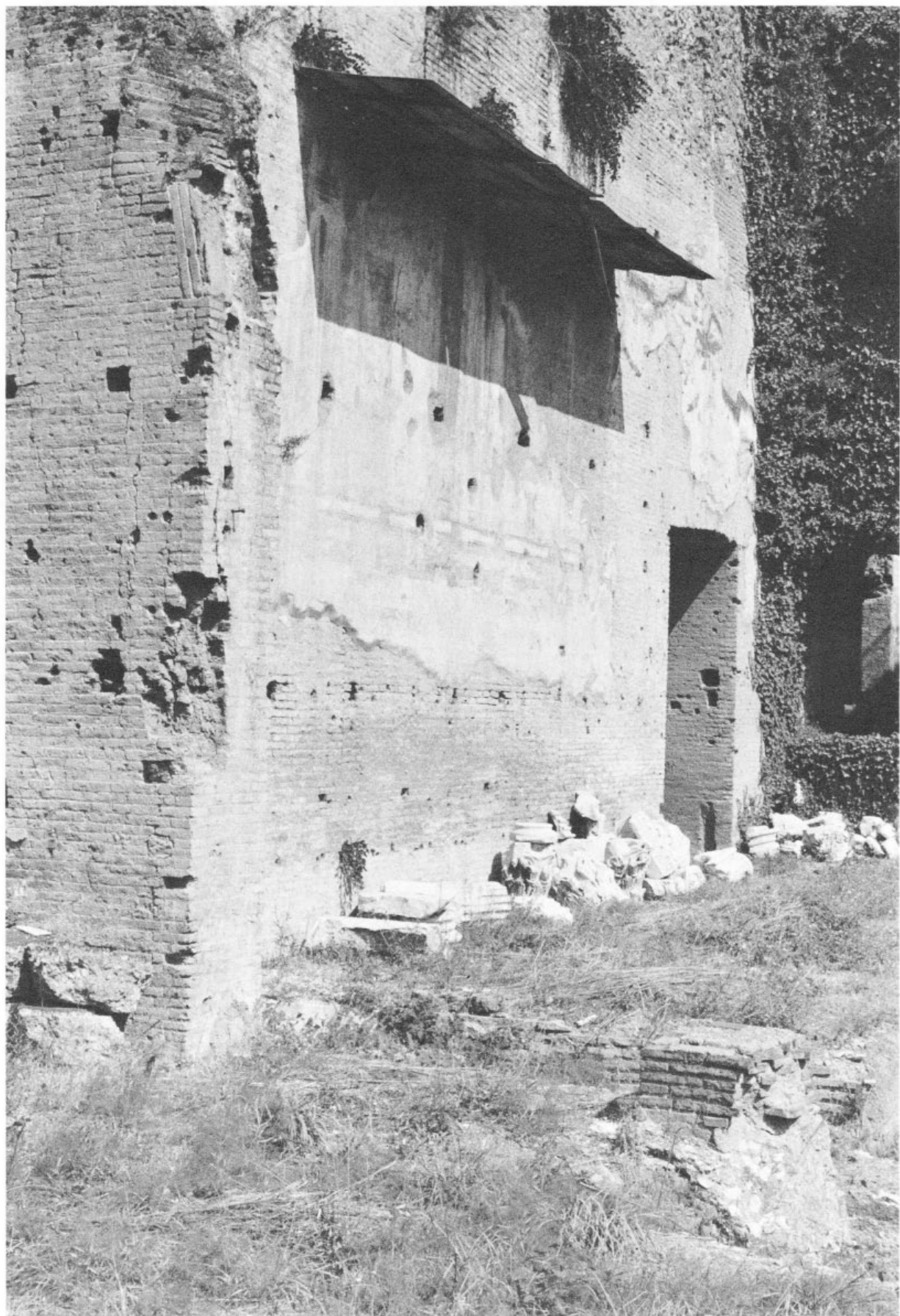
63. The Domus Augustana, the northeast wall of room 8 on Plate 58 and the remains of its pier and doorway arch
