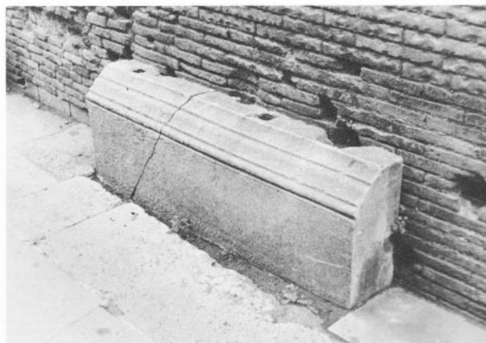
120b. Another level I exterior base molding block
