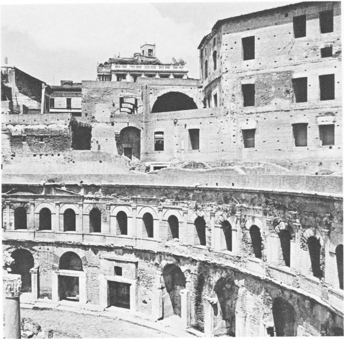
82. Trajan's Markets, sections A2, B1, and part of B2, from the south
