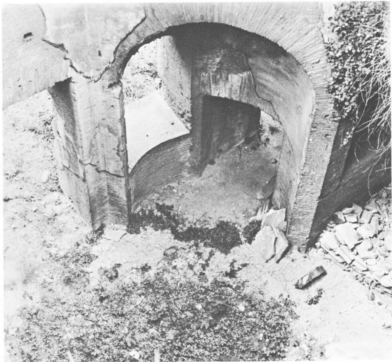
59. The Domus Augustana, looking into one of the octagonal rooms (number 5 on Plate 58) from the east
