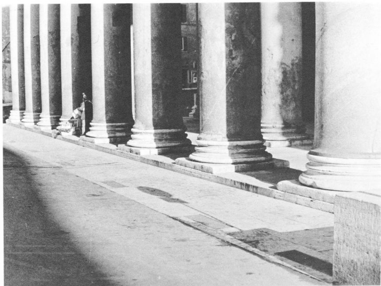
97. The Pantheon, portico column bases and the modern paving over the original steps
