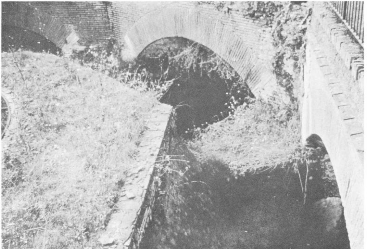
33b. Detail of the superstructure
