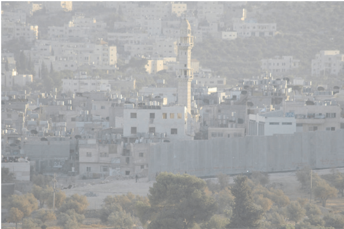
Figure 66.2: The Security Fence Separating Israel and the West Bank. Photo © Gershon Baskin. Publication permission was granted.
