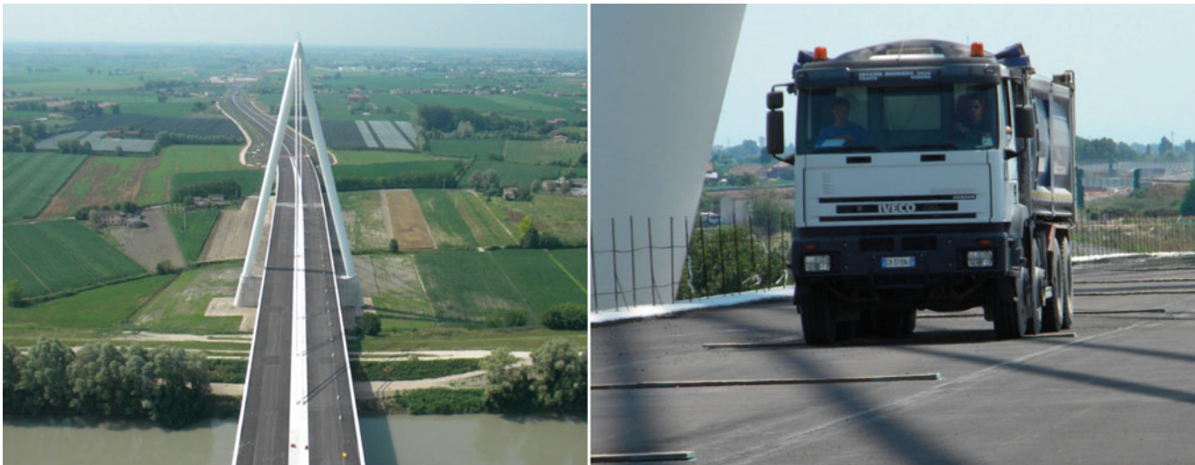
Fig. 17.2 Aerial view on the bridge and truck passing on the obstacles on the deck
