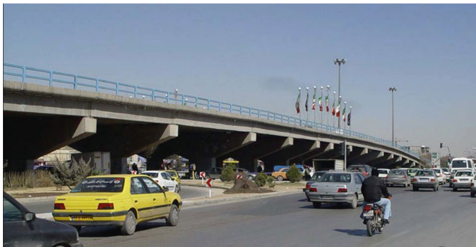
Fig. 18.2 Bridge elevation and vehicle traffic below
