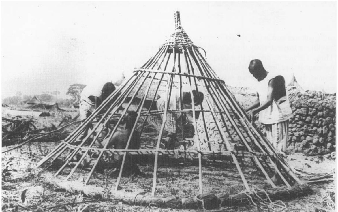
Building the conical roof for a dwelling in Nigeria
