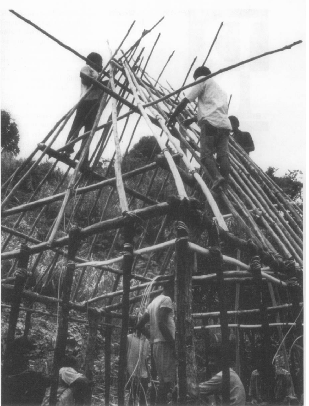
Building a house in Fiji
