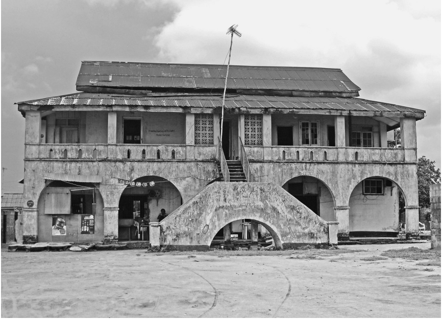
Figure 5.4 Decaying former District Officer's residence
