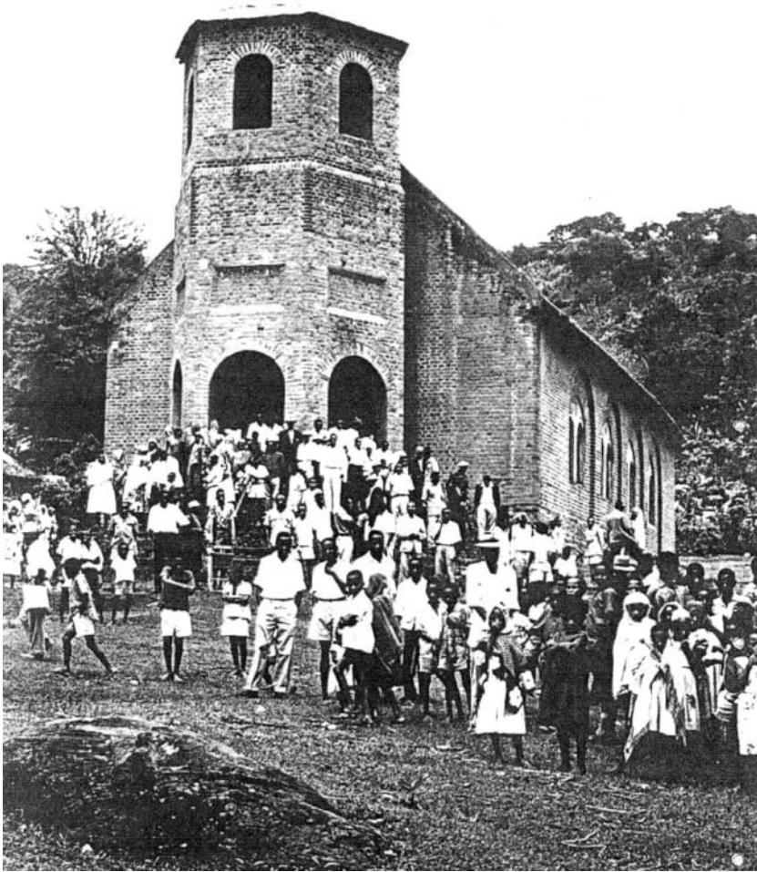
Figure 12. Mamba-Myamba Church Building 7
