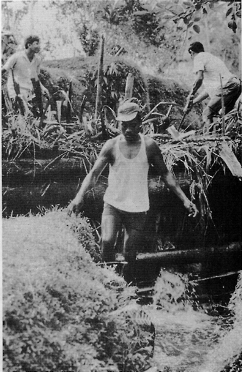
11. Reconstruction in progress on the weir at Mundak Bolo
