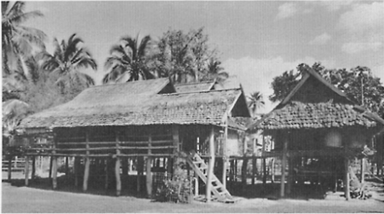
12. Village house in northern Thailand (1969). House of a small landowning farmer's family. Main house entrance is aligned North-South; granary (on right) situated to the South. Note the kalae on the roofs
