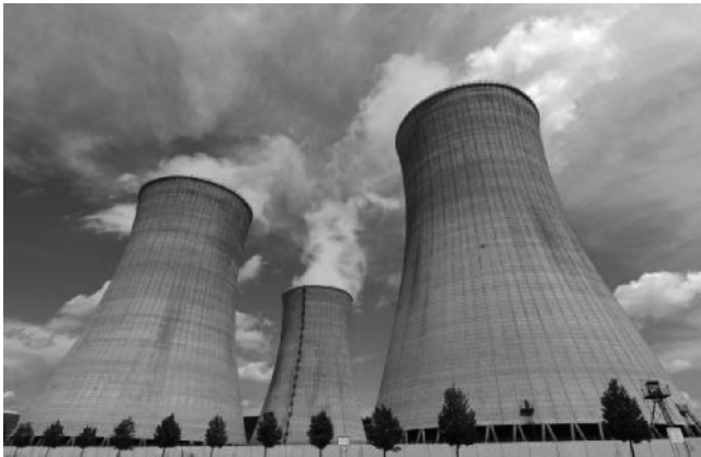
Figure 1.1 An aging nuclear power plant.
