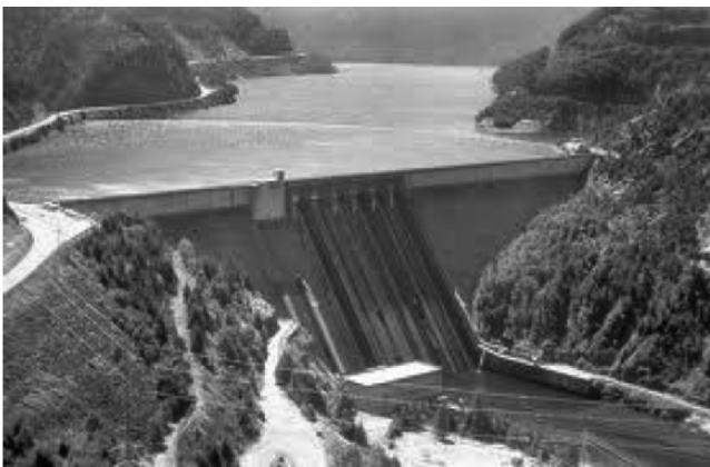
Figure 5.2 One of the 80,000 dams in the United States. Dams have important economic benefits as well as environmental issues. (Courtesy images.google.com.)
