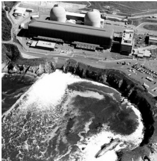
Figure 1.4 Diablo Canyon nuclear power station.
