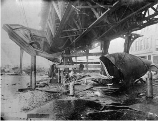
Figure 5.15 The flood damaged Boston's elevated railway.
