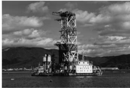
(c) Wet mixing method for marine works.
