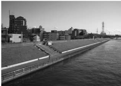
(c) River embankment at the Naka River.
