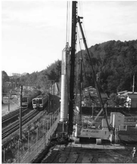
Figure 5.25 CDM-LODIC machine (by the courtesy of Cement Deep Mixing Method Association).
