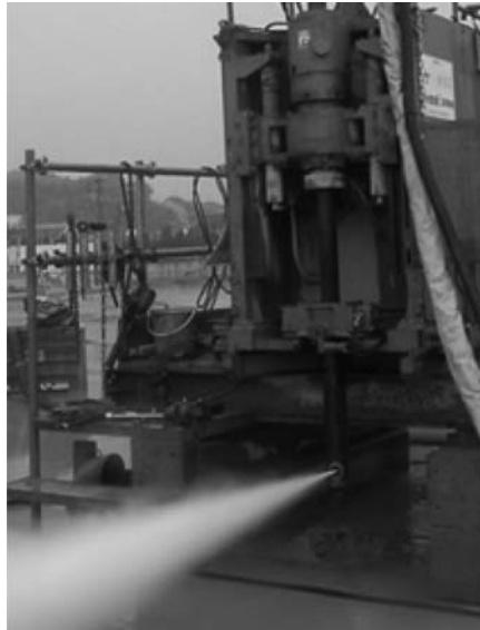
Figure 1.10 High pressure injection ( http://www.kajima.co.jp/news/digest/jul_2010/searching/index ).
