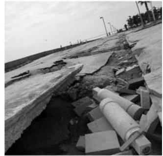
(c) Road without improvement.
