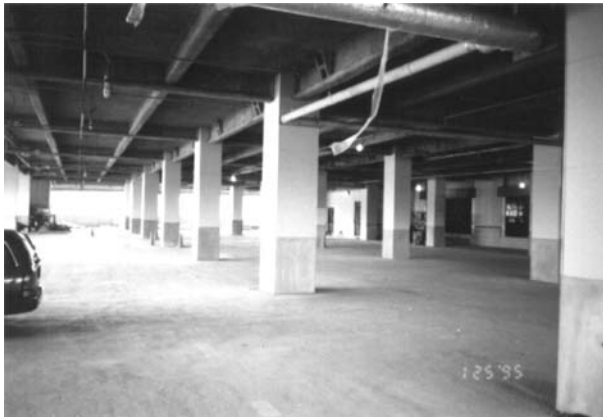
Figure 4.18(d) Parking area in the building.
