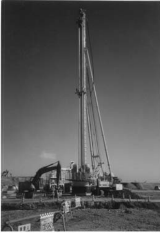
(a) Dry mixing method for on-land works.
