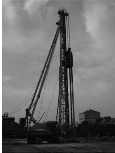
Figure 5.16 Typical CDM machine for on-land work in operation.
