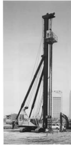
(b) Wet mixing method for on-land works.
