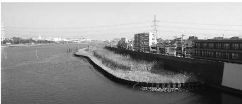
(b) River embankment after earthquake.
