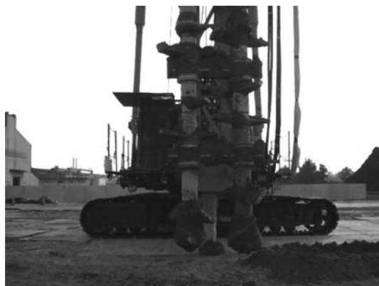
Figure 5.22 CDM machine in operation.
