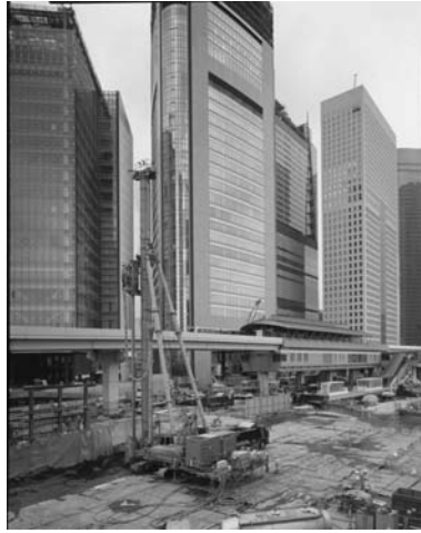
Figure 5.68 JACSMAN machine in operation (by courtesy of Fudo Tetra Corporation).
