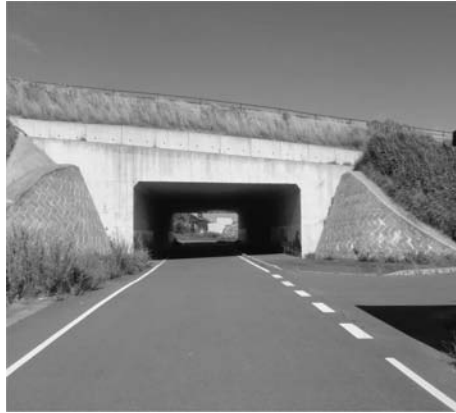
Figure 4.26 DJM improved ground for the box culvert in Chiba Prefecture.
