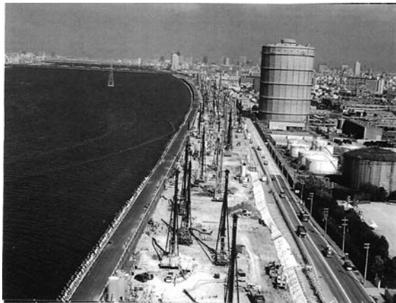
Figure 4.15(d) Deep mixing machines in operation.
