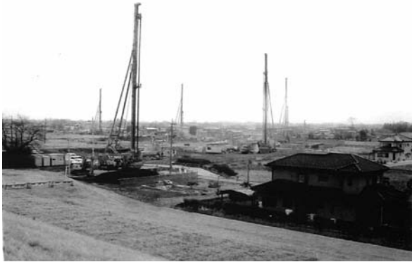
Figure 4.14(c) DJM machines in operation.
