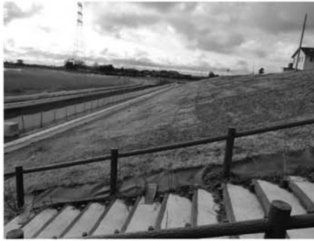
(b) River embankment at the Oshitsuke Nitta River.
