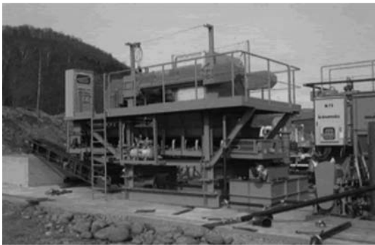
(a) High pressure compressor.
