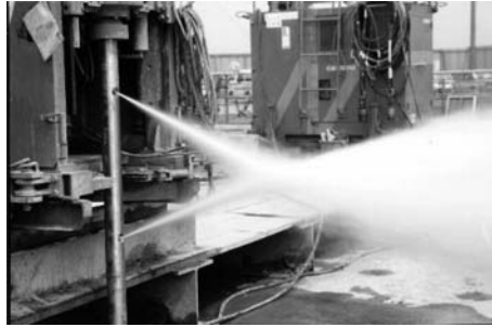
Figure 5.65 Injection of water jets from tip of X-jet method (X-jet Association, 2011).
