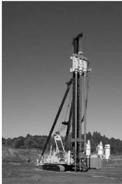
Figure 5.32 CDM-Lemni 2/3 machine (by the courtesy of Cement Deep Mixing Method Association).
