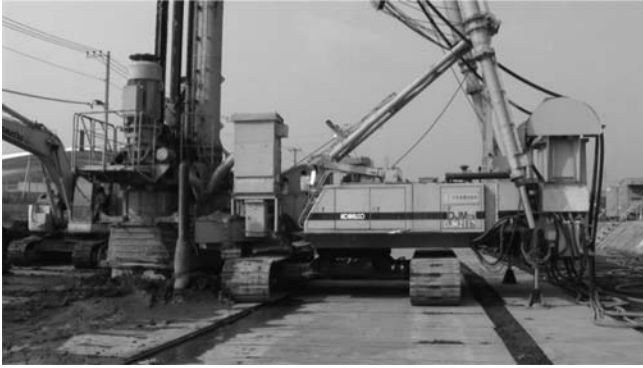
Figure 5.11 DJM machine in operation.
