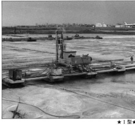
Figure 1.7 Floating type stabilization machine ( http://www.chemico.co.jp/02improvement/category01/pdf/mr001.pdf ).
