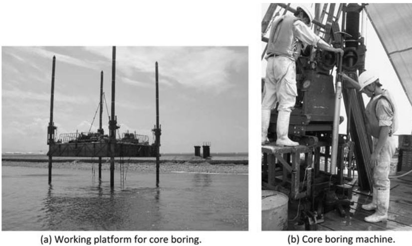
Figure 7.3 Core boring in marine construction.
