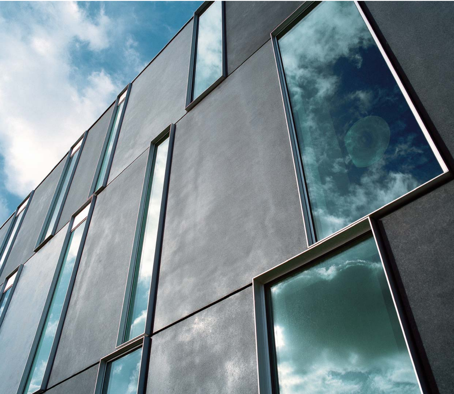
Storey-high panels and window openings
