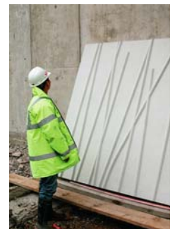
Panels in precast yard
