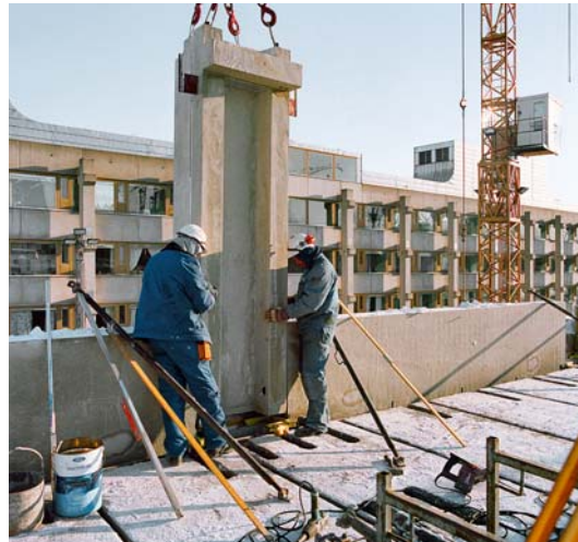
U-shaped precast column sits between spandrel edge beams
