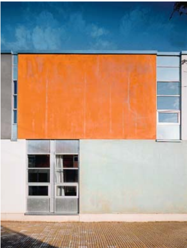
Chemically stained precast
