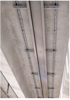
Services fit to underside of floor beams
