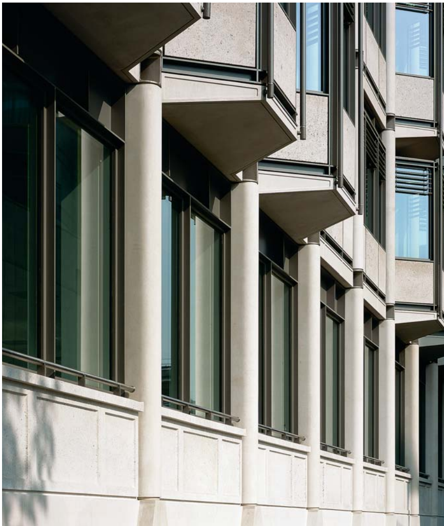
Bay windows keep rainwater away from GRC
