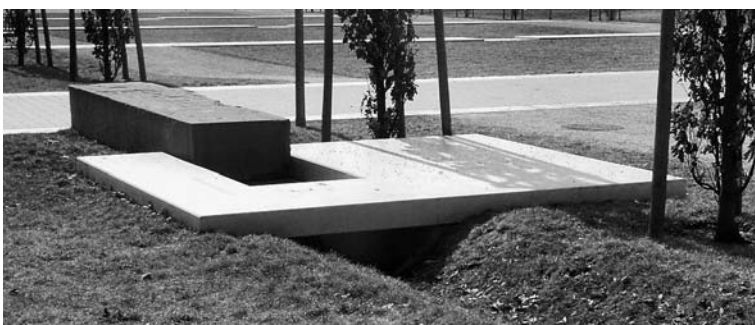
Detail of drainage outlet
