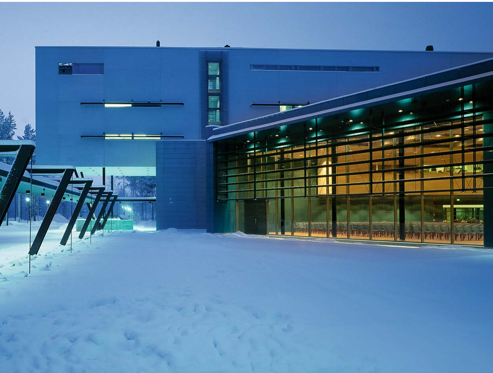
Administration building and auditorium from the east
