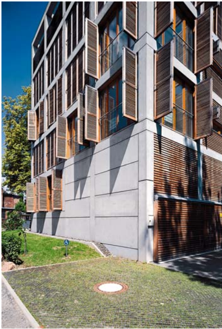
GRC panels and wooden shuttered windows
