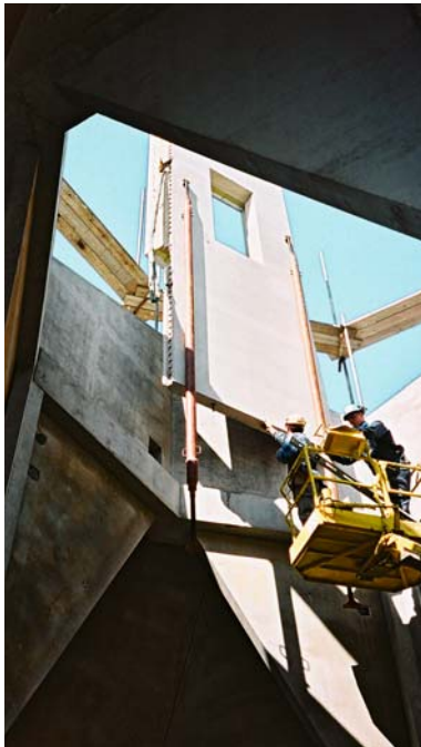
Construction of 'egg box' light well
