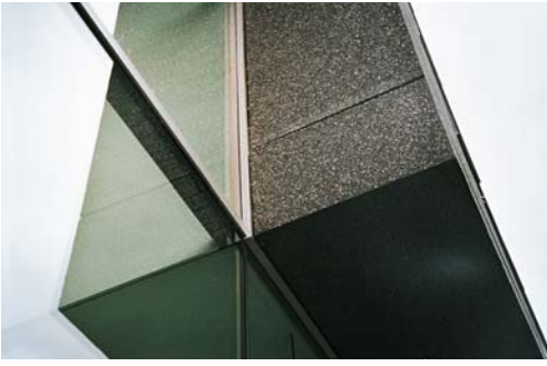
Soffit above entrance
