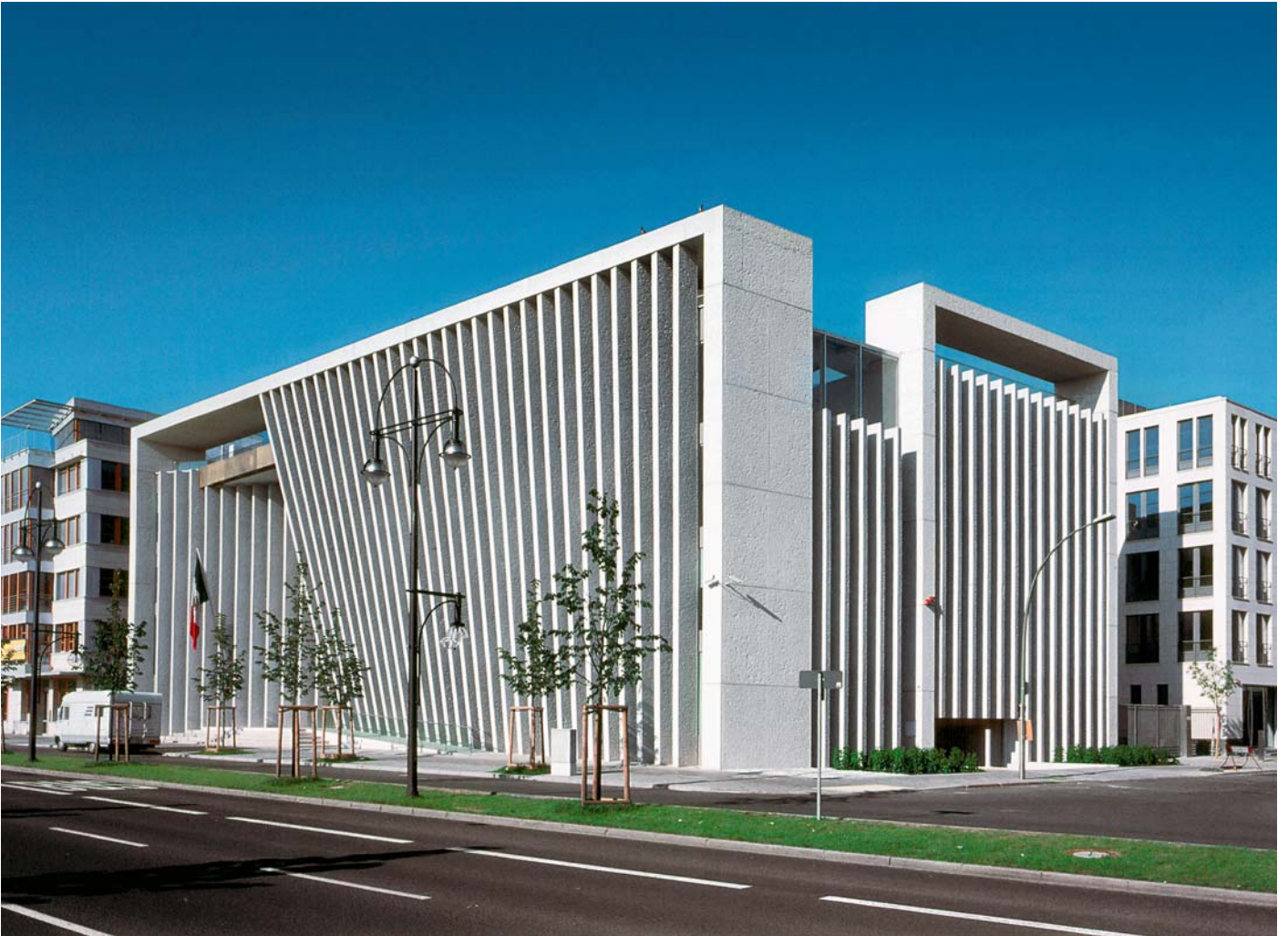
Portal framed blade beam elevations
