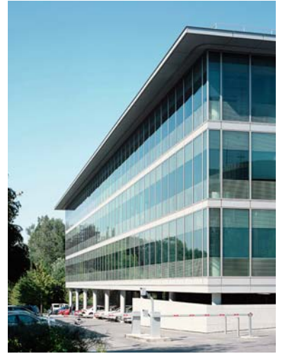
South-west long elevation and undercroft
