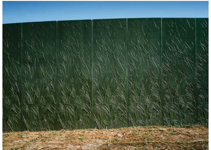
Close-up of precast wall
