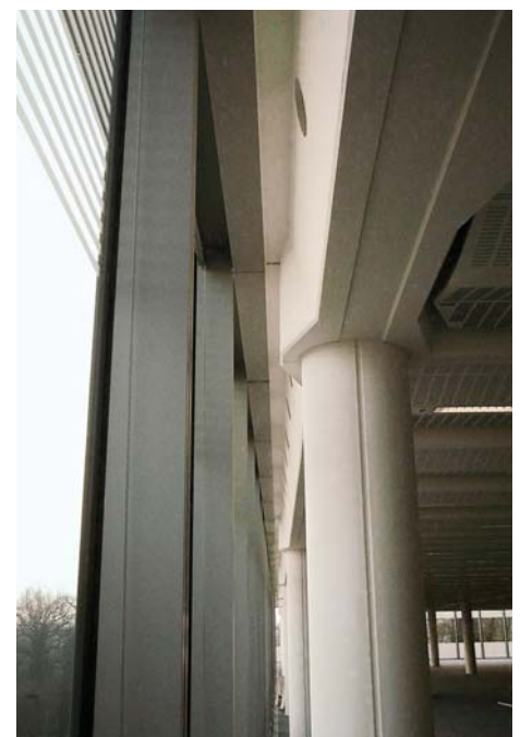
Precast structure exposed behind glass curtain wall
