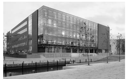
Main elevation, Tuborg 15 building
