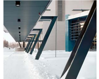
Covered walkway, cranked steel supports
