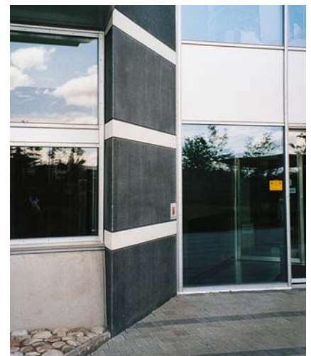
Views of base building façade
