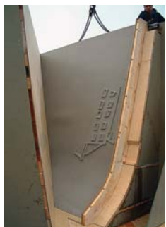
Casting the leading edge panel
