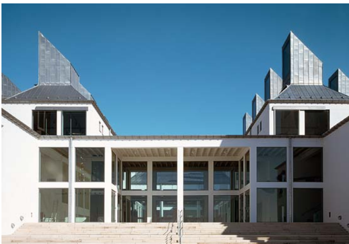
Main corridor and exit leading to waterfront
