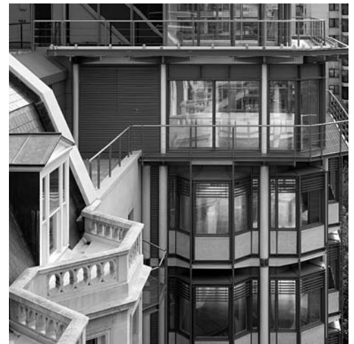
Existing building and new wing
