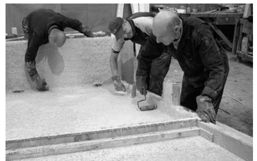
Top: Rolling and compacting GRC Bottom: Spraying GRC
