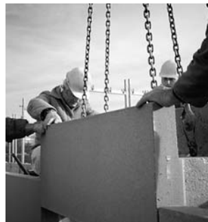
Laying the heavy precast stone blocks
