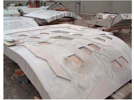
Precast panel before finishing
