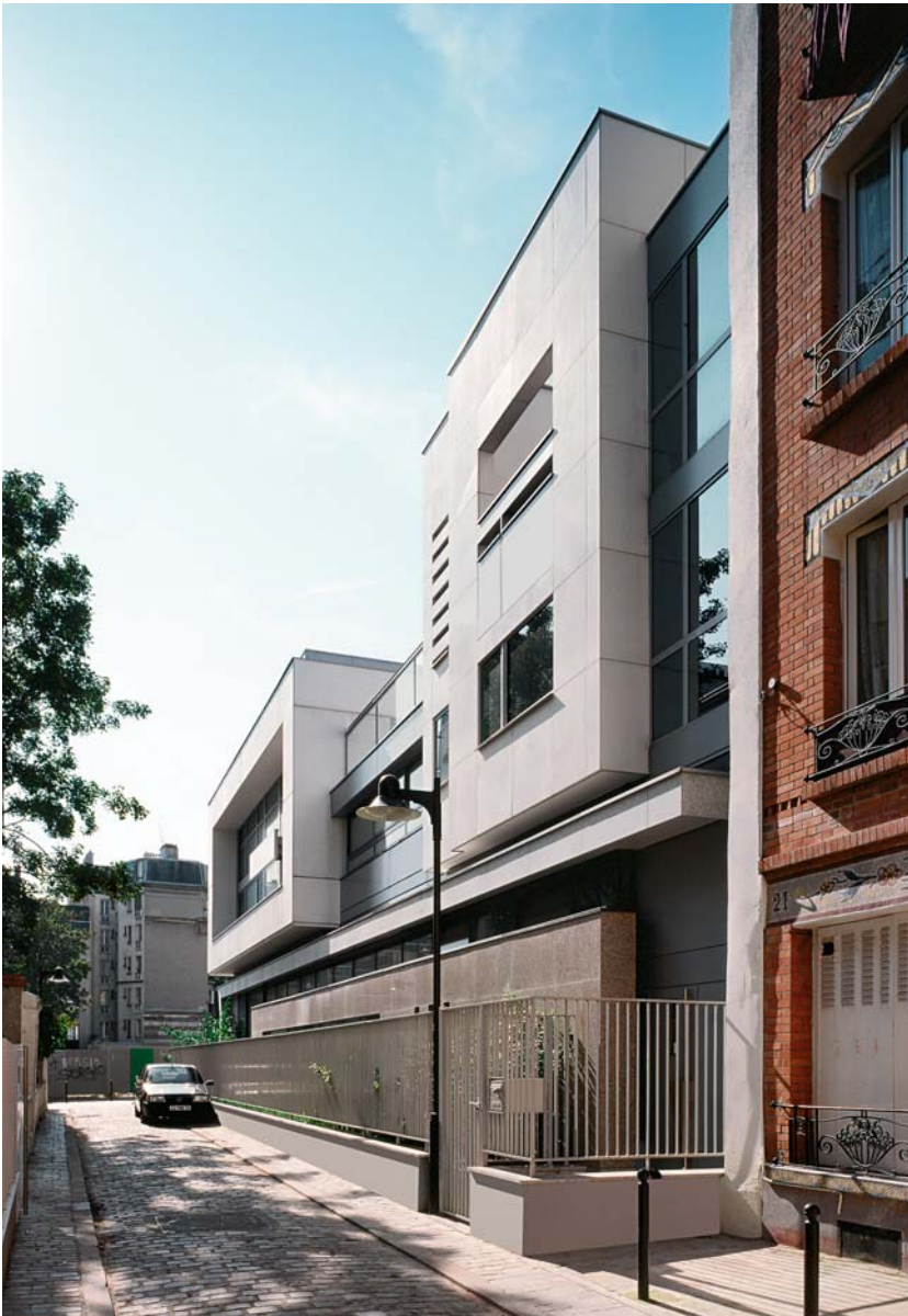
Street elevation (north side) and accommodation block in foreground
