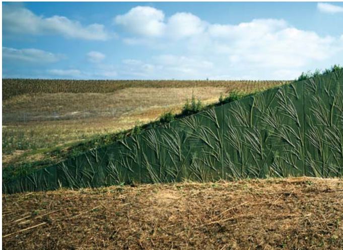
Precast wall with imprinted plants
