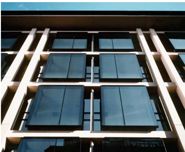
Precast façade set back from windows
