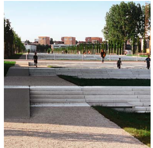
Precast terraces and central channel looking uphill
