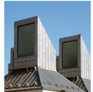
Completed lantern light well
