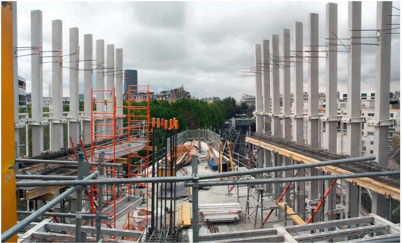
Construction of the upper floors
