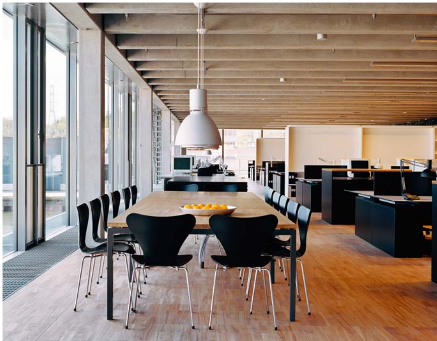
Exposed precast floor beams and columns
