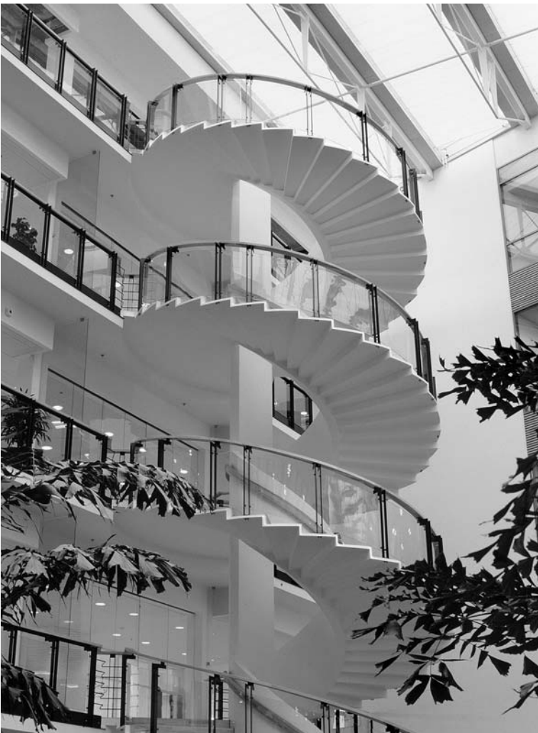
Cantilever treads and curved column profile
