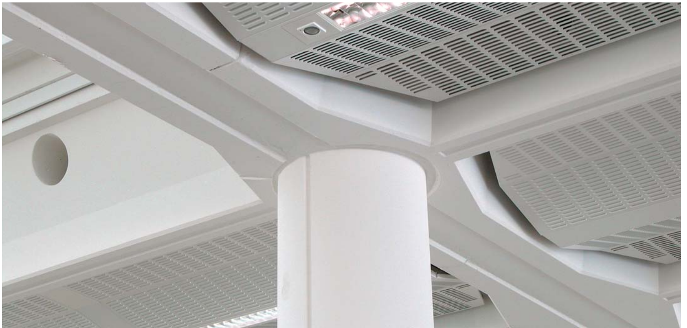
Exposed precast beam soffit at atrium corner and slotted ceiling panel
