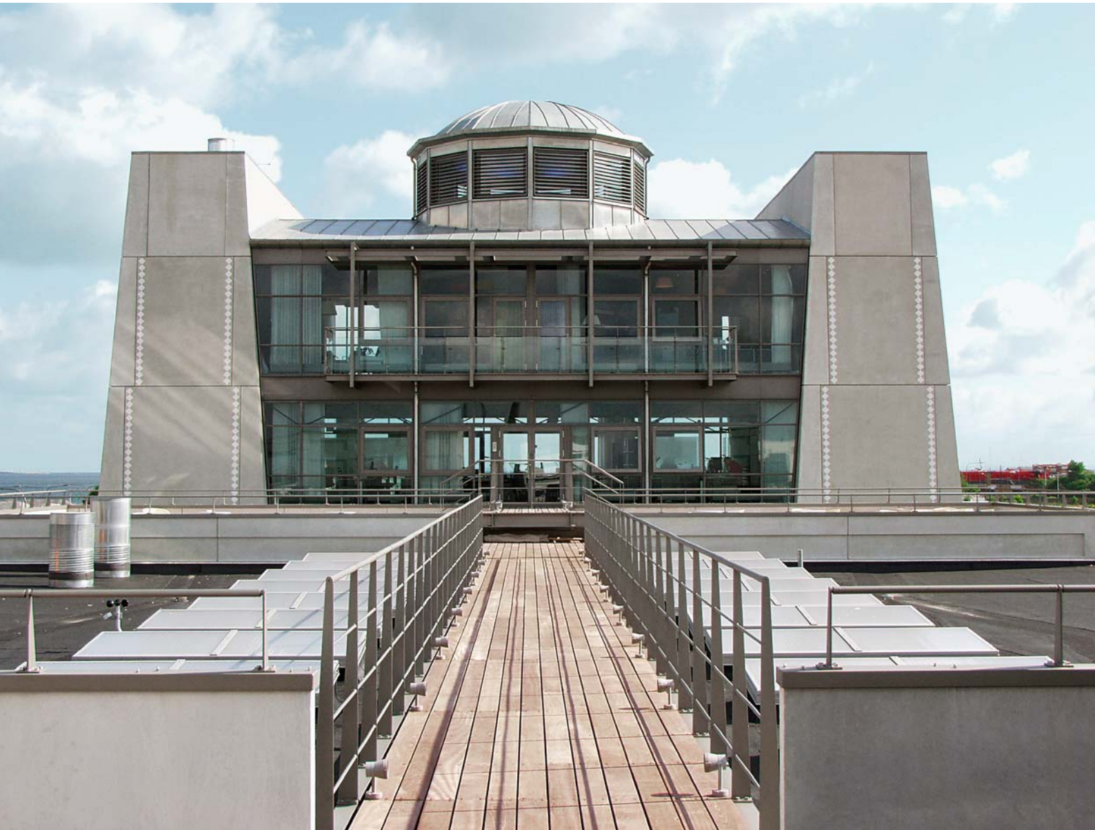
Roof level walkway above the production hall, looking towards the office building
