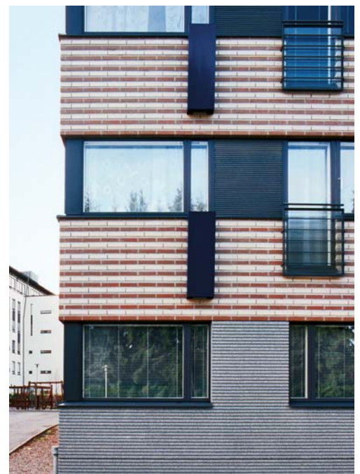
Ribbed finish to ground floor, brick faced above
