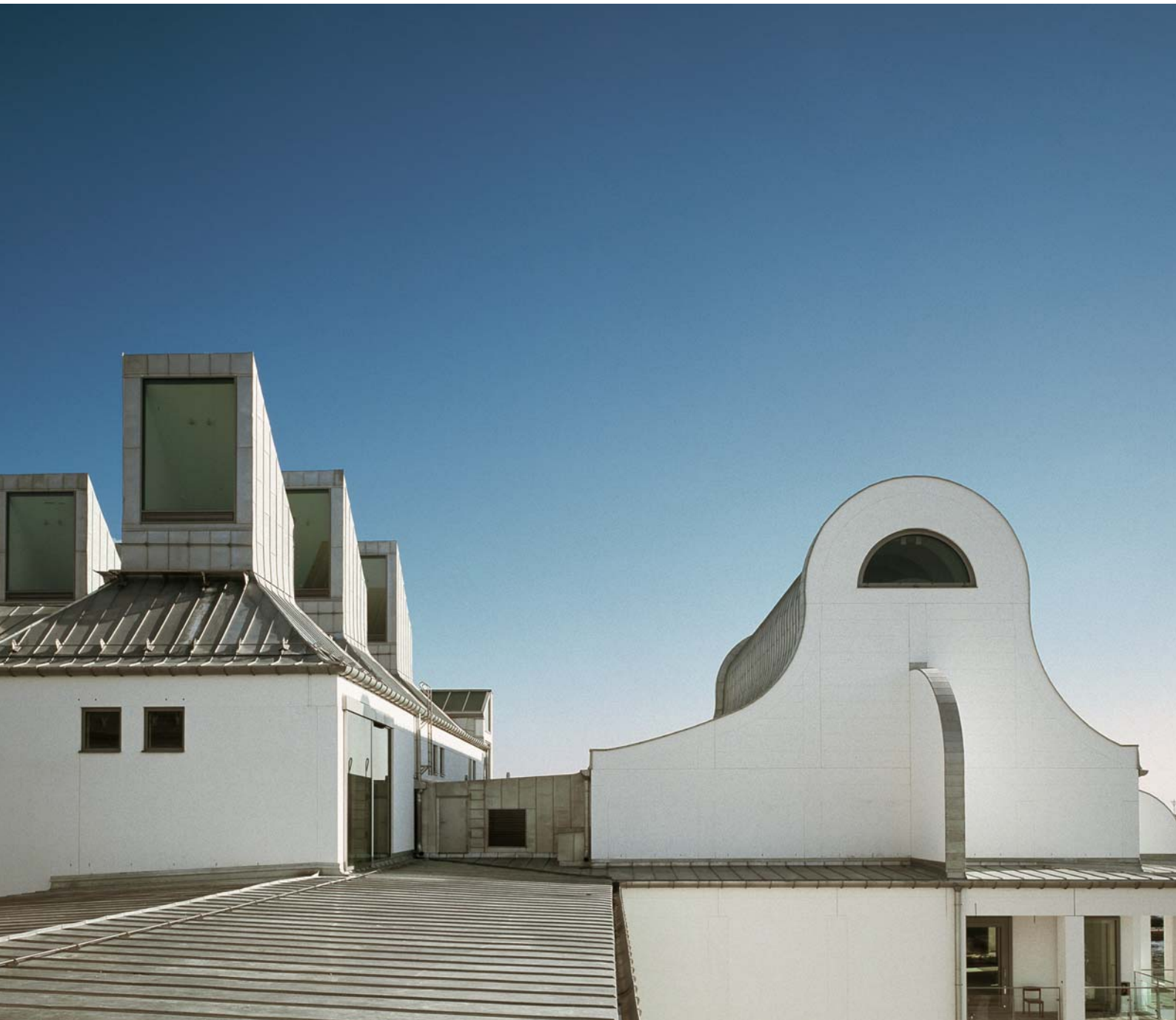
Lantern skylights and curved roof of concert hall
