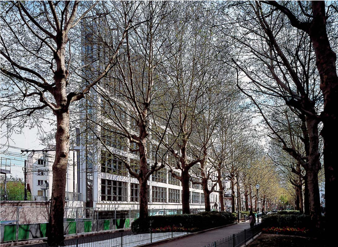
Front elevation seen from Avenue René Coty
