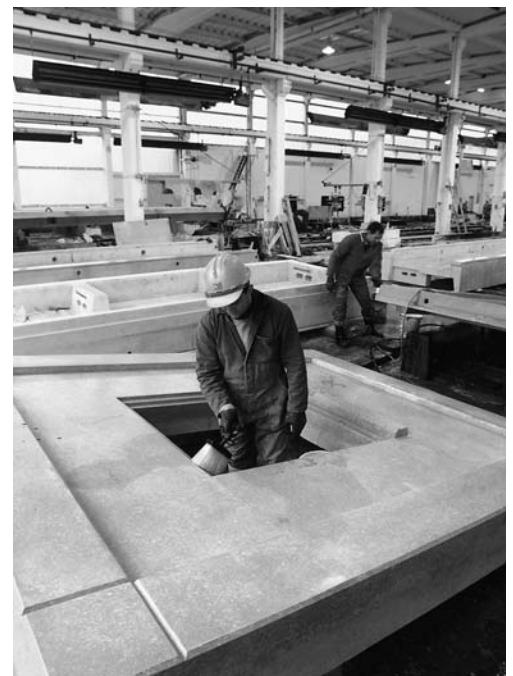
Cleaning edges of precast panel before despatch
