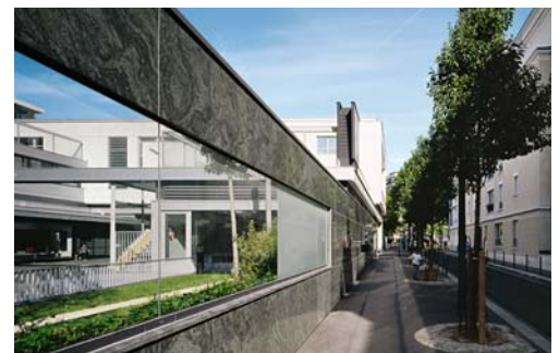
Glass panel 'fence' abutting street (south side)
