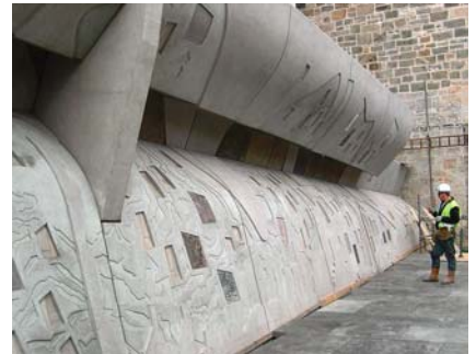
Canongate panel in position
