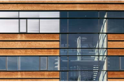
Pine cladding to elevation
