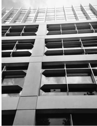
Crisp definition of precast structure and window grillage
