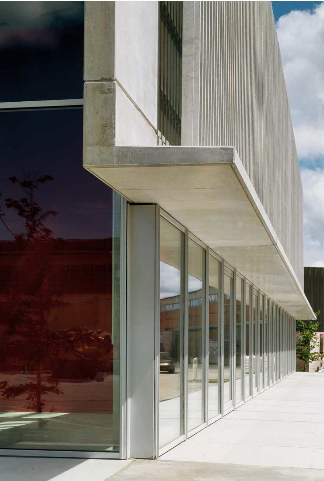
Canopy, glazing line and screen wall
