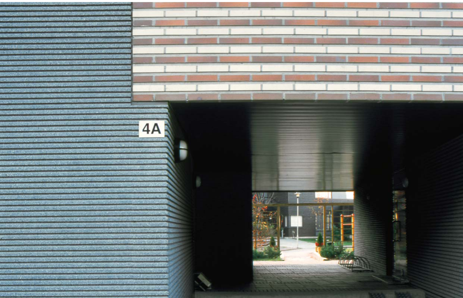
Access to the rear community garden and courtyard
