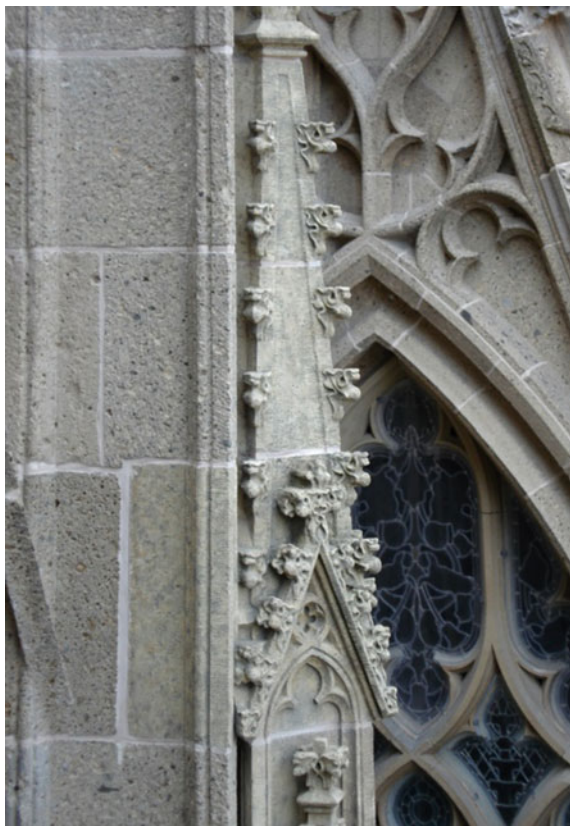
Fig. 6 Colour on Peperino Duro to visually match Weiberner tuff stone at St. Johns' Cathedral, 's-Hertogenbosch (photo: W. J. Quist)
