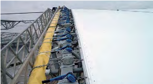
Fig. 100: Pulling in and tensioning the membrane for the stand roofing at stadium Volkswagen Arena Wolfsburg, Germany
