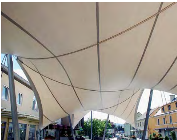
Fig. 95: Diagonally arranged uplift ropes underneath an awning surface
