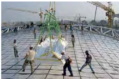
Fig. 274: Lifting in the outer membrane
