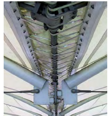
Fig. 134: left: Erection of valley for the roof over the Sony Center in Berlin, Germany; right: Valley detail at the Gottlieb Daimler Stadion in Stuttgart, Germany
