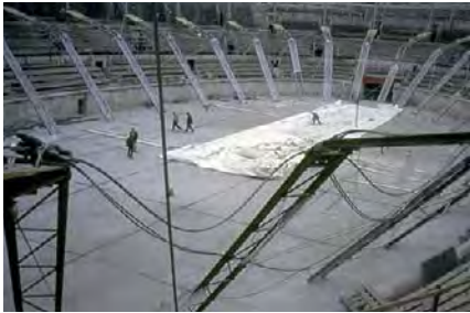
2 Laying out the rope net and the lower membrane
