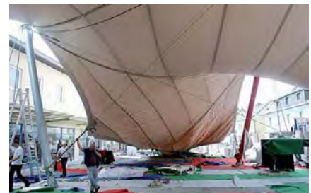
d Interior view with temporary stays
