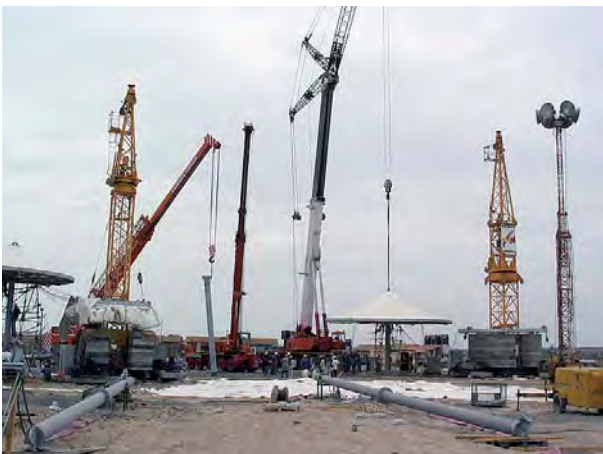
Fig. 213: Use of cranes in membrane construction; left: Truck crane with telescopic boom, lattice-boom crane; right: Tower crane
