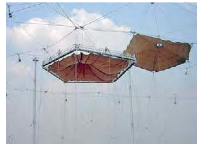
Fig. 260: Lifting up a membrane panel
