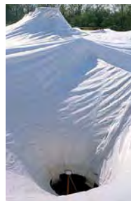
Fig. 246: Erection procedure – high point surface
