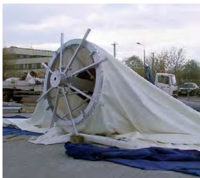
Fig. 299: left: Pre-assembled high point; right: Preassembly of a low point
