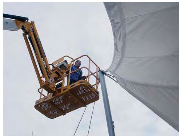
Fig. 196: Articulated and telescoping platform in use for the erection of a pneumatic pillow and the erection of a four-point awning
