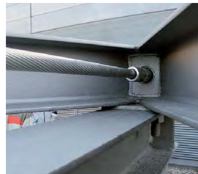
Fig. 232: left: Hinged support on arch; middle: Connection of the diagonal struts to the longitudinal rope; right: Rope connection to the horizontal framing
