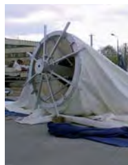
Fig. 245: Erection of an internally supported high point surface
