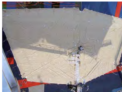
Fig. 259: Preassembly of membrane panel
