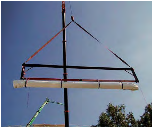
Fig. 168: Load suspension and load transfer devices for lifting a rolled membrane
