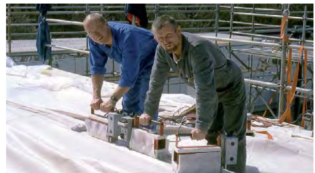
Fig. 118: left: Repair work with a hot air pistol; right: Welding of partial surfaces of Glass/PTFE membrane at the Munich Waste Management Office (AWM), Germany
