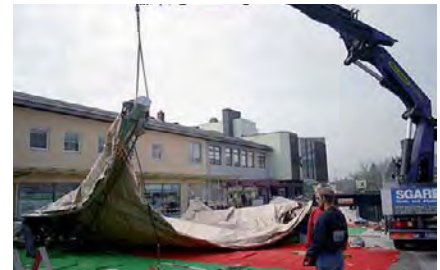
b Pivoting of the first mast
