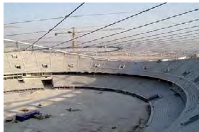
Fig. 249: Single layer ropenet construction
