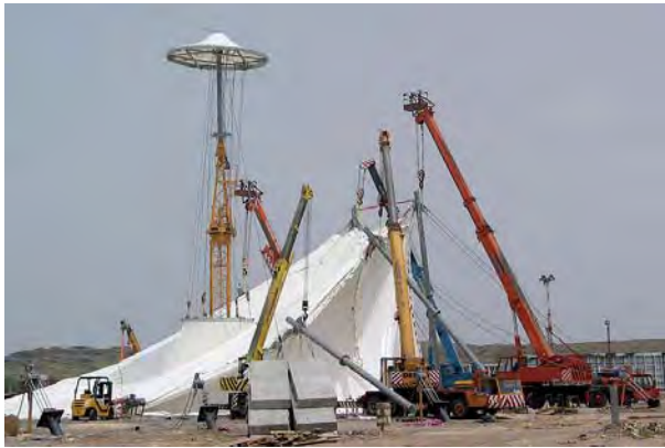
Fig. 202: Temporary state during the erection of a high point roof
