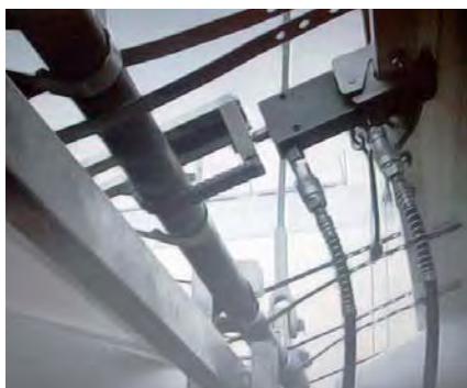
Fig. 347: Tensioning a clamping clip edge
