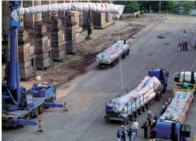
Fig. 308: Lifting of rolled membrane for the wrapping of the Reichstag in Berlin, Germany
