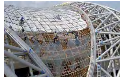
Fig. 273: Installation of the polycarbonate boards
