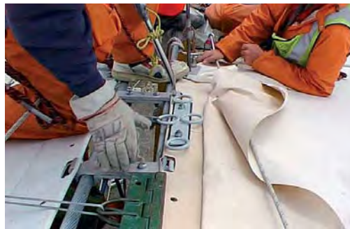
Fig. 343: Transverse tensioning of a keder rail edge (Glass/PTFE fabric)
