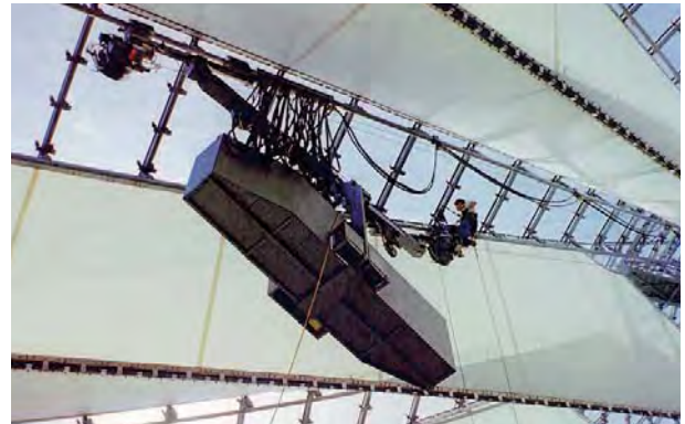
Fig. 198: Travelling platforms for the membrane erection of the Tropical Island in Brand and for the Forum roof in the Sony Center in Berlin
