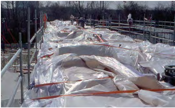
Fig. 195: Use of system scaffolding as working platforms for the installation of membrane surfaces
