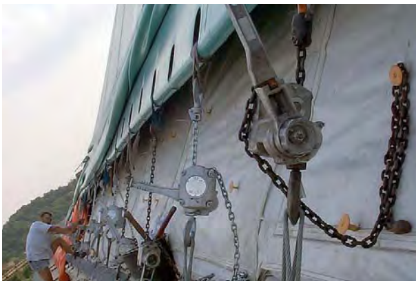
Fig. 346: left: Tensioning a tube edge; right: Tube edge against standing bolts
