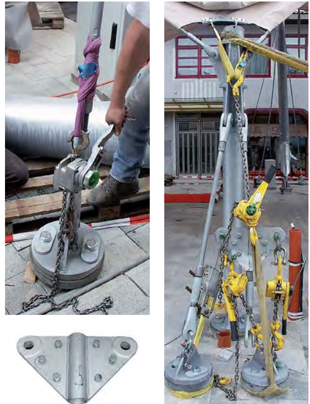
Fig. 182: Tensioning a stay rope with ratchet lever hoists and butterfly plates
