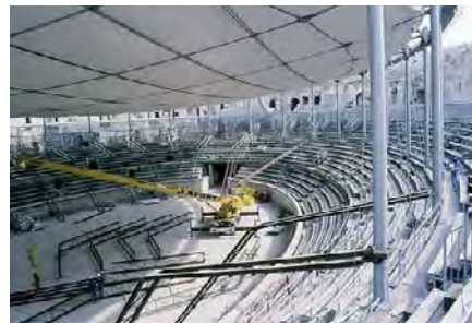
10 Dismantling the temporary bridge
