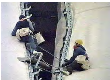
Fig. 279: Roof erection at the stadium in Riyadh, Saudi Arabia
