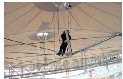
Fig. 253: Application of the pretension
