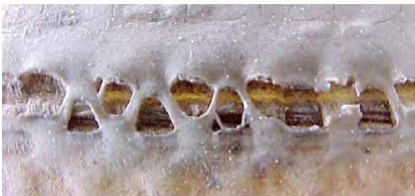
Fig. 50: Polyester fabric exposed through breakdown of the coating
