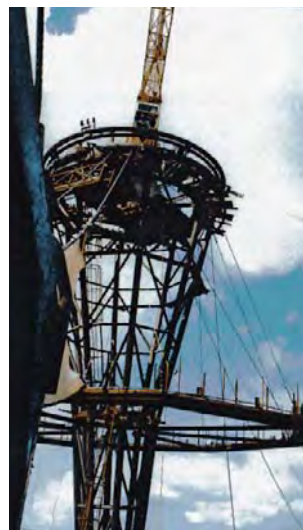
Fig. 226: left: Foot point of the king truss with cable anchorage nodes; middle: Head part of the king truss; right: King truss sections
