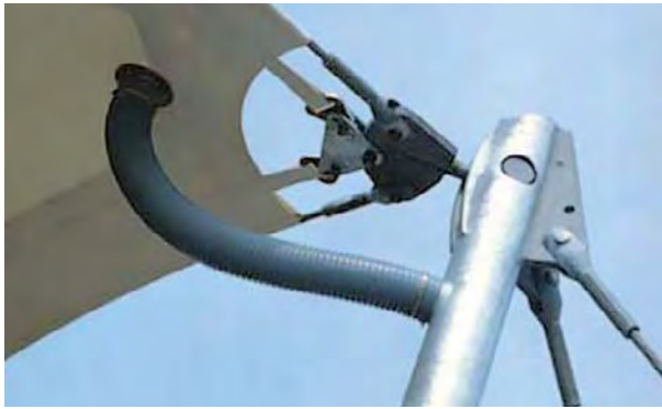
Fig. 39: Webbing fixing to corner fitting
