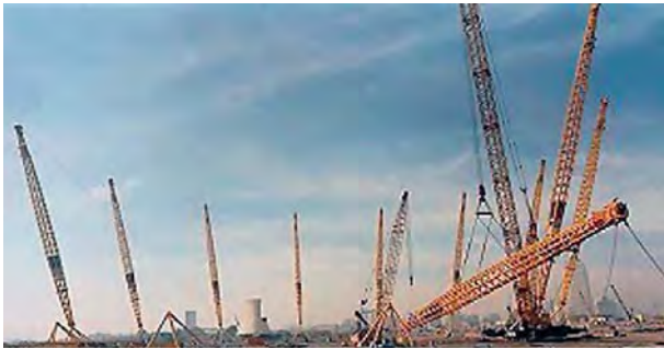
Fig. 219: Lifting the masts at the Millennium Dome in London, England
