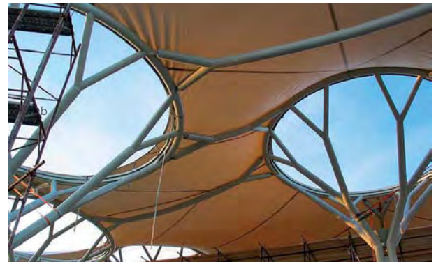
d) Installation of low point membrane
