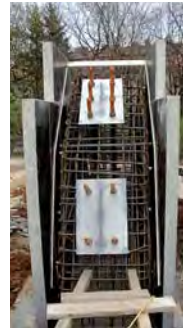
Fig. 34: left: Crosshead with threaded tie bars; middle: Tolerance adjustment for highly loaded cables; right: Tensioning equipment
