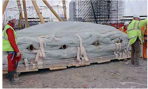
Fig. 294: left: Folded package – roofing of the amphitheatre in Nîmes; right: Folded package – roofing of the Millennium Dome in London, England
