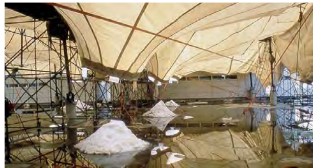
Fig. 360: Erection of the compartmental high point surface at the Munich Waste Management Office, Germany
