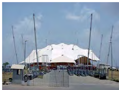
Fig. 262: Erection of edge panels
