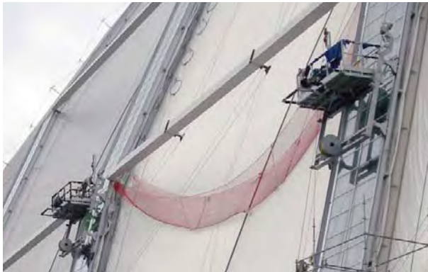
Fig. 198: Travelling platforms for the membrane erection of the Tropical Island in Brand and for the Forum roof in the Sony Center in Berlin
