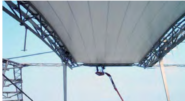
Fig. 100: Pulling in and tensioning the membrane for the stand roofing at stadium Volkswagen Arena Wolfsburg, Germany
