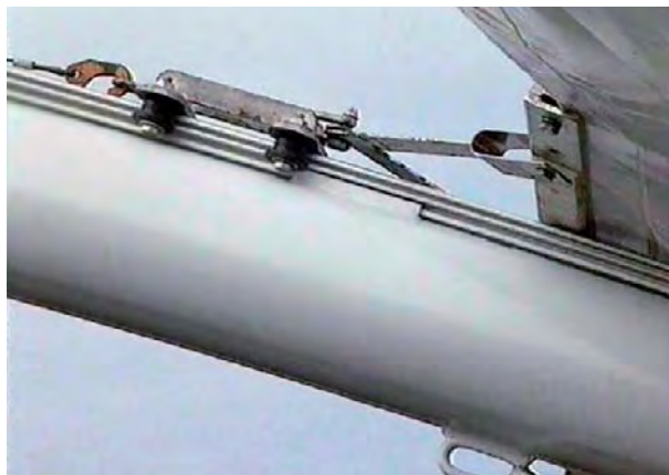
Fig. 189: Pulling in the membrane for the roofing over of the Gottlieb Daimler Stadion in Stuttgart, Germany
