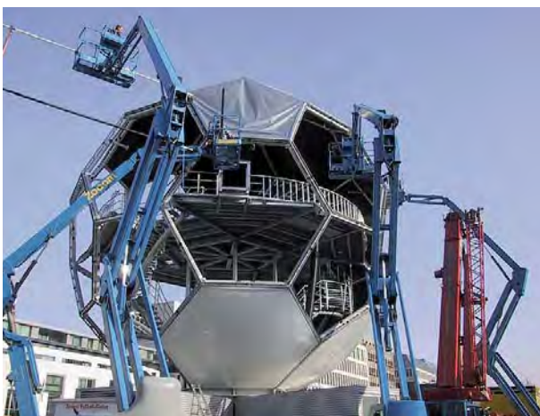
Fig. 196: Articulated and telescoping platform in use for the erection of a pneumatic pillow and the erection of a four-point awning
