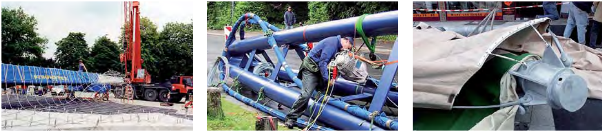
Fig. 218: Preparatory work left: for pivoting; middle: for lifting; right: Pylon head with preassembled membrane
