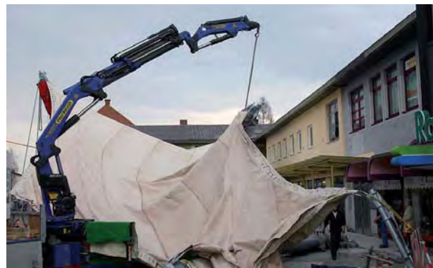
b) Erection of an awning
