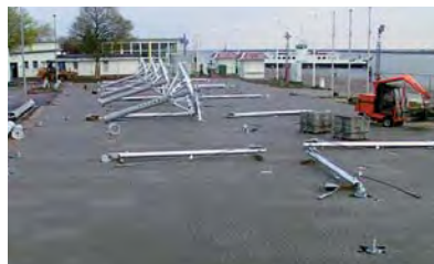
Fig. 244: Erection procedure – high point surface
