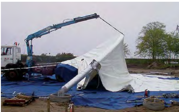
c) Erection of an arch membrane
