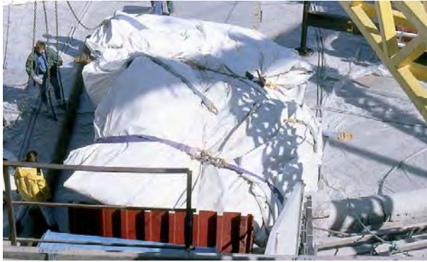
Fig. 294: left: Folded package – roofing of the amphitheatre in Nîmes; right: Folded package – roofing of the Millennium Dome in London, England
