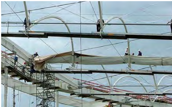
c) Installation of arch membrane
