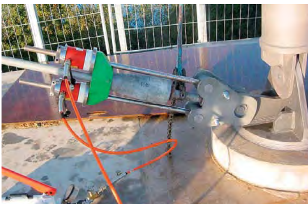
Fig. 172: left: Tensioning set-up for a stay rope; right: Tensioning set-up for a group of ropes
