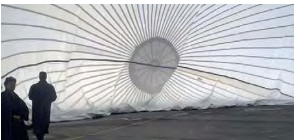
Fig. 365: Fabric membrane during the inflation of an air-supported hall
