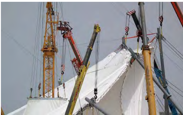
a) Erection of a high point structure
