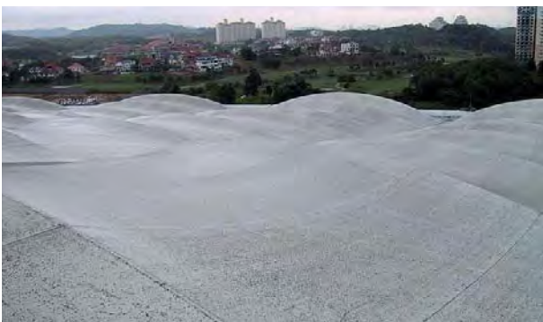
Fig. 54: Separation of coating from a polyester/PVC fabric caused by fungal attack
