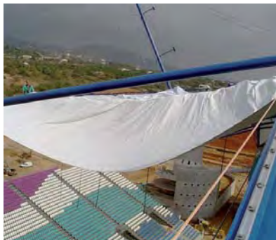
Fig. 101: Pulling in and tensioning the membrane for the stand roofing at Estádio Intermunicipal Faro, Portugal
