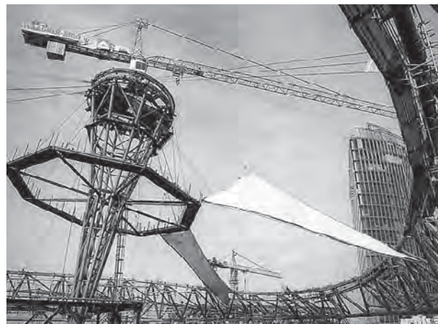
Fig. 213: Use of cranes in membrane construction; left: Truck crane with telescopic boom, lattice-boom crane; right: Tower crane
