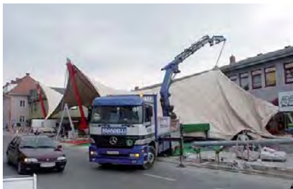
Fig. 334: Erection of the roof over the marketplace in Zeltweg, Austria
