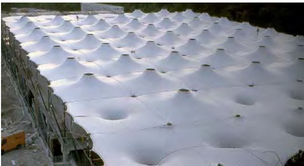
Fig. 360: Erection of the compartmental high point surface at the Munich Waste Management Office, Germany
