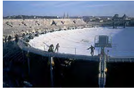
7 Spanning the festoon ropes to the compression ring
