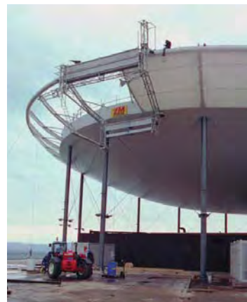
Fig. 199: Mobile working platform for membrane erection at Neuchâtel, Switzerland
