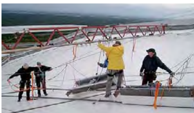
Fig. 284: Installation of the GRP gutter
