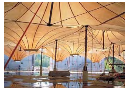
Fig. 246: Erection procedure – high point surface
