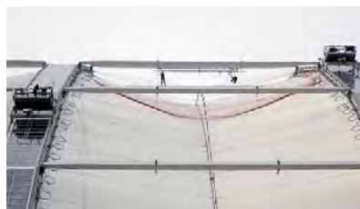
Fig. 285: Access unit and rope traverse
