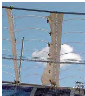
Fig. 265: Erection sequence – Arch membrane and detail of arch crown
