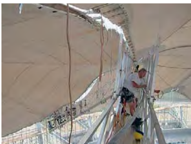
Fig. 261: Connecting a membrane panel
