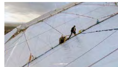
Fig. 286: Installation of the foil pillow
