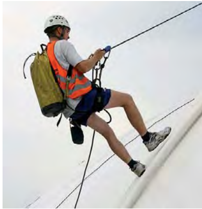
Fig. 200: Abseil work for membrane erection
