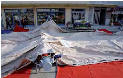
b Pivoting of the first mast
