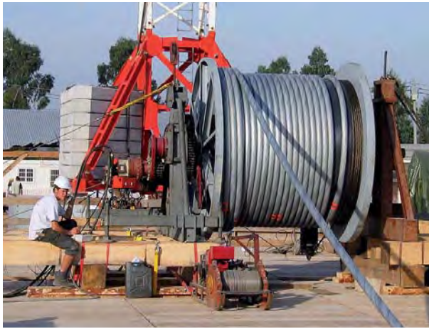
Fig. 290: Unrolling rope from a braked stand
