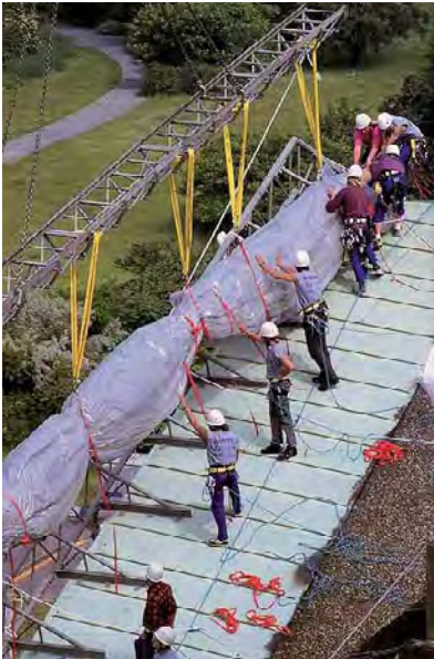
Fig. 308: Lifting of rolled membrane for the wrapping of the Reichstag in Berlin, Germany
