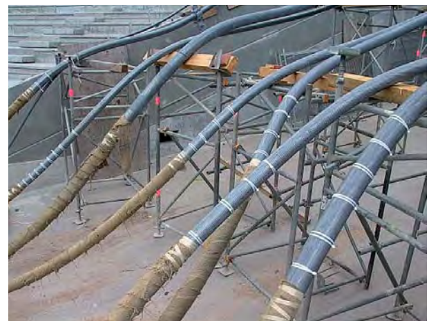
Fig. 291: left : Laying out the carrier cable at the stadium in Braga, Portugal; middle, right : Preassembly of the cable structure at the Waldstadion in Frankfurt/M., Germany
