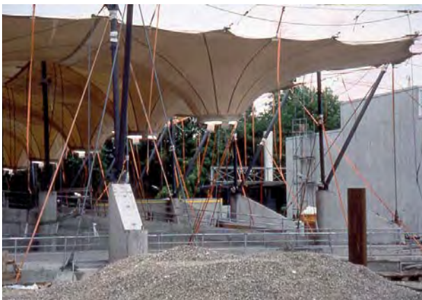
Fig. 201: left: Stabilising the primary structure during the erection of the roof over the carport at the Munich Waste Management Office; right: Stabilising the wire rope construction at the Millennium Dome in London, England
