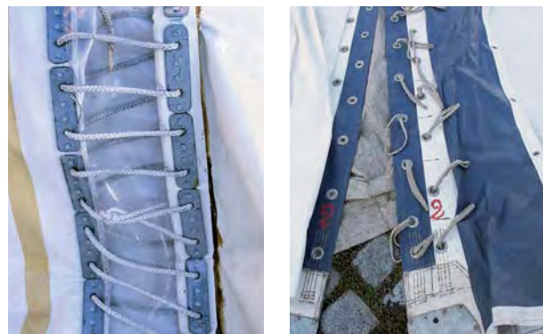
Fig. 125: left : Laced connection of the large pillow of the arena in Nîmes, France; right : Loop joint of a circus tent
