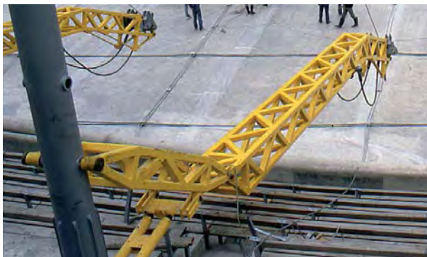
Fig. 318: Distance beam, telescopic beam and lattice boom
