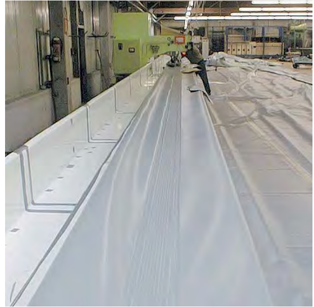
Fig. 114: Welding under pretension
