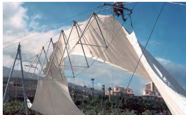
d) Erection of high point structures
