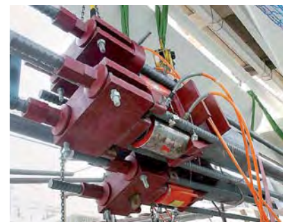
Fig. 215: left: Apparatus for tensioning stay rope; middle: Apparatus for tensioning carrier rope; right: Apparatus for tensioning stay rope
