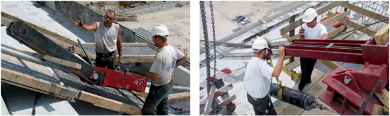
Fig. 177: left: Installation of the rope clamp and the deflection system; right: Installation of the guide traverse and hanging the rope
