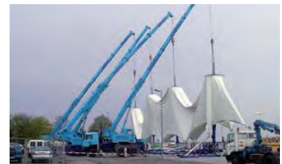
Fig. 244: Erection procedure – high point surface
