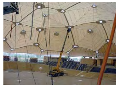
Fig. 263: Application of the pretension
