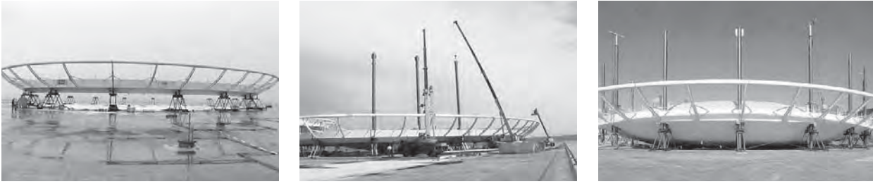
Fig. 330: left: Preassembled compression ring; middle: Lifting the columns; right: Preassembled pillow
