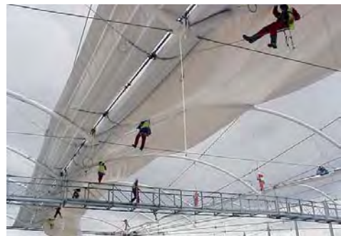
Fig. 265: Erection sequence – Arch membrane and detail of arch crown
