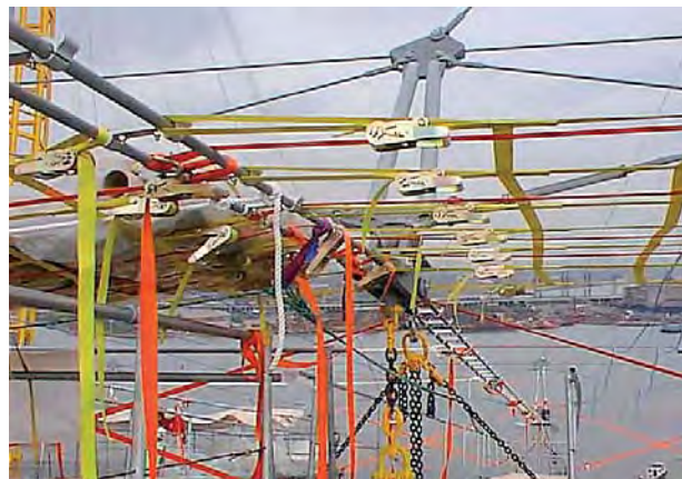
Fig. 201: left: Stabilising the primary structure during the erection of the roof over the carport at the Munich Waste Management Office; right: Stabilising the wire rope construction at the Millennium Dome in London, England
