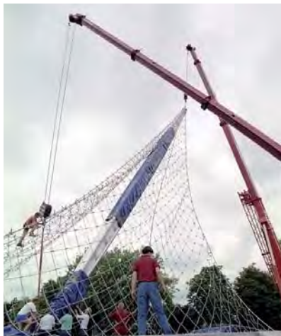
Fig. 220: Pivoting a mast with preassembled rope net
