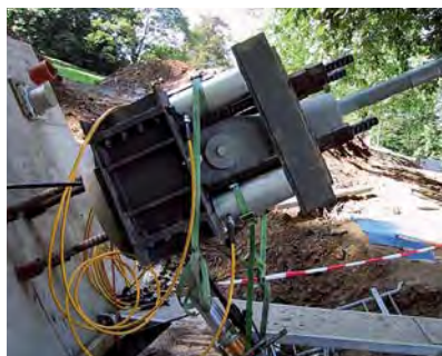
Fig. 215: left: Apparatus for tensioning stay rope; middle: Apparatus for tensioning carrier rope; right: Apparatus for tensioning stay rope
