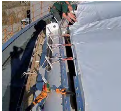
Fig. 342: Tensioning a clamping plate edge (PES/PVC fabric)
