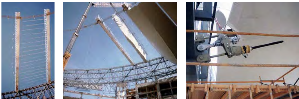
Fig. 277: Erection sequence – ridge and valley surface
