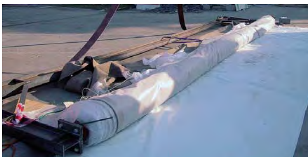
Fig. 296: Rolled membrane surface and unrolling mechanism
