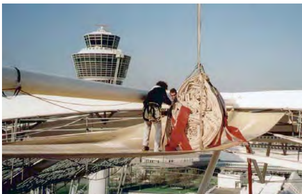
Fig. 306: Lifting and unfolding a folded package for the erection for the Airport Center in Munich, Germany
