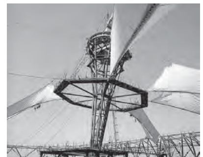
Fig. 209: Diagonally alternating installation of the Forum roof of the Sony Center in Berlin, Germany ( bottom ) and at the Millennium Dome in London, England ( top )
