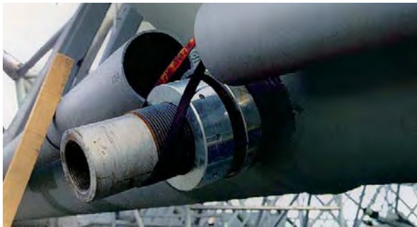
Rope anchorage to edge beam
