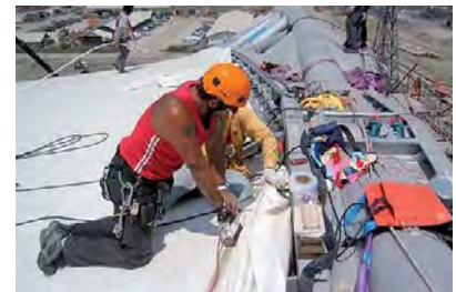
Fig. 276: Welding the covering membrane
