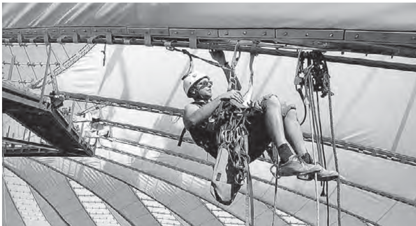
Fig. 134: left: Erection of valley for the roof over the Sony Center in Berlin, Germany; right: Valley detail at the Gottlieb Daimler Stadion in Stuttgart, Germany
