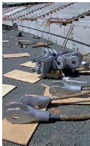
Fig. 291: left : Laying out the carrier cable at the stadium in Braga, Portugal; middle, right : Preassembly of the cable structure at the Waldstadion in Frankfurt/M., Germany
