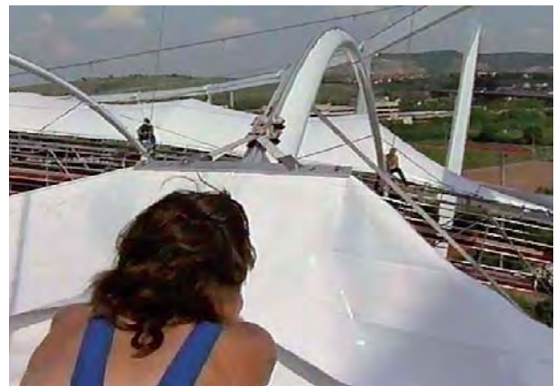
Fig. 189: Pulling in the membrane for the roofing over of the Gottlieb Daimler Stadion in Stuttgart, Germany
