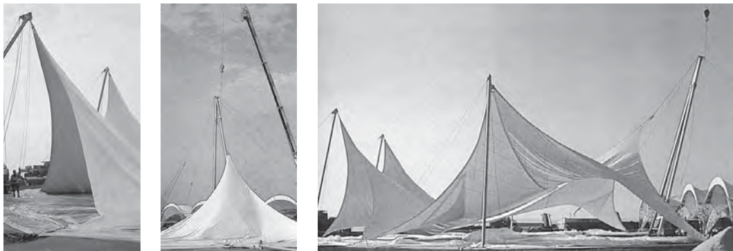
Fig. 243: Erection of a multi-point awning
