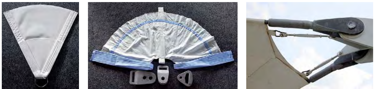
Fig. 145: left : Webbing corners with continuous and butted webbing; right : Rope corner with tangential webbing
