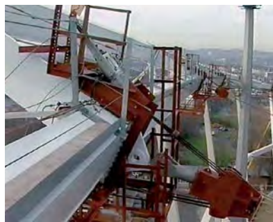
Fig. 215: left: Apparatus for tensioning stay rope; middle: Apparatus for tensioning carrier rope; right: Apparatus for tensioning stay rope
