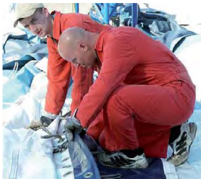
Fig. 298: Joining the panels of a circus tent
