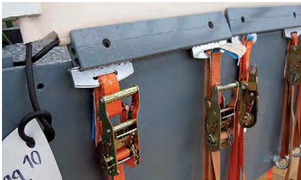
Fig. 193: Tensioning a keder rail edge at the control tower in Vienna airport, Austria
