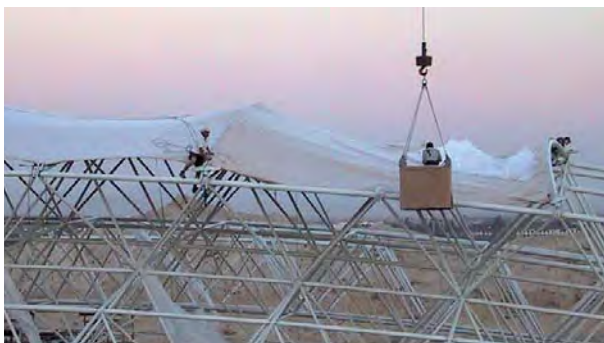
Fig. 350: Erection of the stand roofing at the stadium in Al Ain, Dubai, United Arab Emirates
