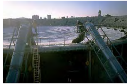
8 Connecting the blower units
