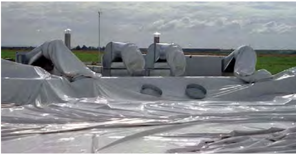
Fig. 364: left: Inflation connections for an air-supported hall; right: Blower plant for a large pillow
