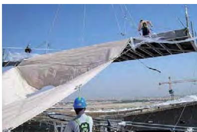
Fig. 251: Pulling the membrane off the package from a temporary platform
