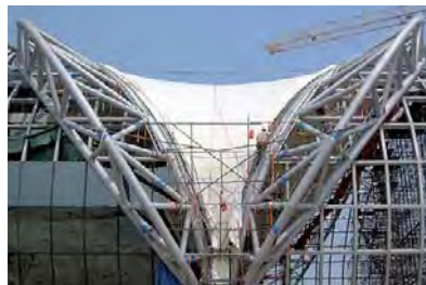
Fig. 275: Tensioning the outer membrane
