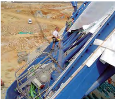
Fig. 101: Pulling in and tensioning the membrane for the stand roofing at Estádio Intermunicipal Faro, Portugal
