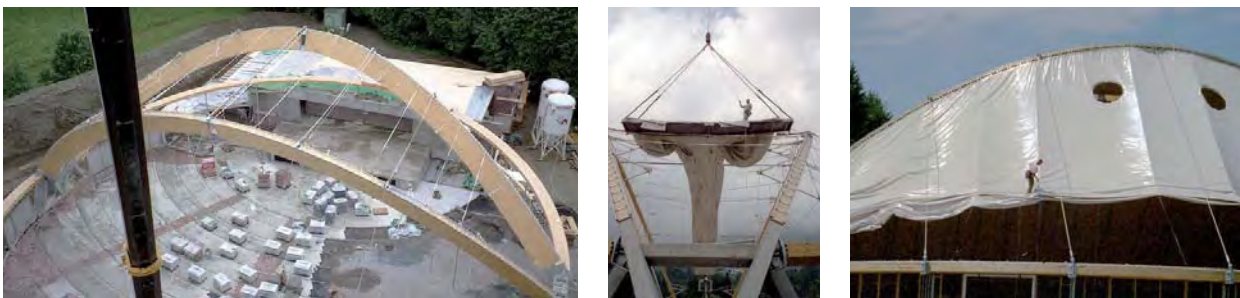
Fig. 270: Erection variant for arched construction
