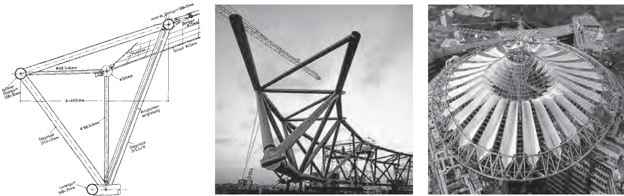
Fig. 227: left, middle: Three-chord ring truss; right: Completed roof
