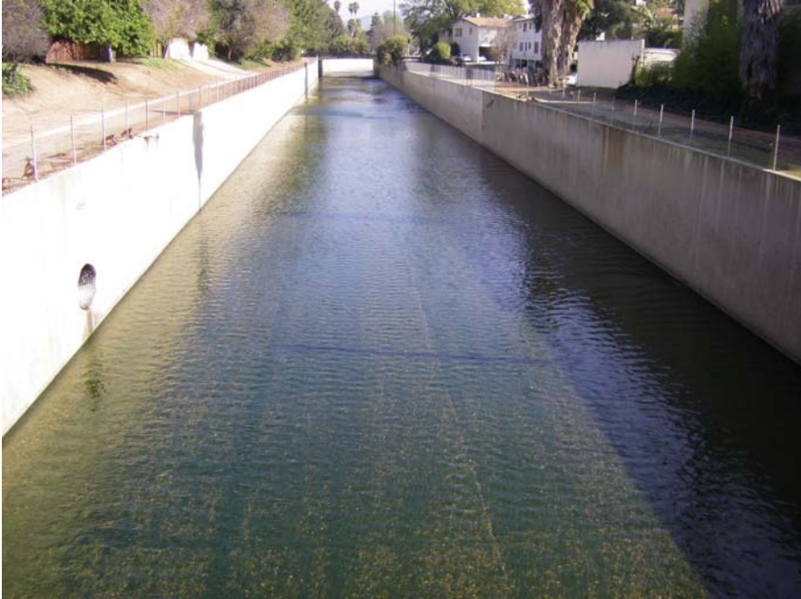
Fig. 6.2 View of a non-alluvial channel, whose boundaries cannot be modified under the current discharge regime (Los Angeles River, California)
