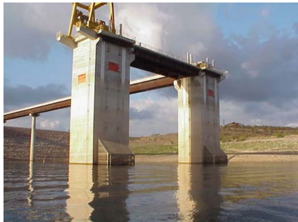
Fig. 4.3 Photographs of a typical outlet structure located in a reservoir (Lake Pleasant, Arizona)
