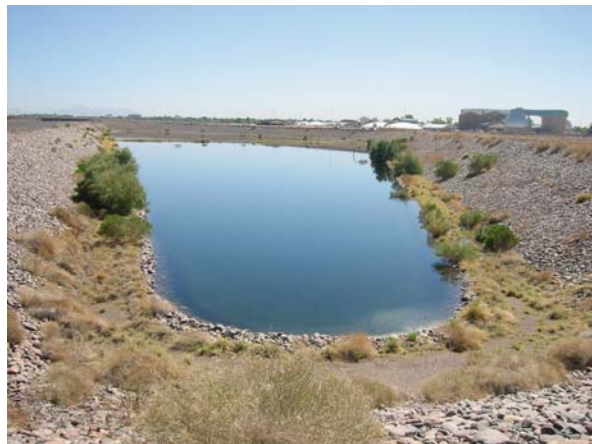
Fig. 4.4 Recharge basin located near a river channel that has high soil permeabilities. A wastewater treatment plant is located in the background, and treated wastewater flows into this recharge basin to supplement regional groundwater supplies
