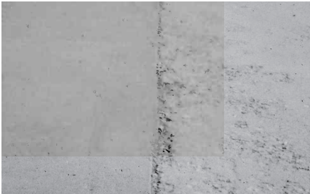
Figure 9.28 (See color insert.) Adjacent concrete slabs on paved parking lot in Wisconsin; both slabs contain 40% Class F fly ash. Slab to left placed and finished by slipform paving machine. Slab to right placed and finished by hand.
