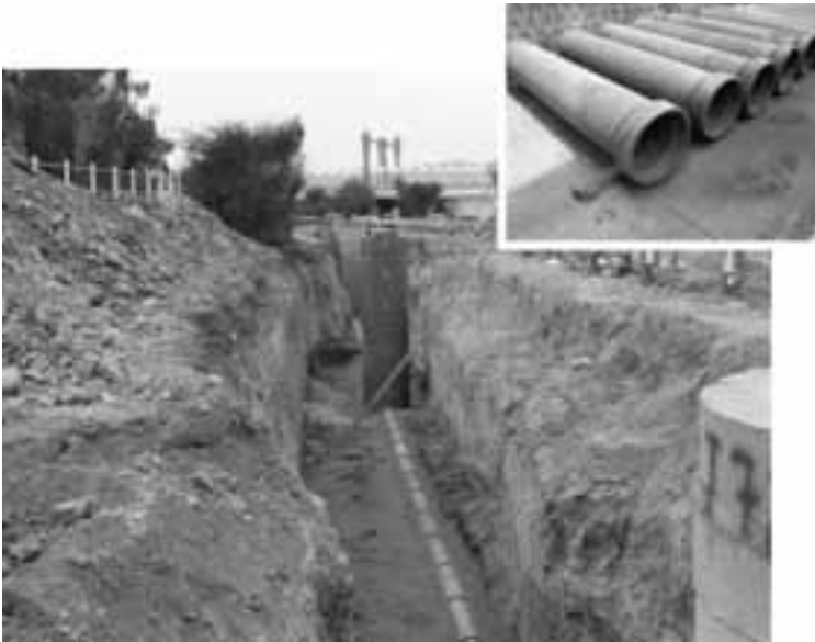
Figure 7.10. Placed modified-sulfur concrete pipes and manhole within the sewerage distribution system in Al Ain, United Arab Emirates, by Nippon Oil Corporation, Japan, in January 2009.
