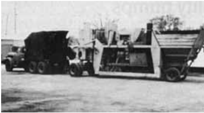
Figure 7.11a. Special heated concrete mixer (left) and aggregate dryer/superheated (right) for sulfur concrete application (Pickard, 1985).
