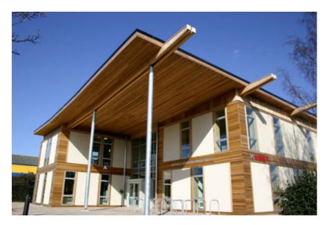
Fig. 2. Media Centre in Bristol constructed from straw bales
