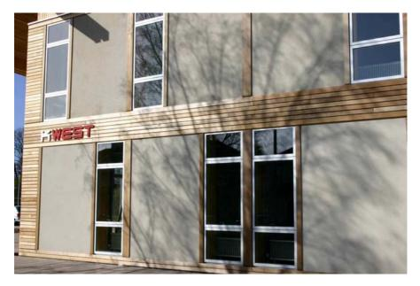
Fig. 1. ModCell Panels used at Knowle West Media Centre, Bristol
