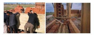
Fig. 4. The straw compound wall under construction
