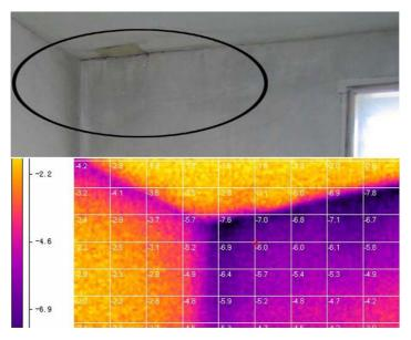
Fig. 1. The status and temperature distribution of interior surface of the exterior walls of traditional rural house in winter in Northern China
