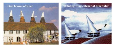
Fig. 1. Traditional and modern rotating wind catcher at Bluewater shopping malls, Kent
