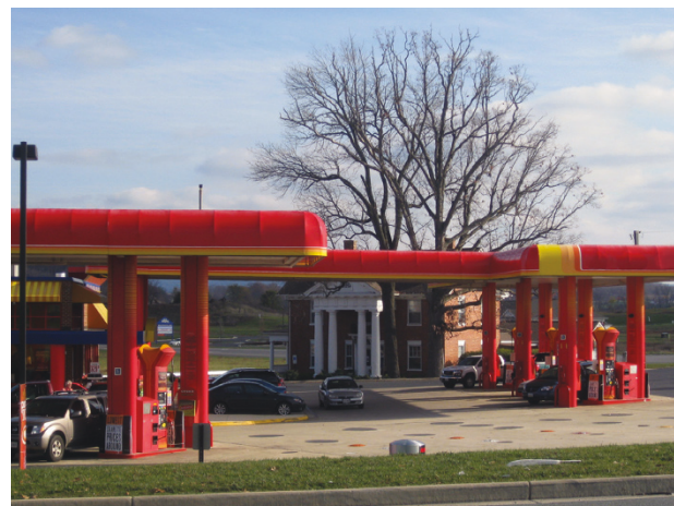
This gas station destroys the historic context for this historic home’s site.
