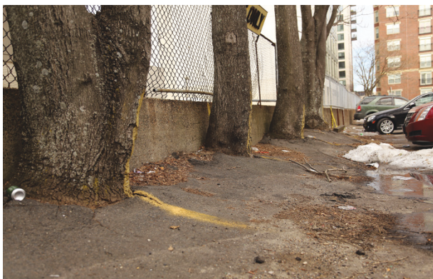
Poor tree planting; not enough room to grow
