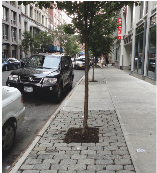
Good tree planting: Pavers allow water and air to enter and may be removed as the tree grows
