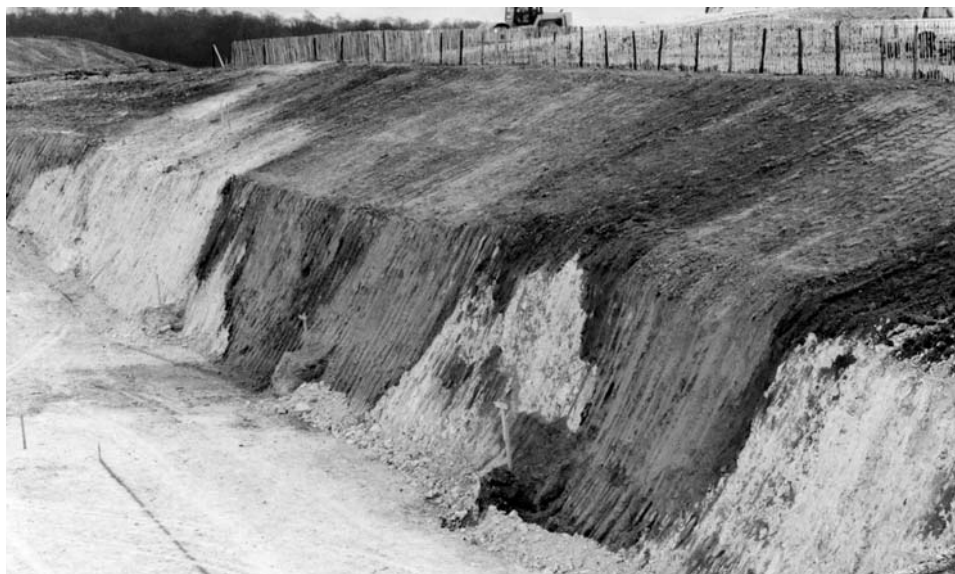
Figure 1.10. Large buried sinkholes filled with clay soils (locally known as chalk pipes) exposed in a road cutting through the chalk in southern England.
