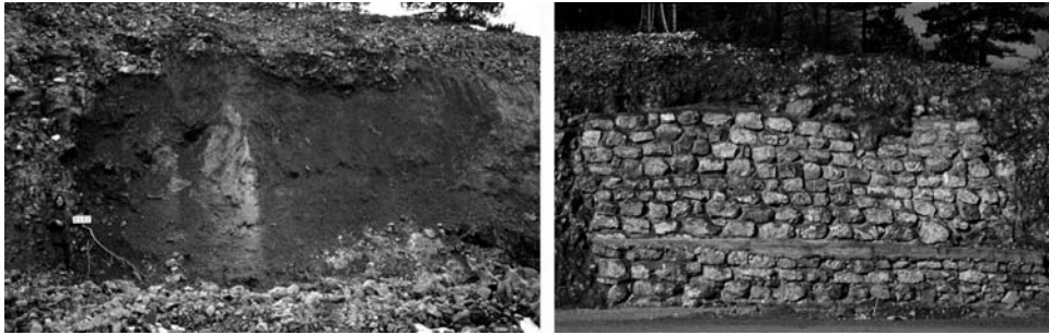
Figure 12.6. A sediment-filled cave in the wall of a road cutting in Slovenia, seen when it was first exposed and later with a masonry wall across its sediment fill.
