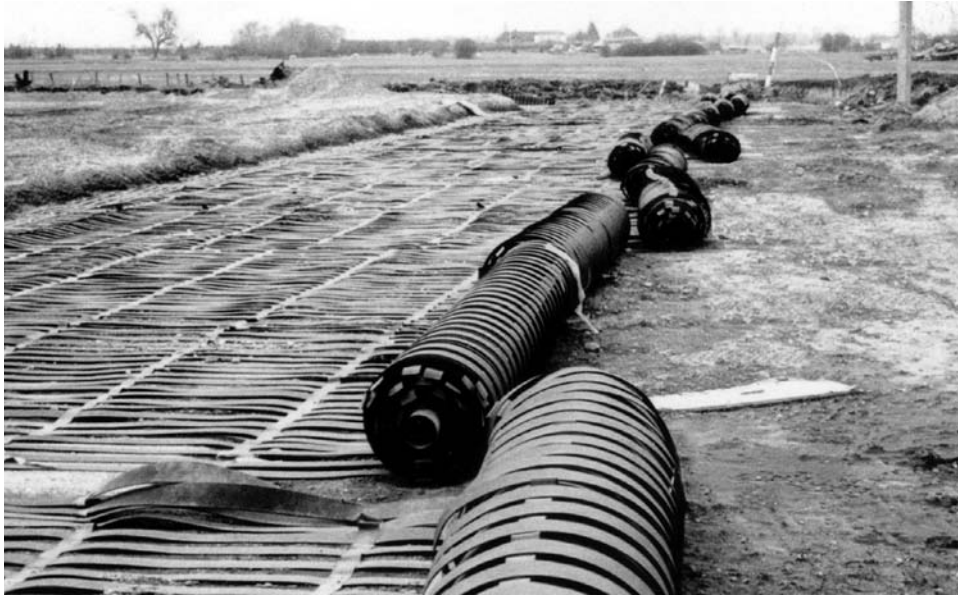
Figure 12.7. Heavy paralink geogrid being rolled out onto a road sub-base as a protection measure against sinkhole development in the underlying soil. TW.
