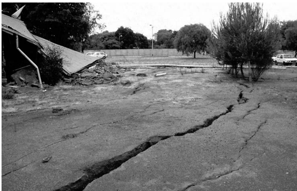
Figure 13.12.2. Ground fissures around the subsidence feature adjacent to the northern end of the Centurion warehouse after it finally collapsed in November 1994.
