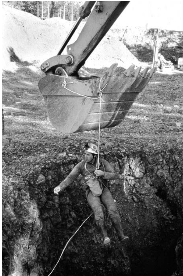
Figure 9.7. Direct exploration: an engineering geologist, who is also an experienced caver, abseils from an excavator bucket into a sinkhole that collapsed into an open cave during road construction in Slovenia.
