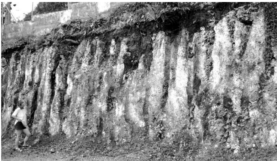
Figure 5.16. Closely spaced pipes within a soft raised limestone on Efate Island, Vanuatu; some of the soil fills have been washed out since the face was exposed on a building site. TW.
