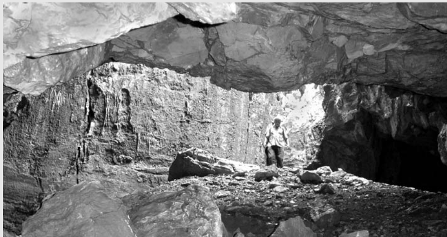
Figure 5.1.3. Looking up the debris pile, from the Chunglim mine tunnel into the open daylight shaft that is the emptied buried sinkhole; the shadowed roof of the mine is scored by narrow soil-choked fissures around the perimeter of the old filled sinkhole.
