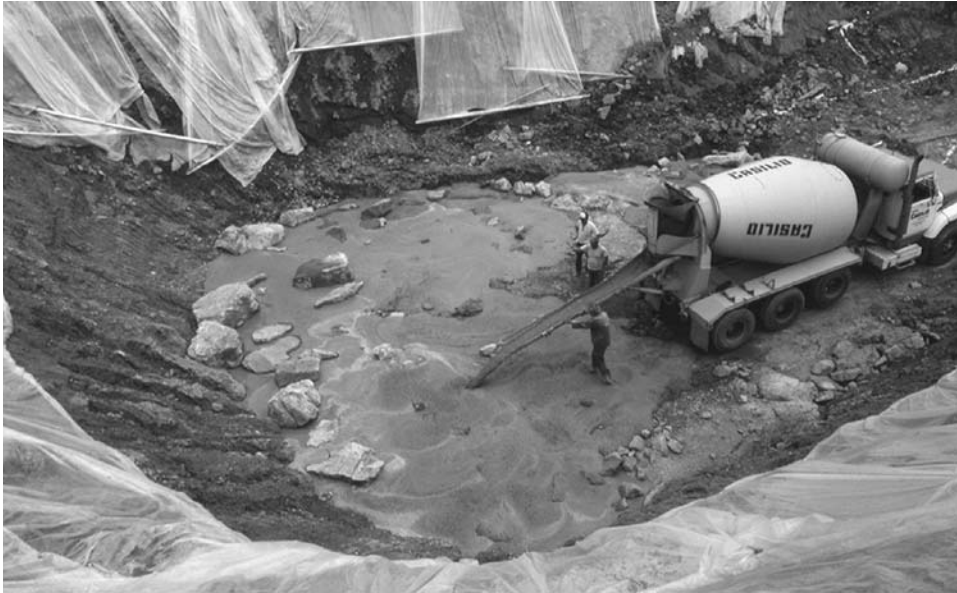
Figure 11.10. Pouring the last of the concrete into the plug of chunk rock in the Macungie sinkhole, before rebar was laid as reinforcement to a cast concrete cap.
