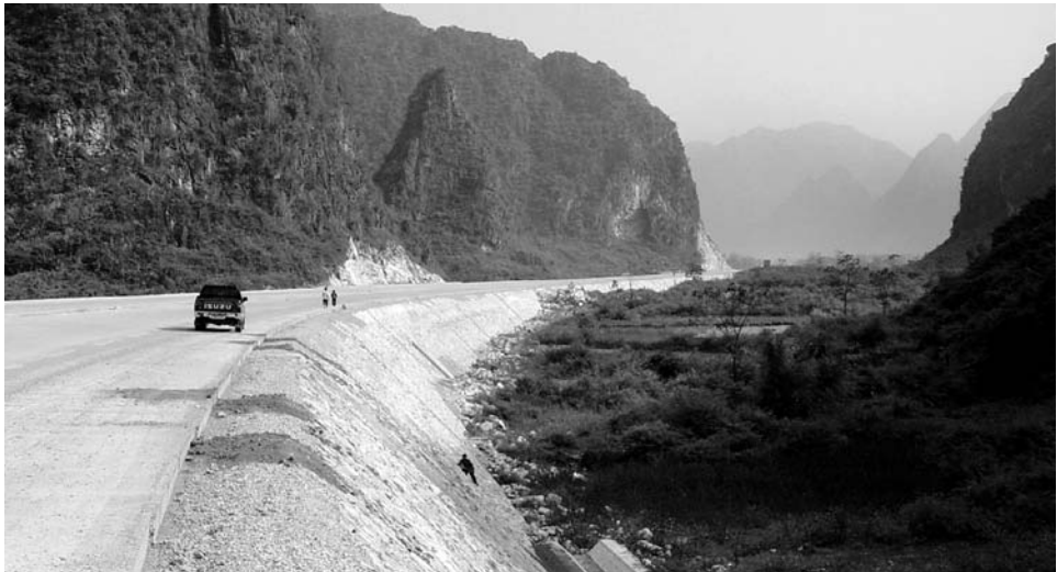
Figure 13.5.3. A rock fill embankment that required considerable ground treatment to carry the Shui-Nan Highway through the Disu karst.
