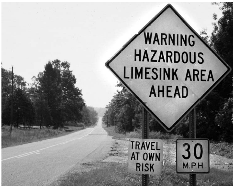
Figure 8.11. Road signs that warn of the ongoing hazard to a road across Alabama's Dry Valley, where sinkholes are induced in the soil by de-watering at a nearby limestone mine. TW.
