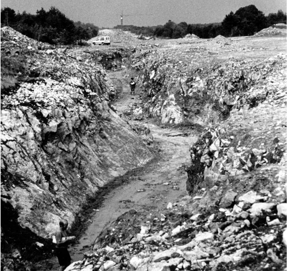
Figure 13.3.2. Large unroofed cave passage that lay parallel to the karst surface, near Divača, seen after its sediment has been removed in preparation for road construction. Photo: Martin Knez.
