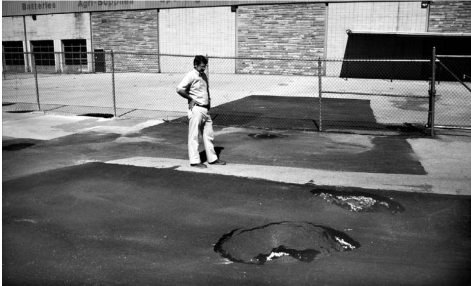
Figure 11.4. A small sinkhole that has been repeatedly filled, without proper treatment, under a much-patched parking lot in Bowling Green, Kentucky. TW.
