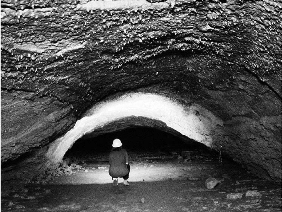
Figure 13.4.4. The stable arch roof in sound basalt where the Sung Gul lava tube lies directly beneath the main road. TW.
