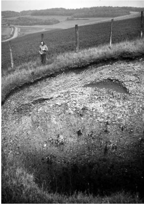
Figure 3.16. The collapse sinkhole of the Bime des Enfants in the chalk karst of northern France, 26 years after its sudden appearance. TW.
