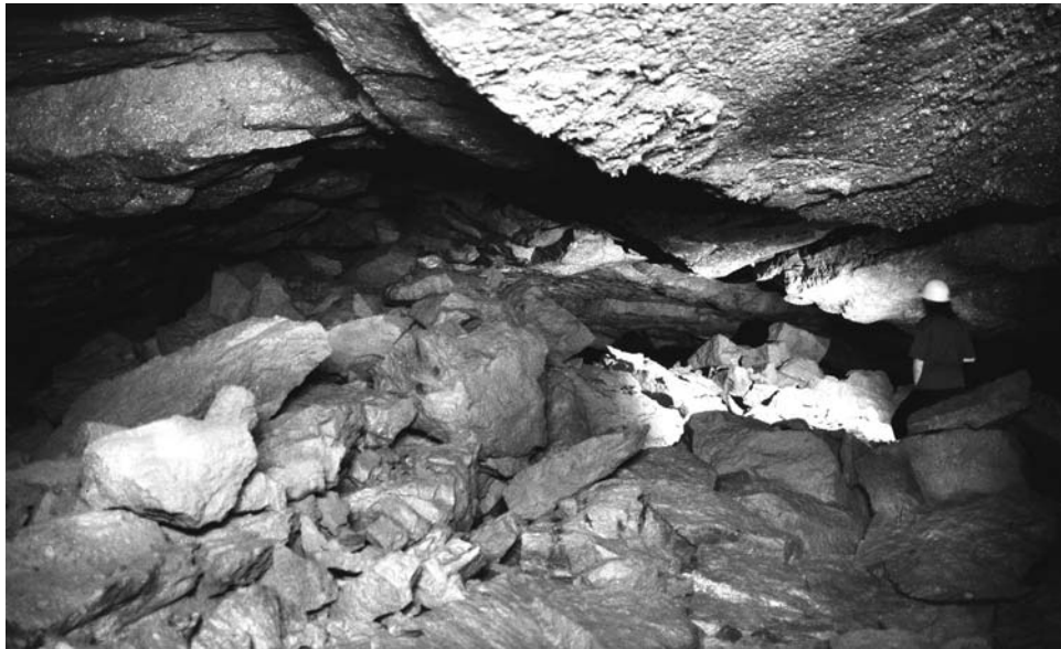
Figure 13.4.3. The collapse zone down-flow of the road, with part of the original tube roof surviving on the right. TW.
