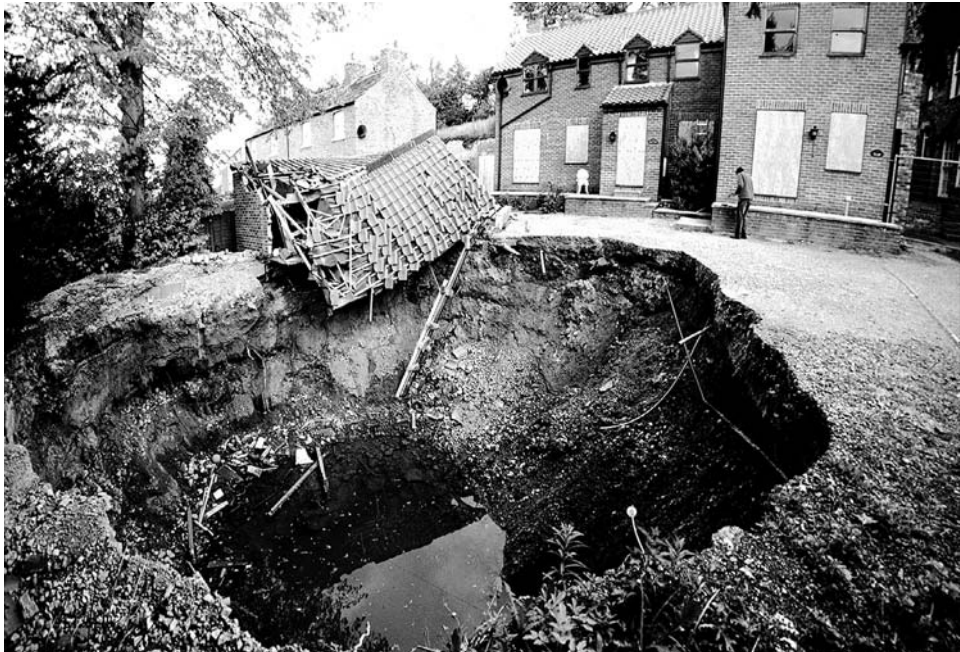
Figure 13.1.1. The open sinkhole that collapsed in front of the house on Ure Bank Terrace, Ripon. TW.
