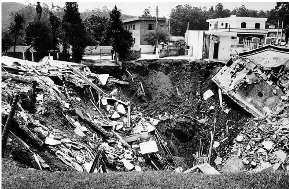
Figure 8.7. Collapse of a house in Cajamar, Brazil, in 1986 over a sinkhole induced in a thick soil cover by excessive groundwater abstraction at a nearby industrial site.
