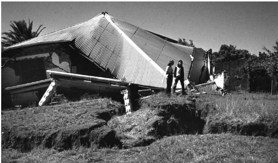
Figure 5.12. A destroyed house within a large compaction sinkhole induced by de-watering the fill in a large and deep buried sinkhole; in the abandoned Bank township in South Africa's Rand karst.
